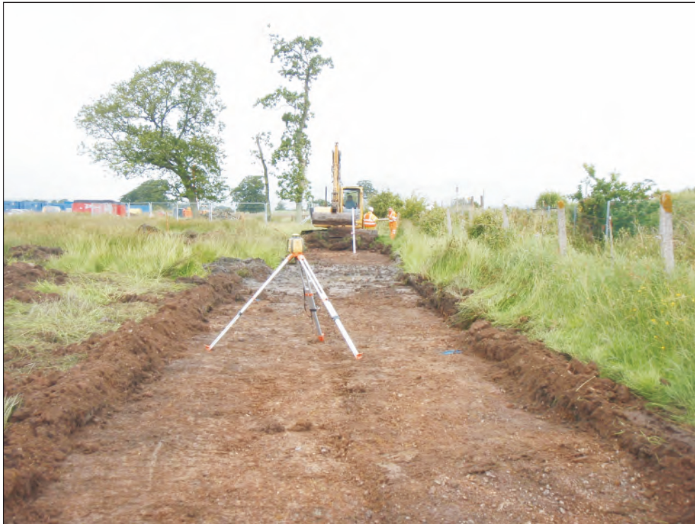
Pl. 3 General view of cycle path excavation near southern bridge abutment showing shallow topsoil (1000) overlying alluvial silts and gravels (1002). Looking northwest.
