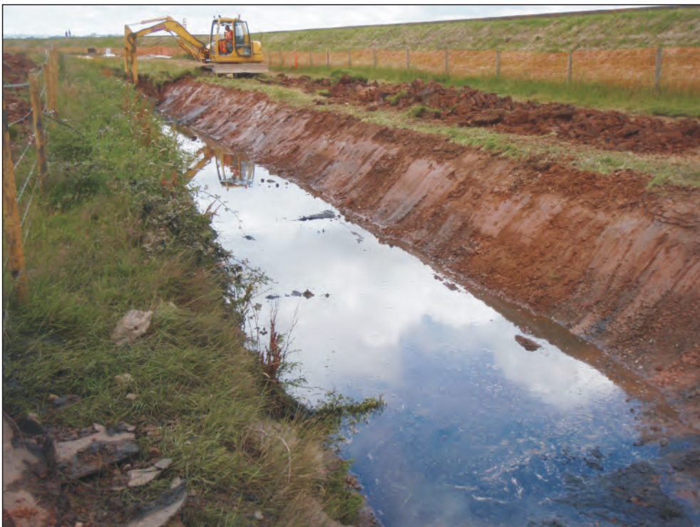
Pl. 4 General view of ditch re-profiling showing level of groundwater. Looking northwest.
