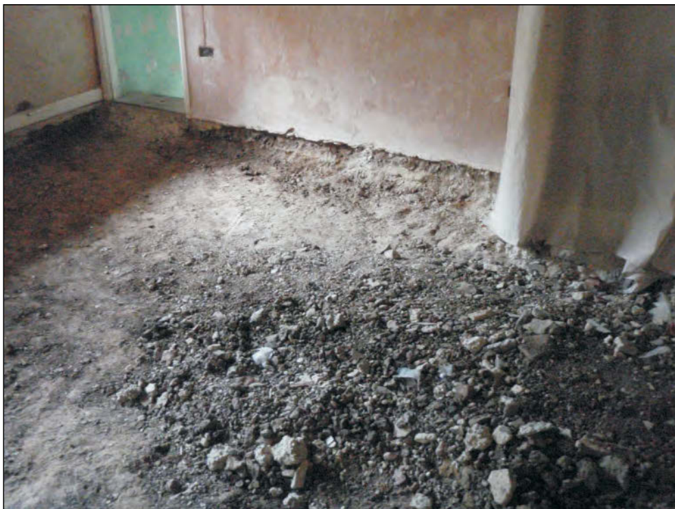
Pl. 2 Sitting Room showing exposed natural subsoil. Looking southwest.
