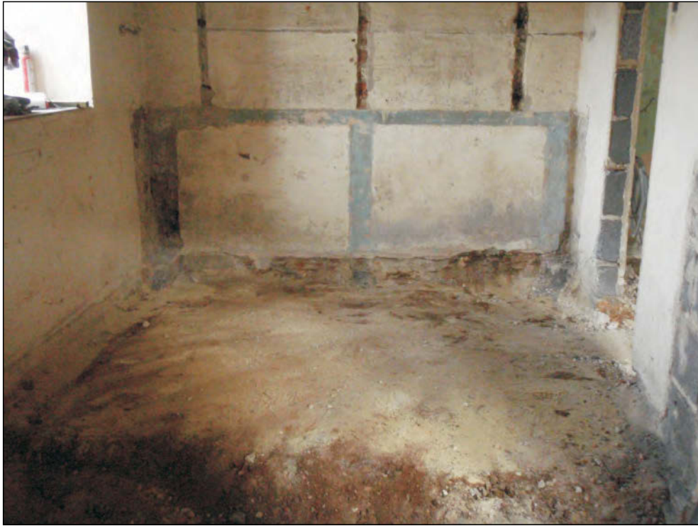
Pl. 1 Utility Room showing exposed natural subsoil. Looking north.
