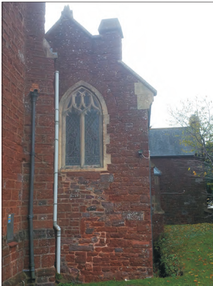
Pl. 2 South Aisle western elevation. Looking northeast.
