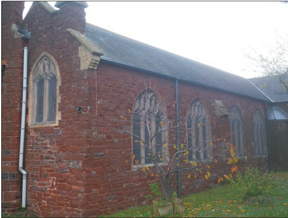
Pl. 1 South Aisle exterior view. Looking northeast.
