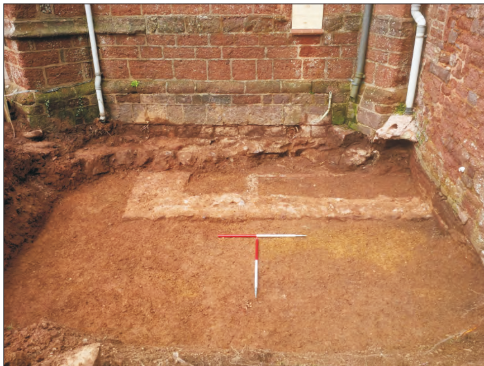
Pl. 4 Annex showing foundation of 19th century boiler house, foundations of tower and burial horizon. 1m and 1m scales. Looking northwest.
