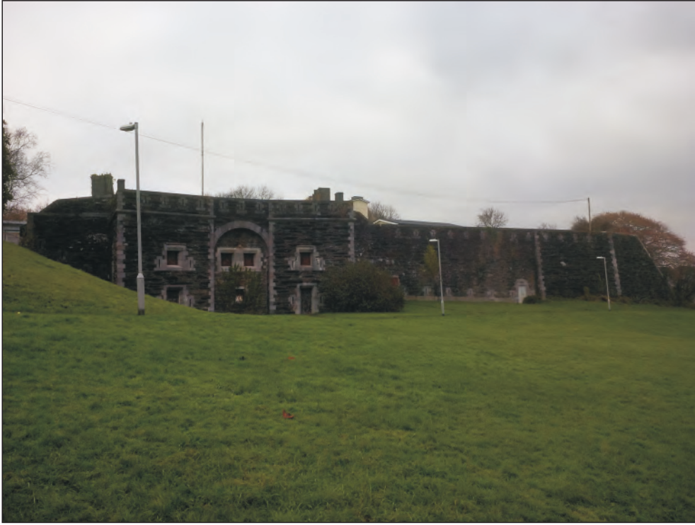
Pl. 1 General view of Knowle Battery. Looking northeast.
