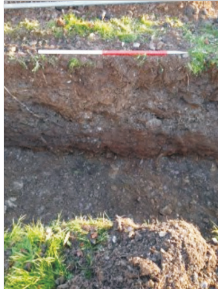
Pl. 12 Close-up section trench 3 showing modern made ground (303) above buried soil (304) and upcast (305). 1m scale. Looking northwest.
