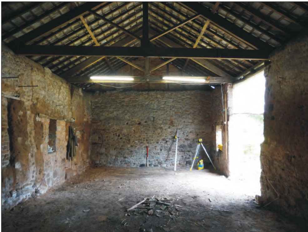
Pl. 18 General view of inside of barn showing west end.
