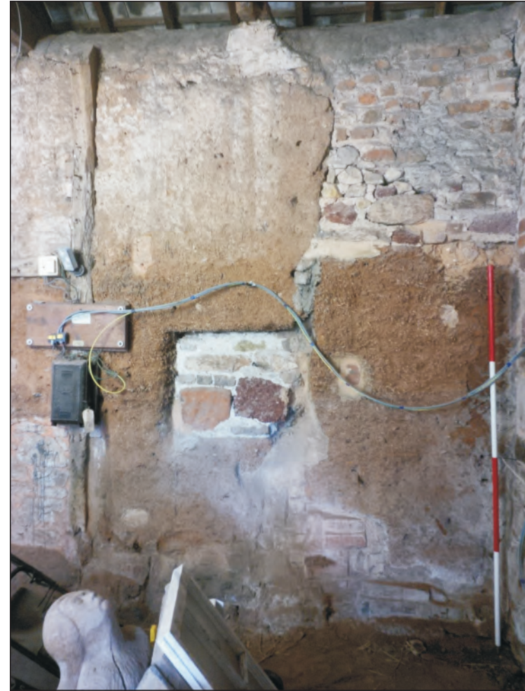
Pl. 14 Detail of south elevation showing blocked opening.
