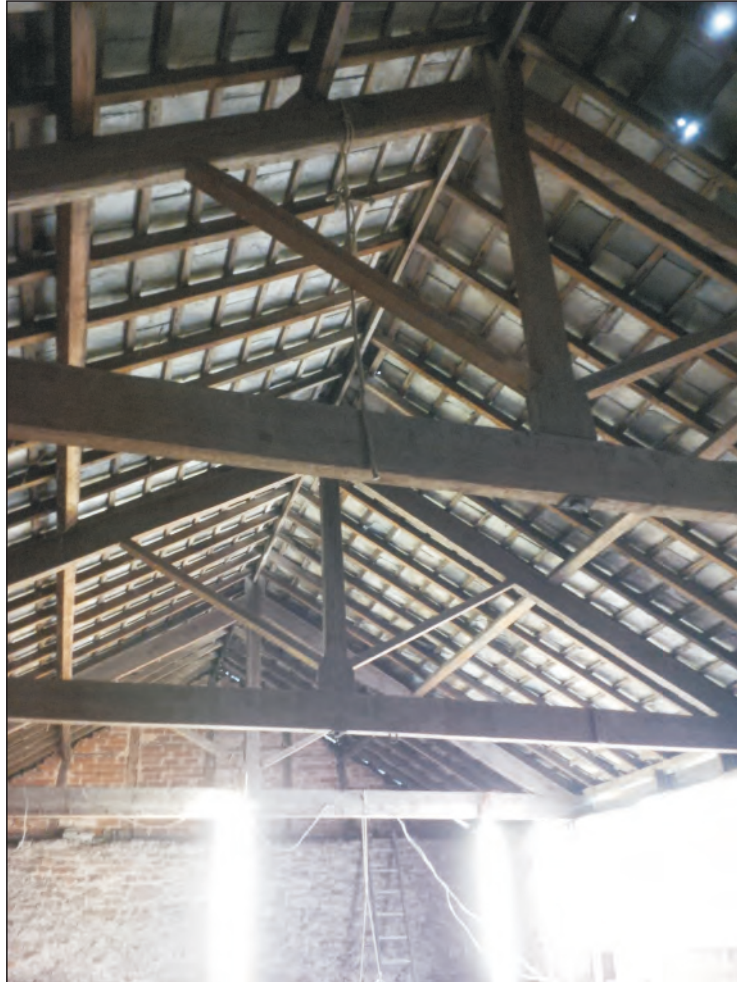
Pl. 21 Detail of 19th century roof arrangement.
