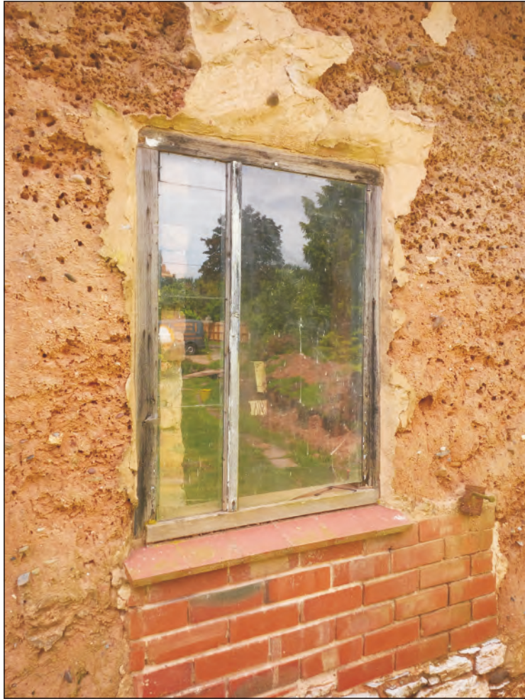
Pl. 5 Detail of north elevation showing modern window.
