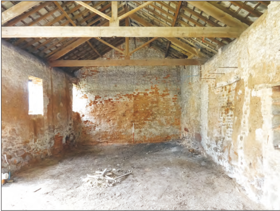
Pl. 17 General view of inside of barn showing east end.
