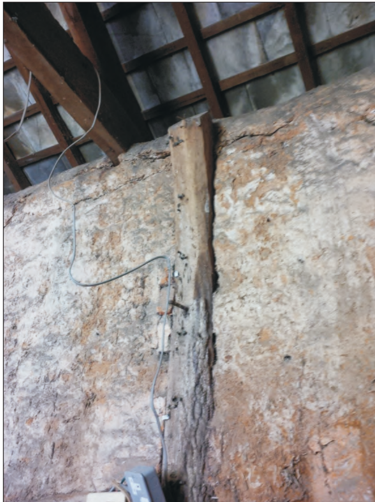
Pl. 12 Detail of in-situ sawn-off cruck in south elevation.
