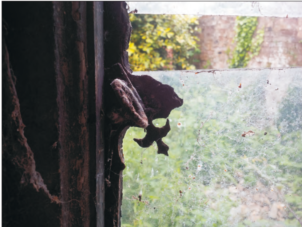
Pl. 8 Detail of original turnbuckle with fleur-de-lys terminal.
