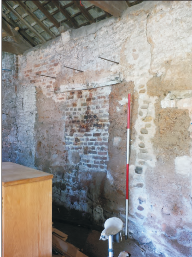
Pl. 15 Detail of south elevation showing infilled cruck chase.
