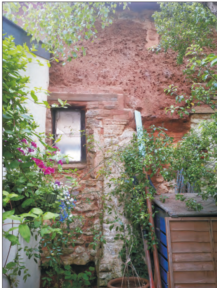
Pl. 10 Detail of south elevation showing blocked doorway.
