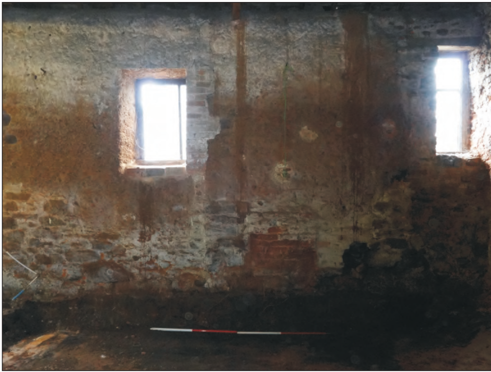
Pl. 11 Detail of north elevation showing infilled cruck chase to the right of the window.
