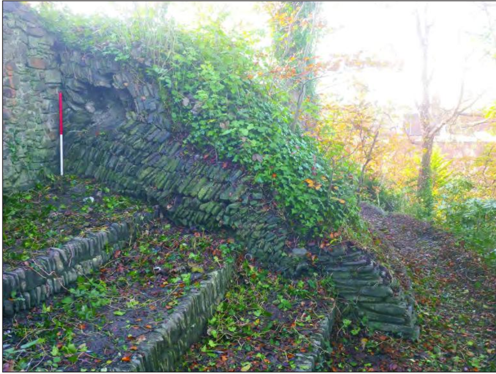
Pl. 5 General view of wall prior to re-building. 2m scale. Looking south.
