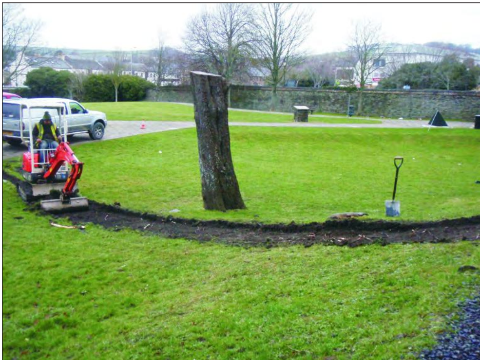
Pl. 10 General view of northern path. Looking northwest.
