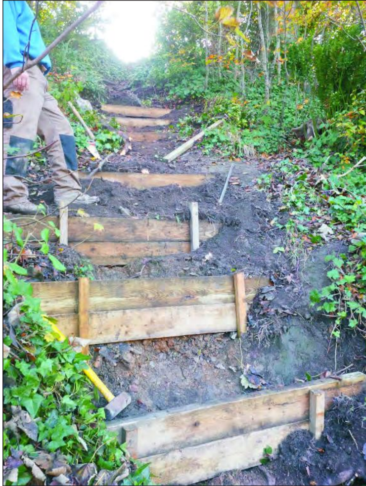
Pl. 3 General view of re-instatement works. Looking south.
