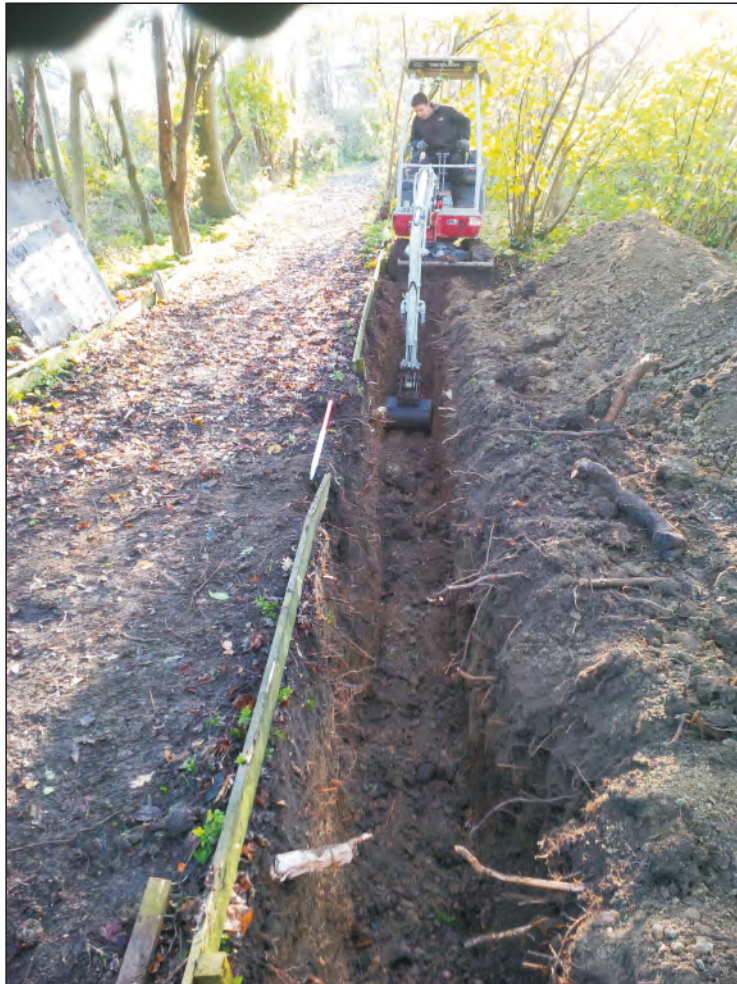
Pl. 1 General view of badger fence trench under excavation. Looking south.
