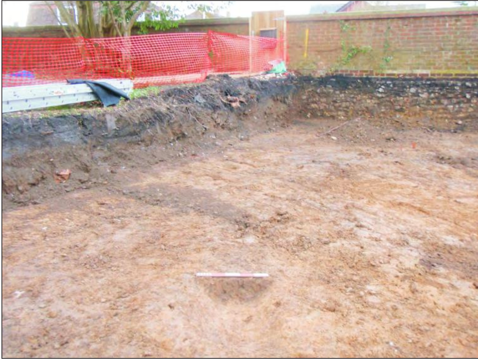
Pl. 3 General view of tree throw [108], 0.5m scale. Looking southwest.
