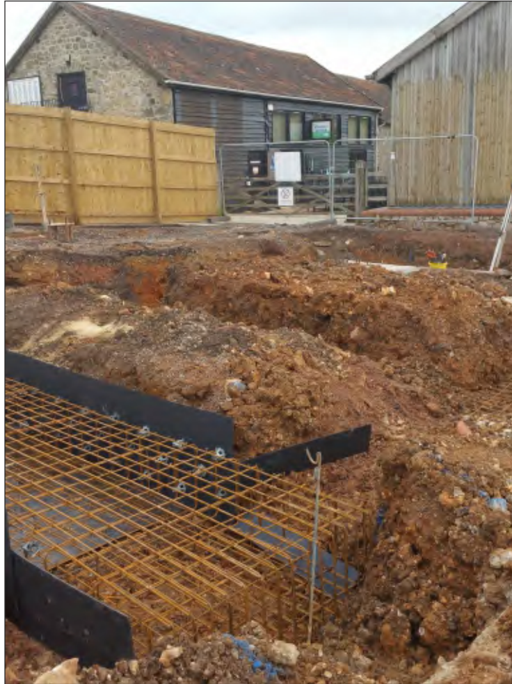
Pl. 1 General view of new restaurant area showing depth of foundations through modern made ground. Looking northeast.
