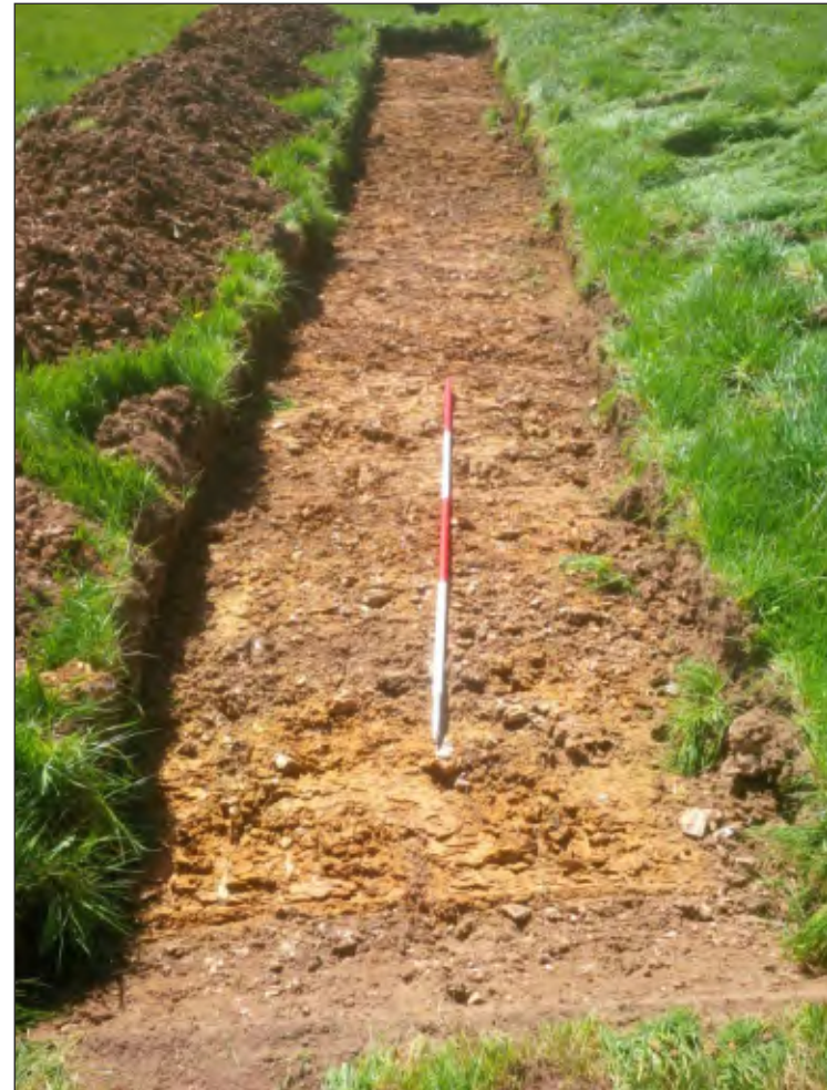
Pl. 19 General view of trench 15. 2m scale. Looking southwest.
