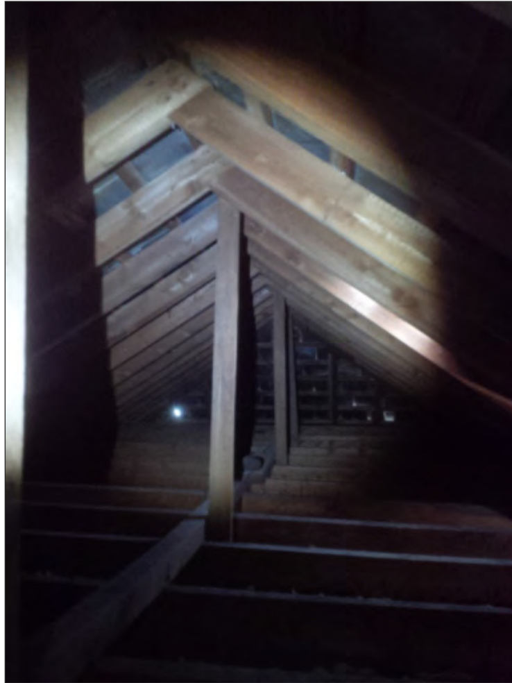
Pl. 13 General view of roof arrangement. Looking south.
