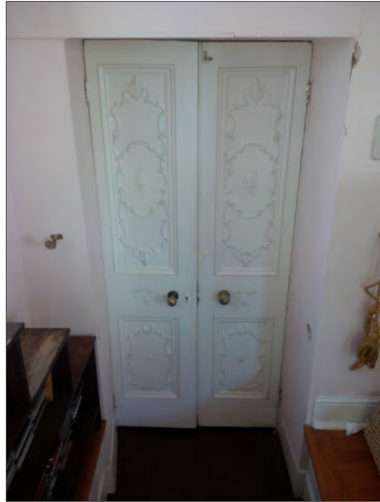
Pl. 8 Close-up of decorated internal door panels. Looking south.
