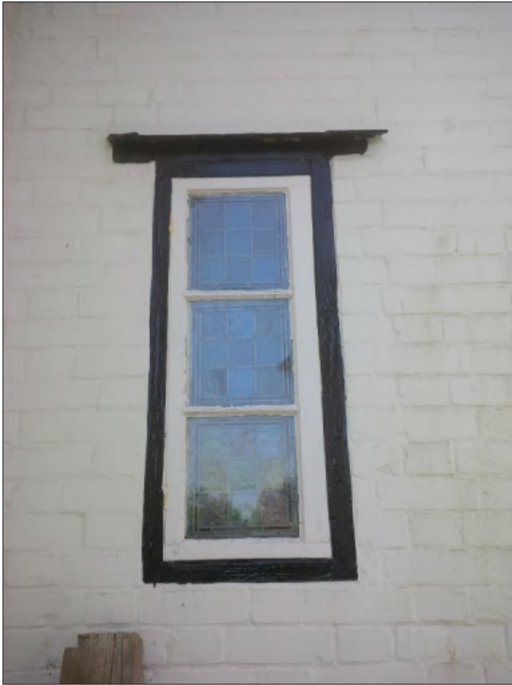
Pl. 7 Close-up of small window in east elevation. Looking west.
