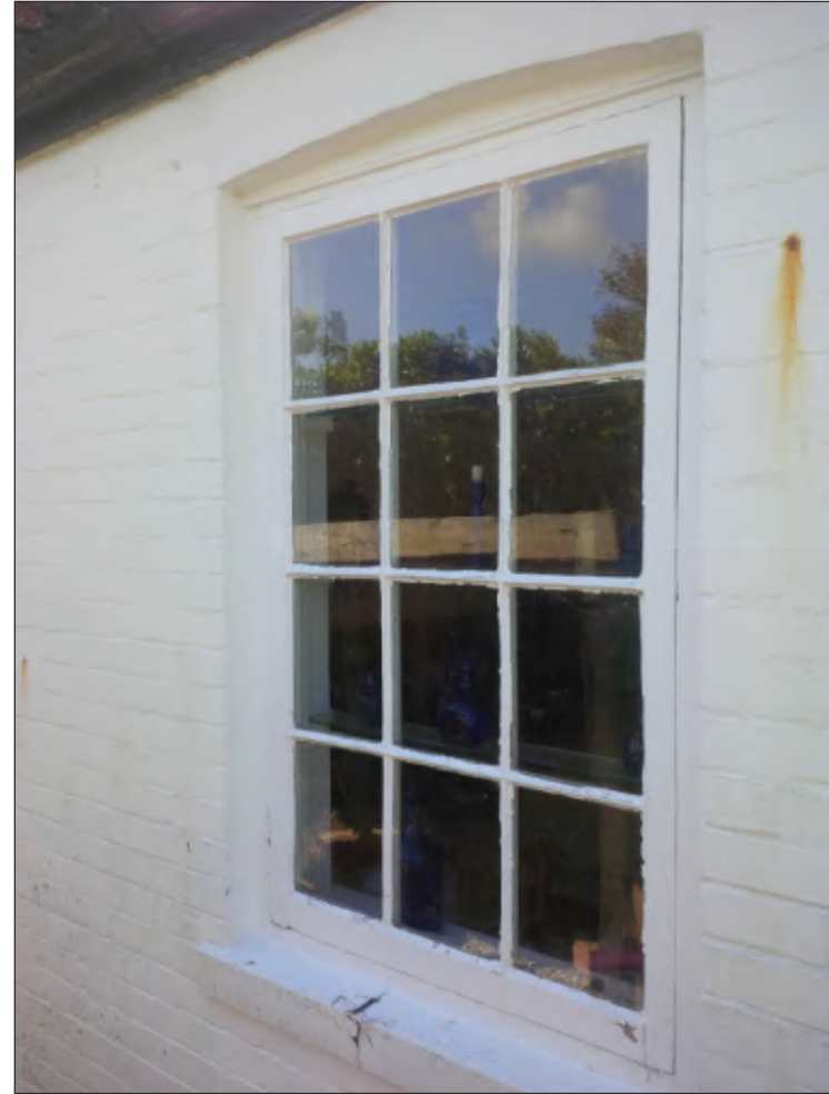
Pl. 4 General view of window in north elevation. Looking southeast.
