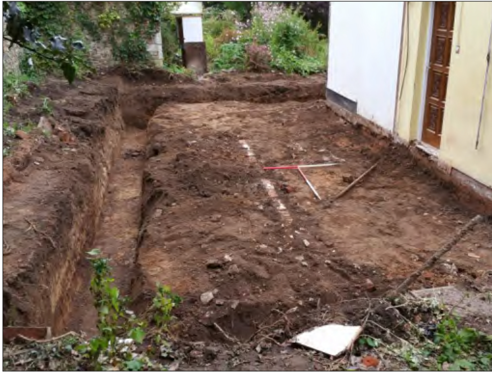
Pl. 1 General view of excavations. 1m scales. Looking south.
