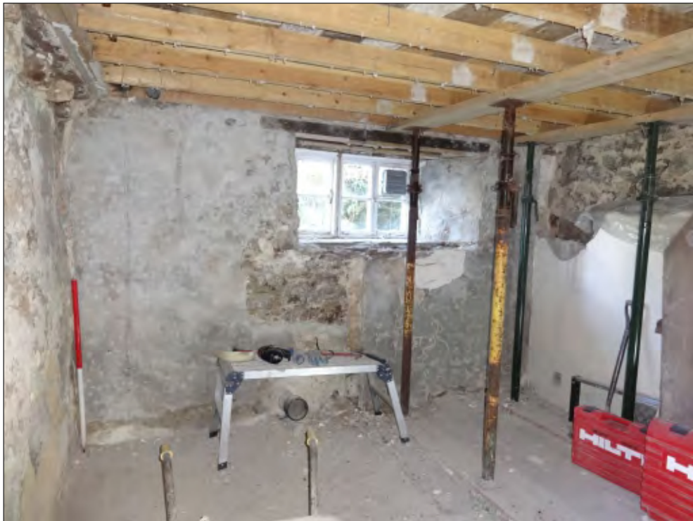
Pl. 2 The inner room after stripping, showing the absence of any sockets for an earlier floor level. 1m scale. Looking west.
