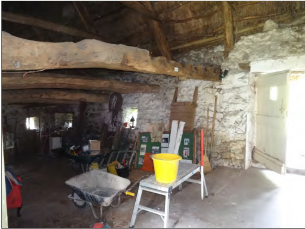
Pl. 11 View of the cross passage showing sockets for the beams supporting a sleeping platform over its western part. 1m scale. Looking southwest.
