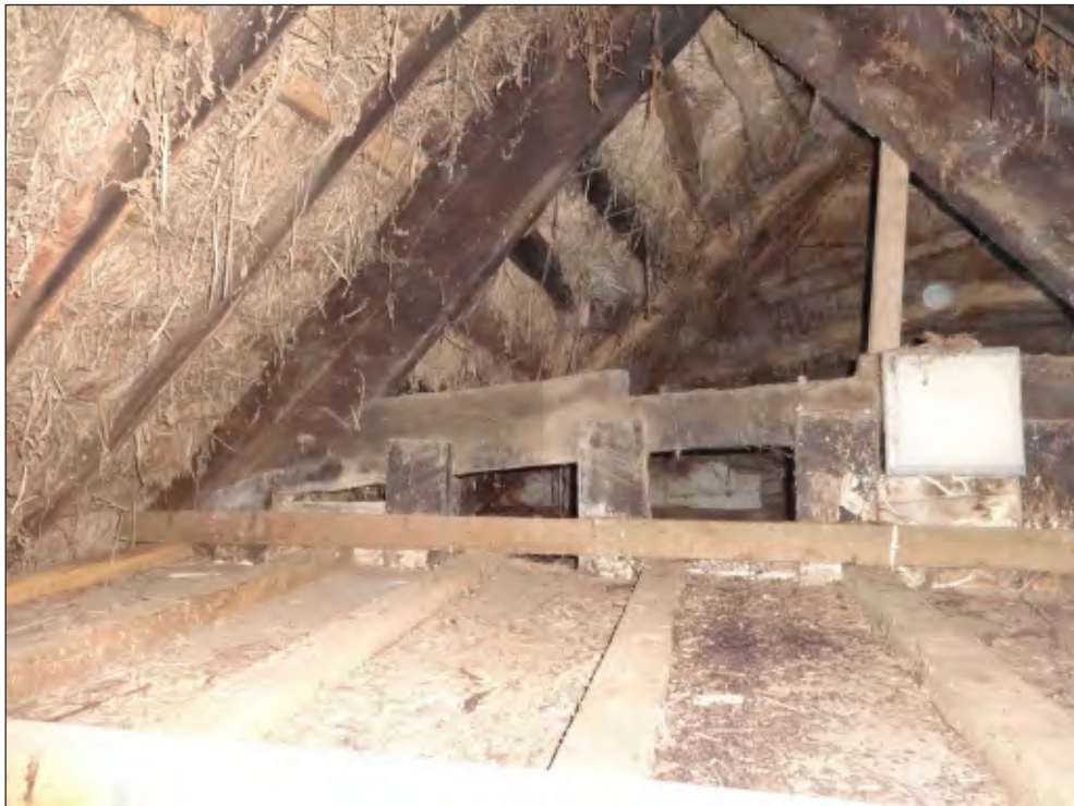
Pl. 18 View of the roof space above the hall chamber, looking north, showing smoke blackening on the inner face of the partition.
