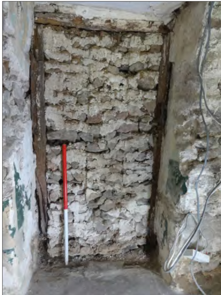
Pl. 6 Detail of the blocked main doorway to the hall, showing the imprint of a 16th- or 17th-century door with applied vertical fillets. 1m scale. Looking east.
