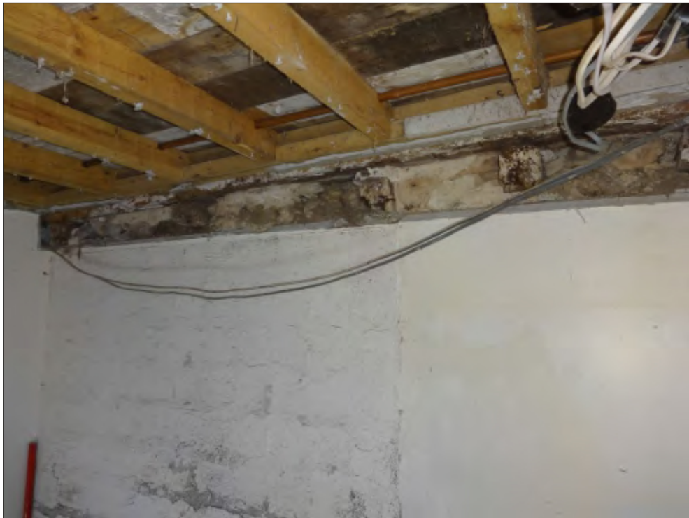
Pl. 4 Detail of the construction of the jetty showing the longer ends of alternate joists beneath the jetty towards the inner room. Looking southeast.
