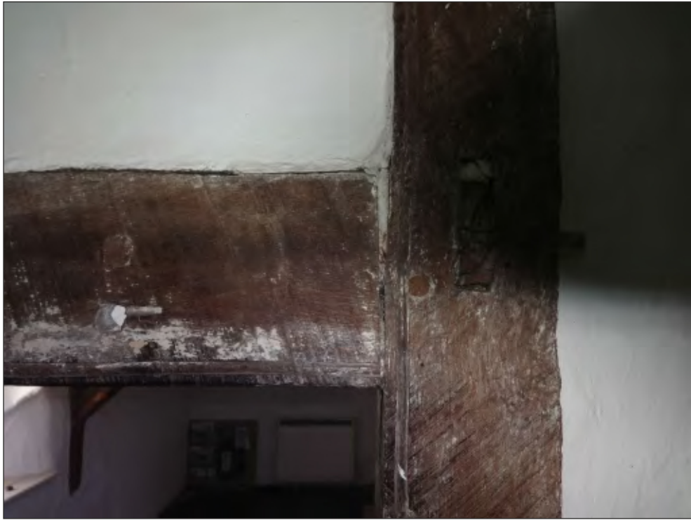
Pl. 19 Detail of the doorway to the hall chamber, seen from the north, showing the scratch mouldings and the tenon of the head beam of the spere.
