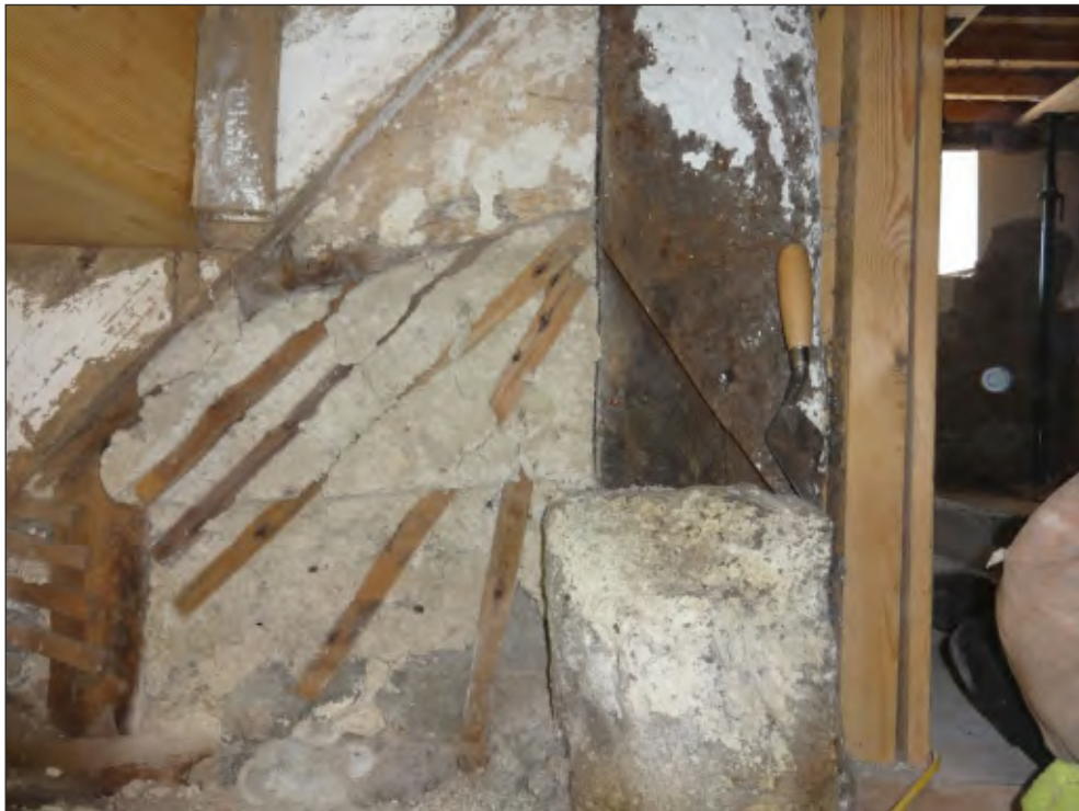
Pl.16 Detail of the area beneath the staircase, showing the diagonal socket and the stone plinth and post. the trowel is added for scale. Looking west.
