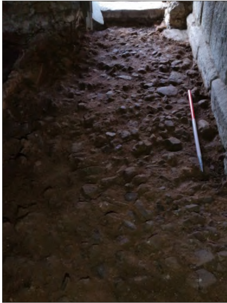
Pl. 13 General view of rough cobbled surface in cross-passage. 1m scale. Looking west.
