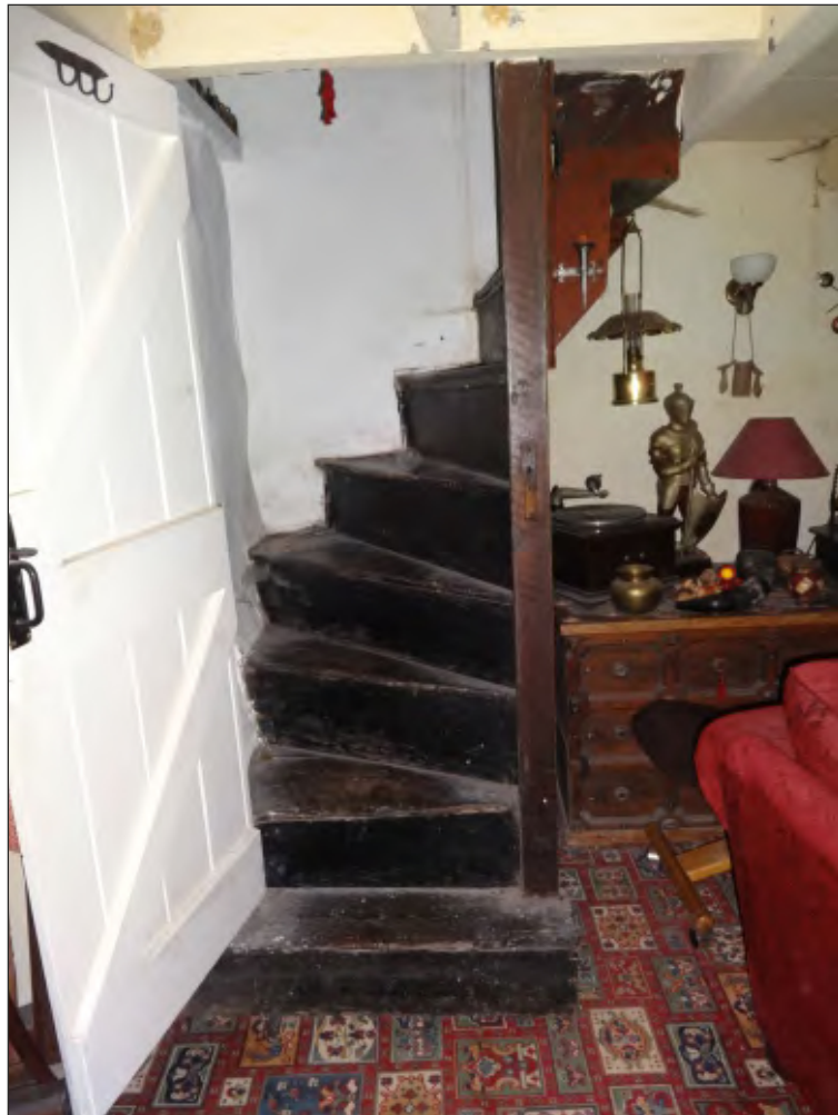
Pl. 20 View of the 19th-century staircase in the parlour wing, showing a timber newel within a confined space. S similar structure may have risen within the inner room. Looking north.
