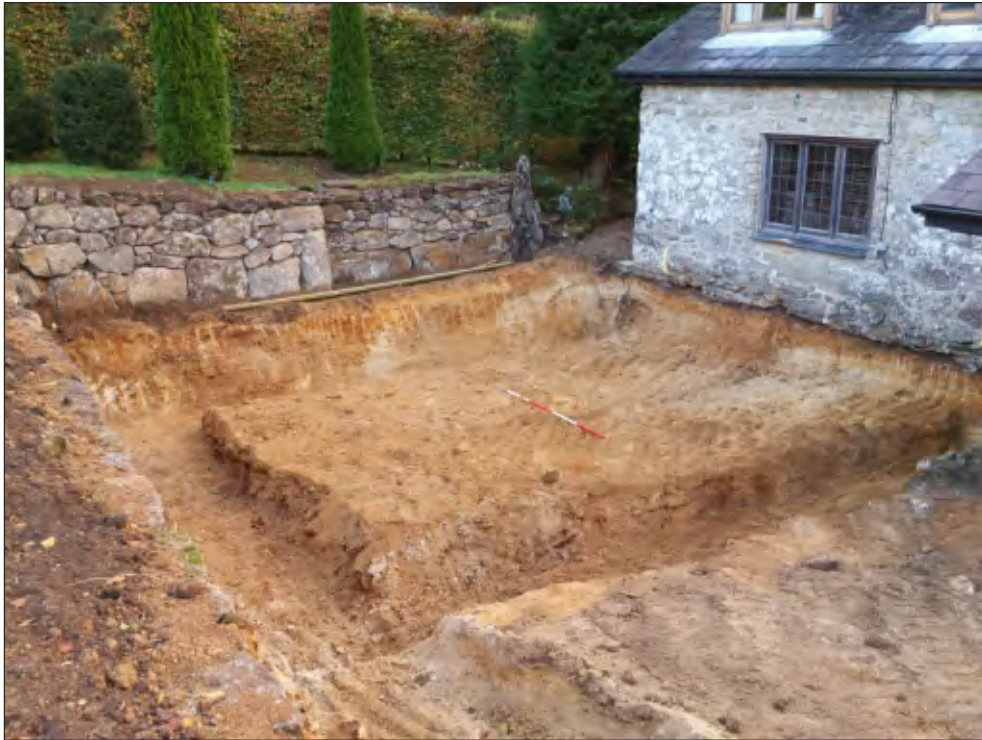
Pl. 1 General view of extension area. 2m scale. Looking northeast.
