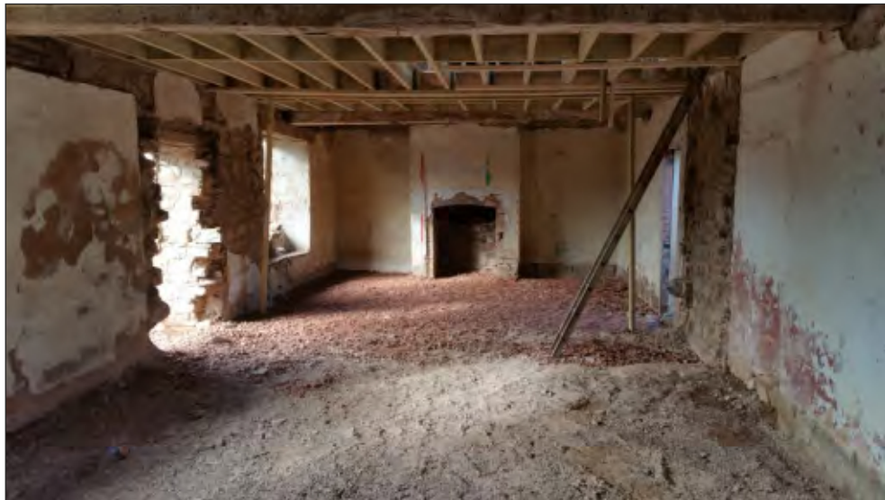
Pl. 3 General view towards room G02 after removal of solid cross walls. 2m scale. Looking west.
