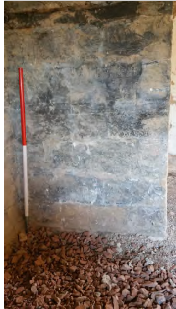
Pl. 6 Detail of painted plaster decoration on jamb. 1m scale. Looking south.
