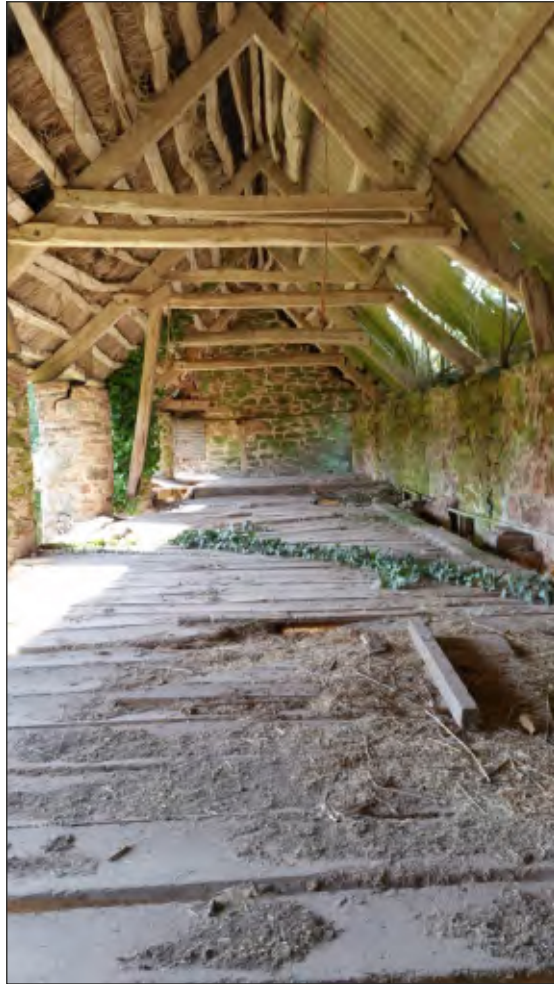
Pl. 17 General view of first floor showing roof construction. Looking west.
