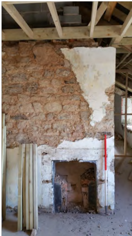
Pl. 8 Close-up of later fireplace room F02. 1m scale. Looking east.
