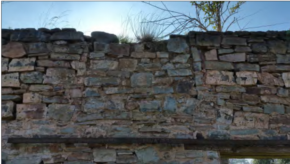
Pl. 22 Close-up showing blocked doorway to hayloft. Looking south.
