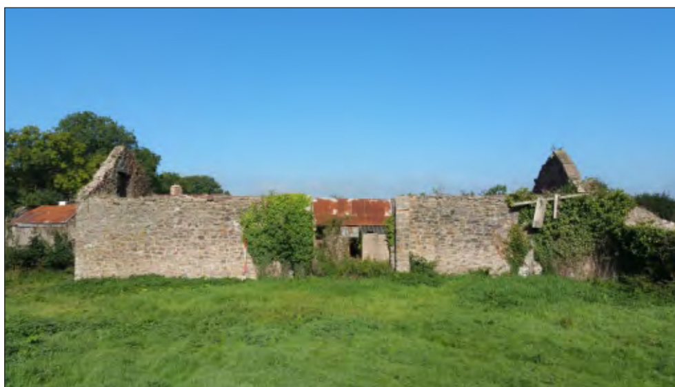
Pl. 20 General view of threshing barn. 2m scale. Looking north.
