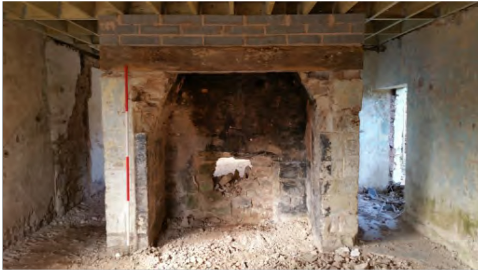
Pl. 7 Close-up of fireplace in room G04. 2m scale. Looking west.
