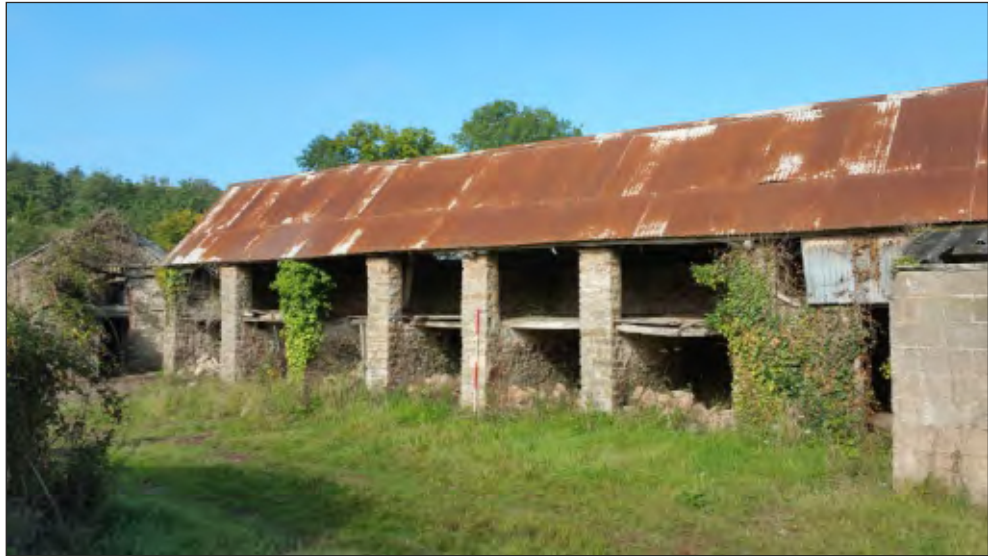
Pl. 15 General view of Linhay. 2m scale. Looking northwest.
