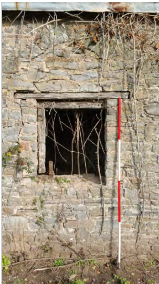
Pl. 12 Close-up of south window showing arch and C18th blocking. 2m scale. Looking north.
