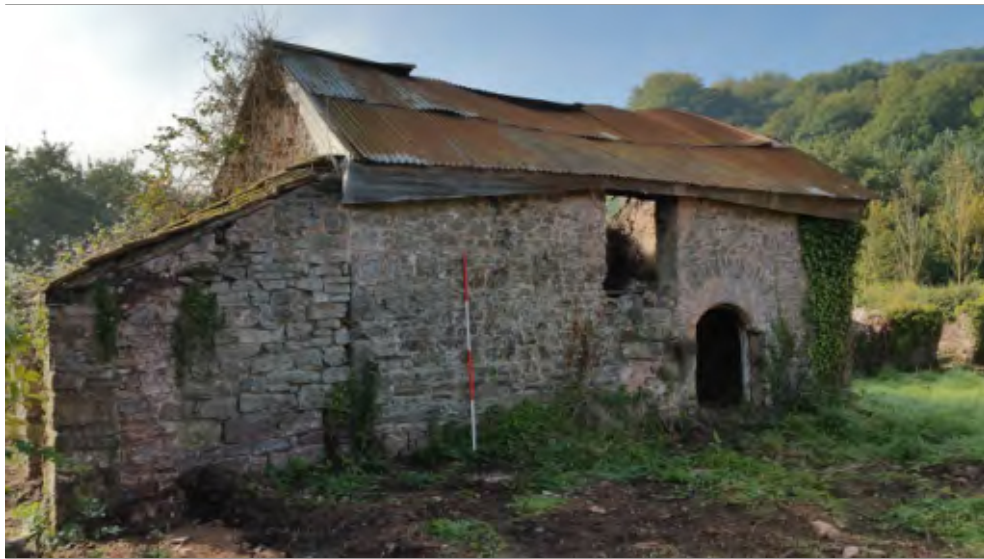
Pl. 9 General view of chapel with C19th extension (left). 2m scale. Looking southwest.
