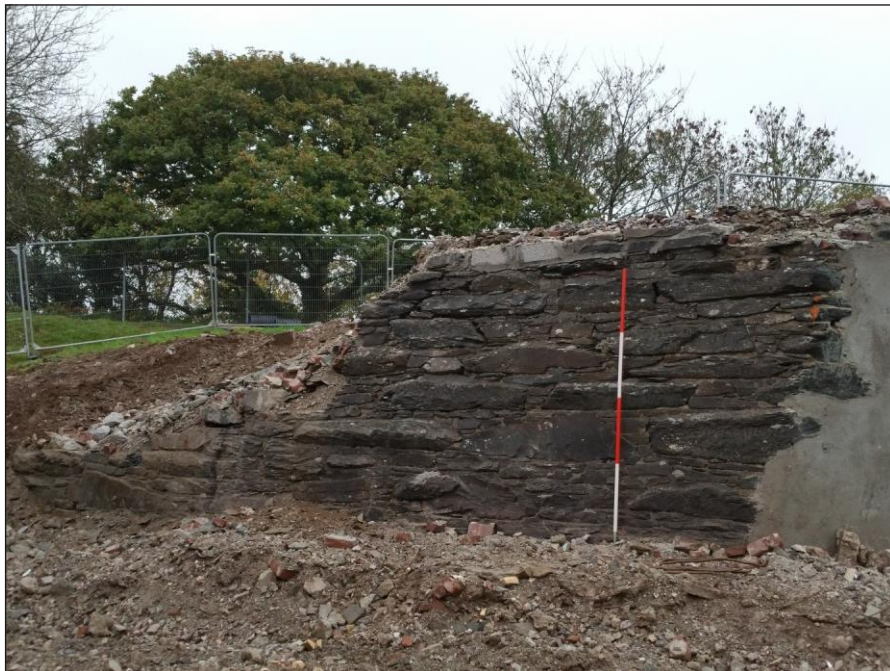
Fig. 4 Exposed section of western battery wall, looking northeast (2m).
