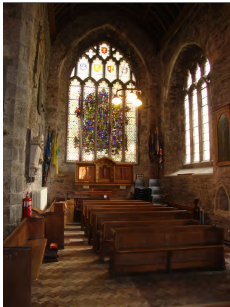
Fig. 12 General view of north transept. Looking north.
