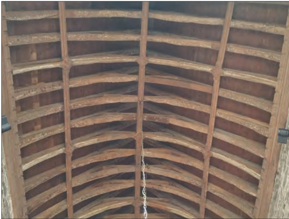
Fig. 16 General view of nave ceiling. Looking east.
