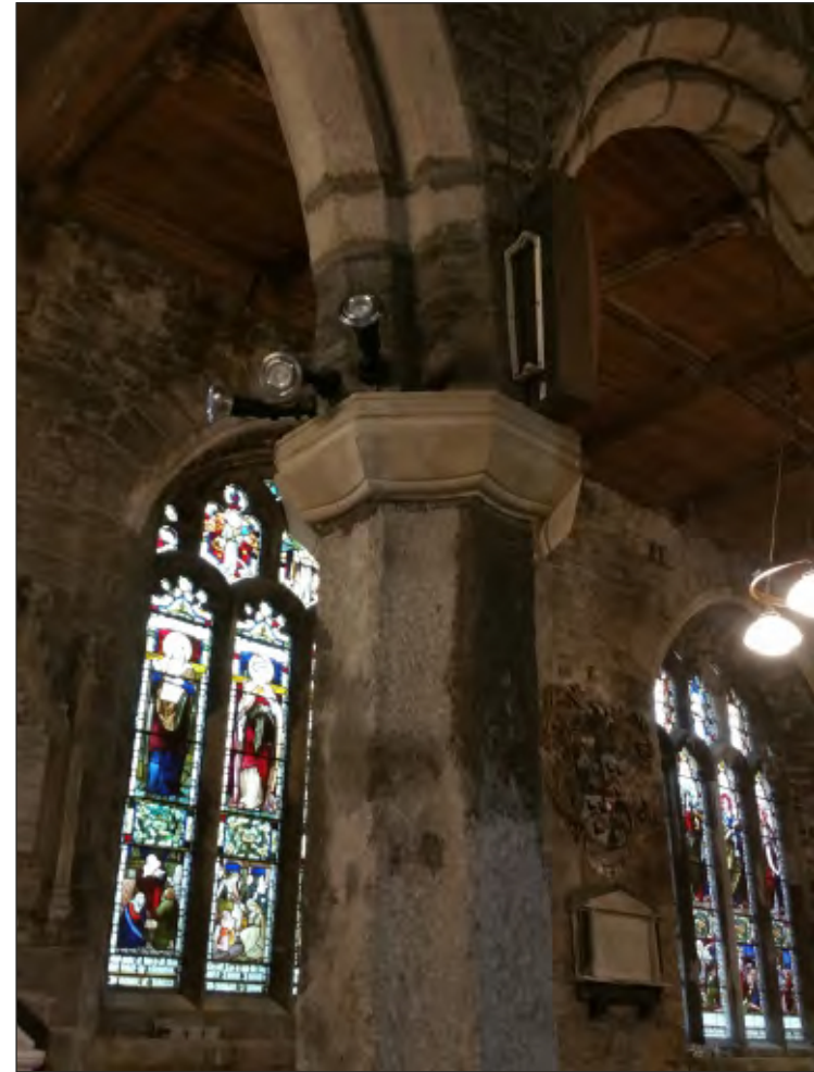
Fig. 11 Close-up of south crossing pier showing volcanic material at base of arch rather than granite highlighting the possible position of early 15th century rood screen. Looking southwest.
