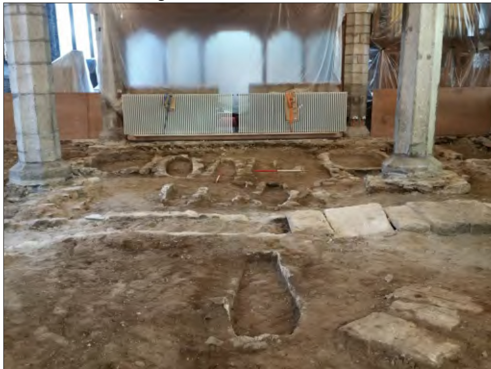
Fig. 31 General view of nave showing stone lined burials and Victorian heating duct (foreground). 1m scale. Looking east.
