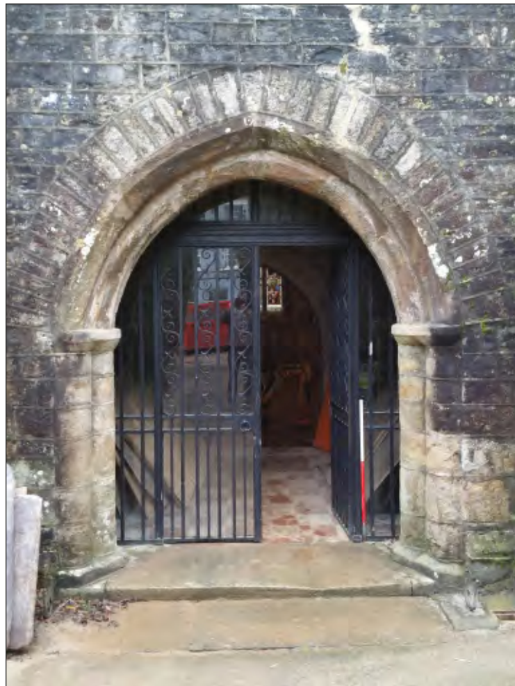
Fig. 2 Close-up of north porch with possible re-used mid-14th century arch. 2m scale. Looking south.
