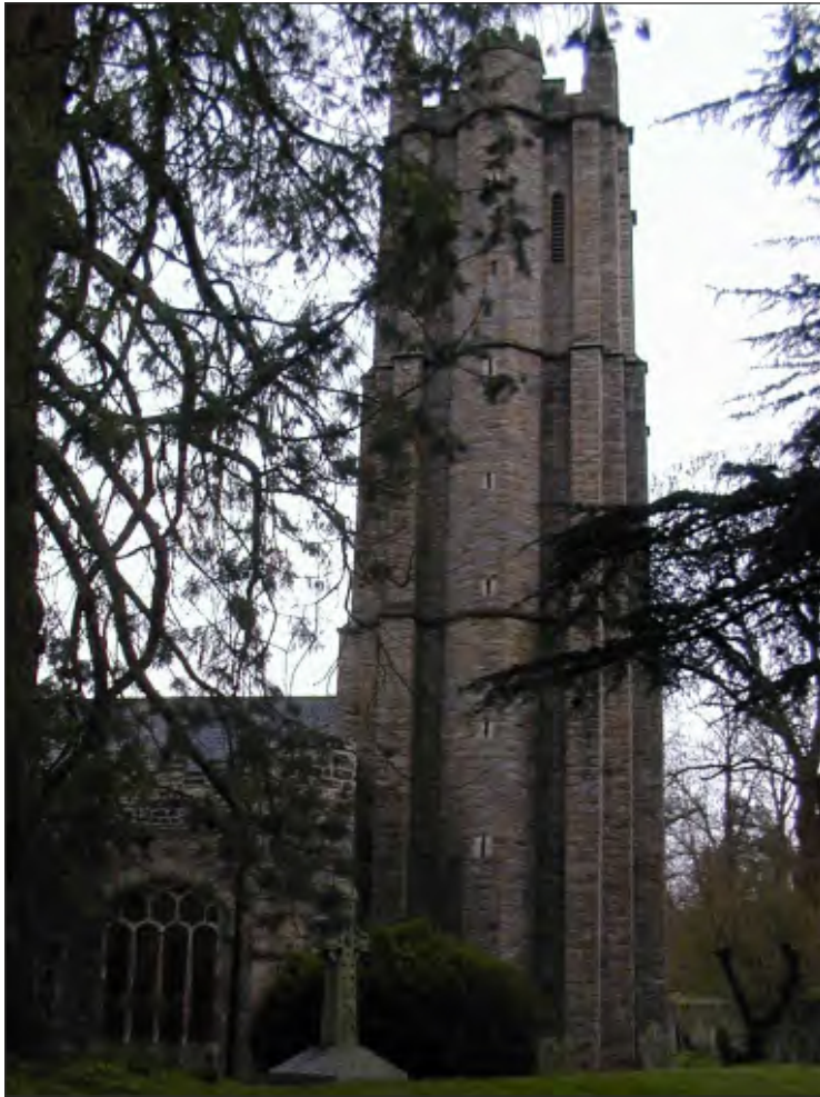
Fig. 8 General view of bell tower. Looking south.
