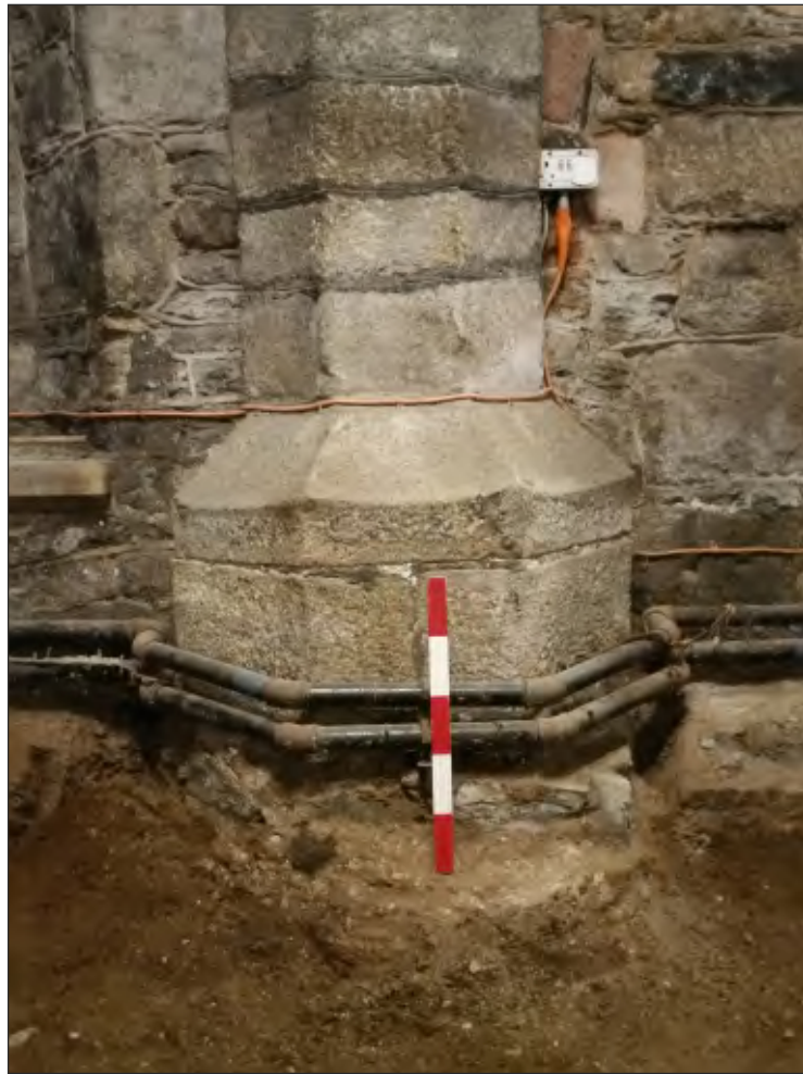
Fig. 28 Close-up showing early 15th century pier base truncating probable 13th century foundations. 0.5m scale. Looking west.
