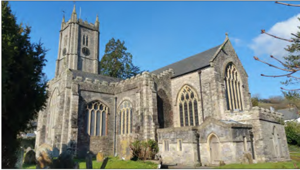
Fig. 2 General view of St Andrew's. Looking northwest.
