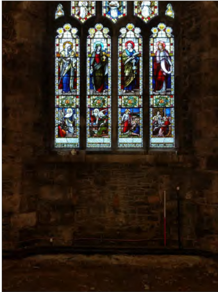
Fig. 4 Close-up showing blocked south doorway and later enlarged window. 1m scale. Looking south.
