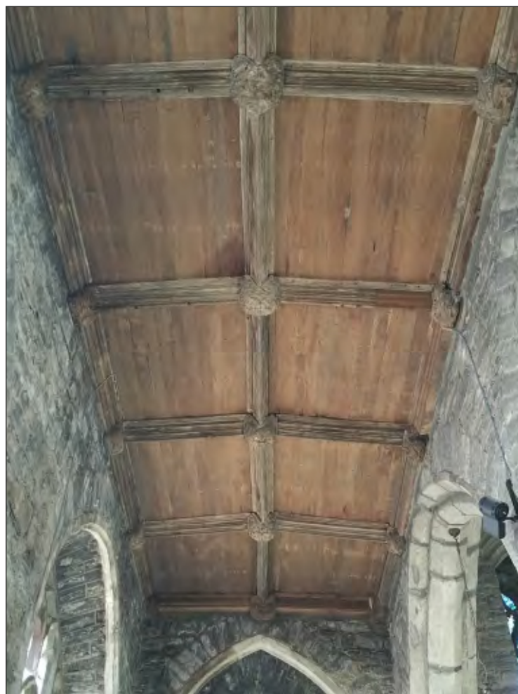
Fig. 19 General view of south aisle ceiling. Looking west.
