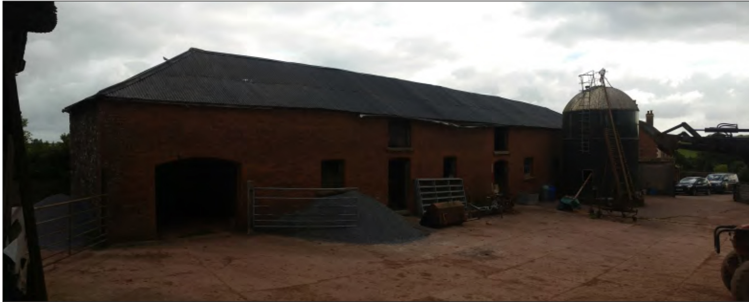
Fig. 11 General view of barn. 2m scale. Looking northeast.
