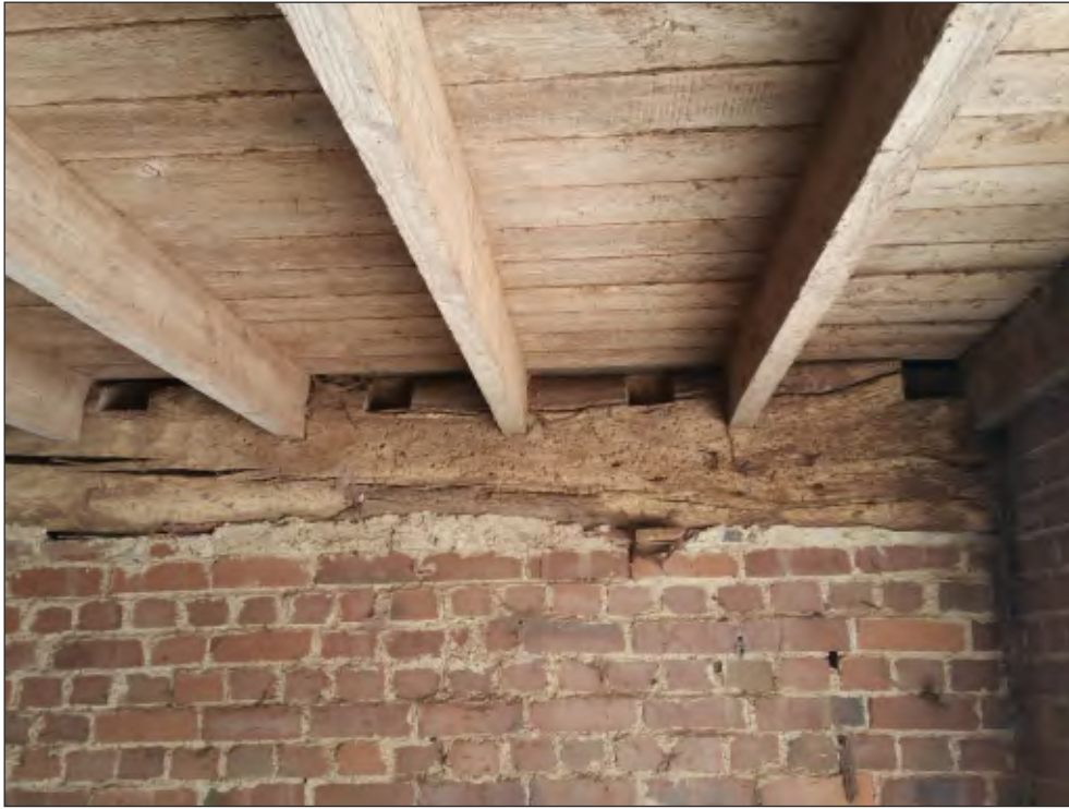
Fig. 21 Close-up showing earlier floor truss and later floor. Looking east.
