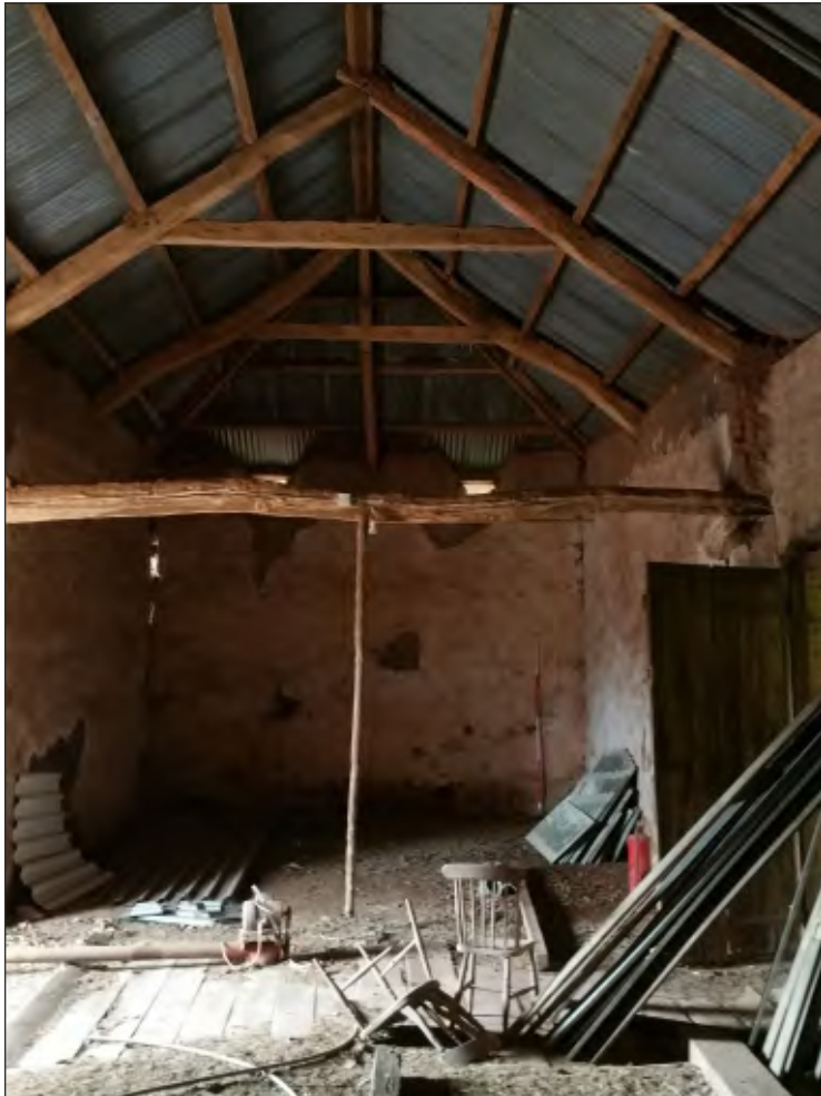
Fig. 37 General view of upper threshing barn interior showing roof construction and owl holes. 2m scales. Looking south.
