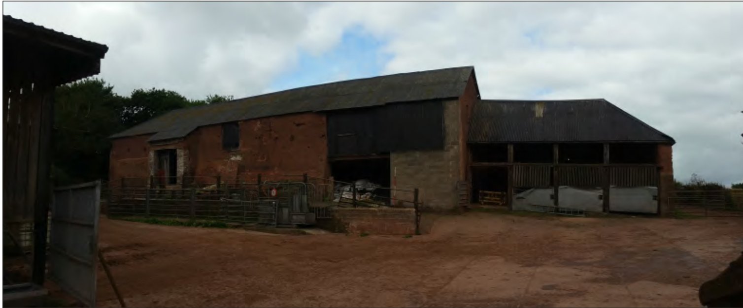
Fig. 28 General view of threshing barn and linhay. 2m scale. Looking southwest.
