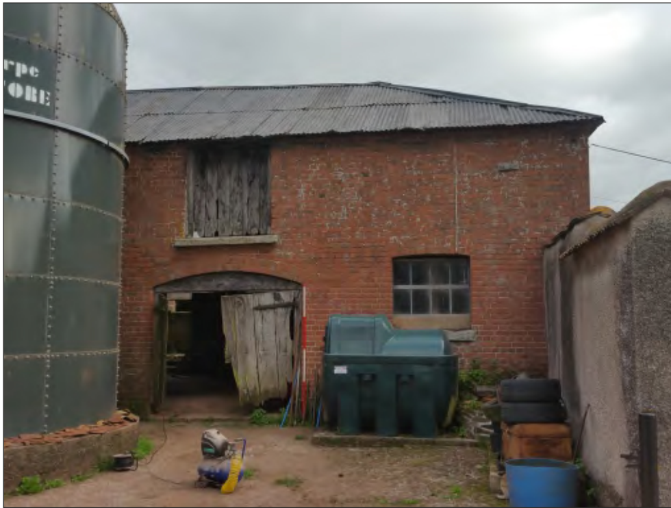
Fig. 12 General view of eastern end of barn. 2m scale. Looking north.
