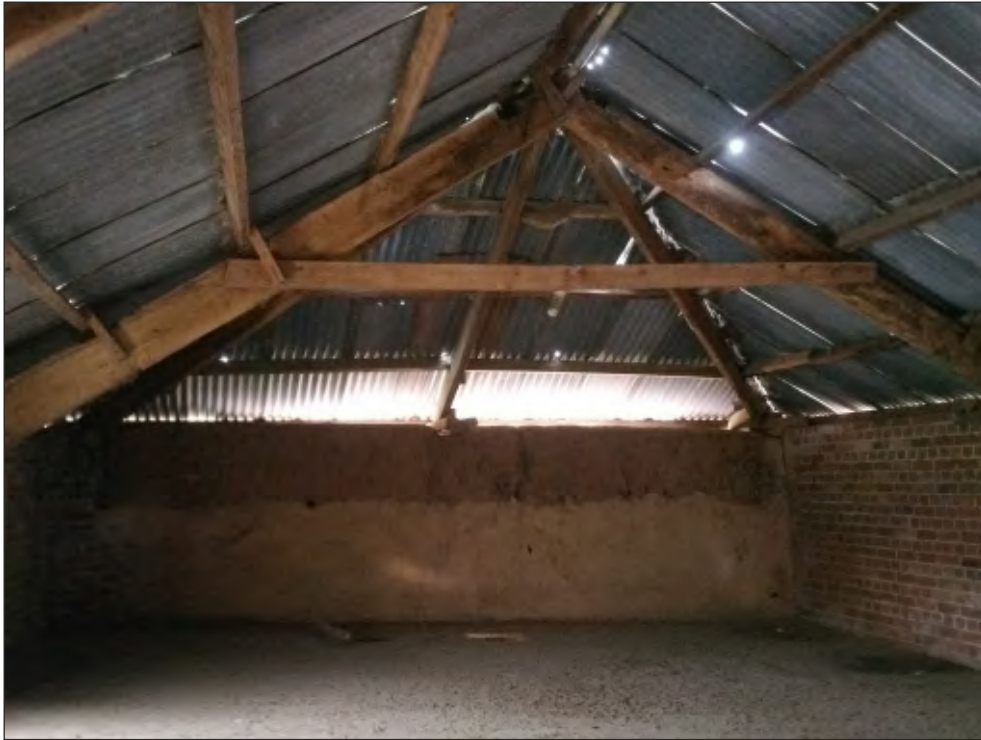
Fig. 23 General view of eastern end showing original cob elevation and later brick re-fronting. Looking east.
