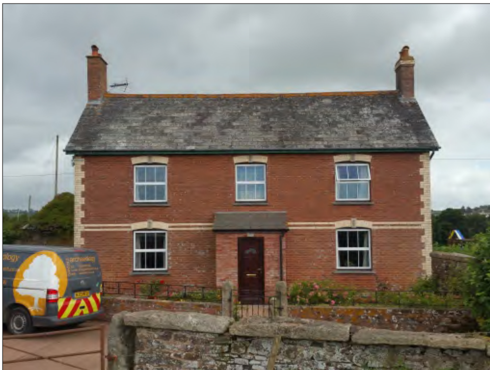
Fig. 7 General view of early 20th century farmhouse. Looking north.
