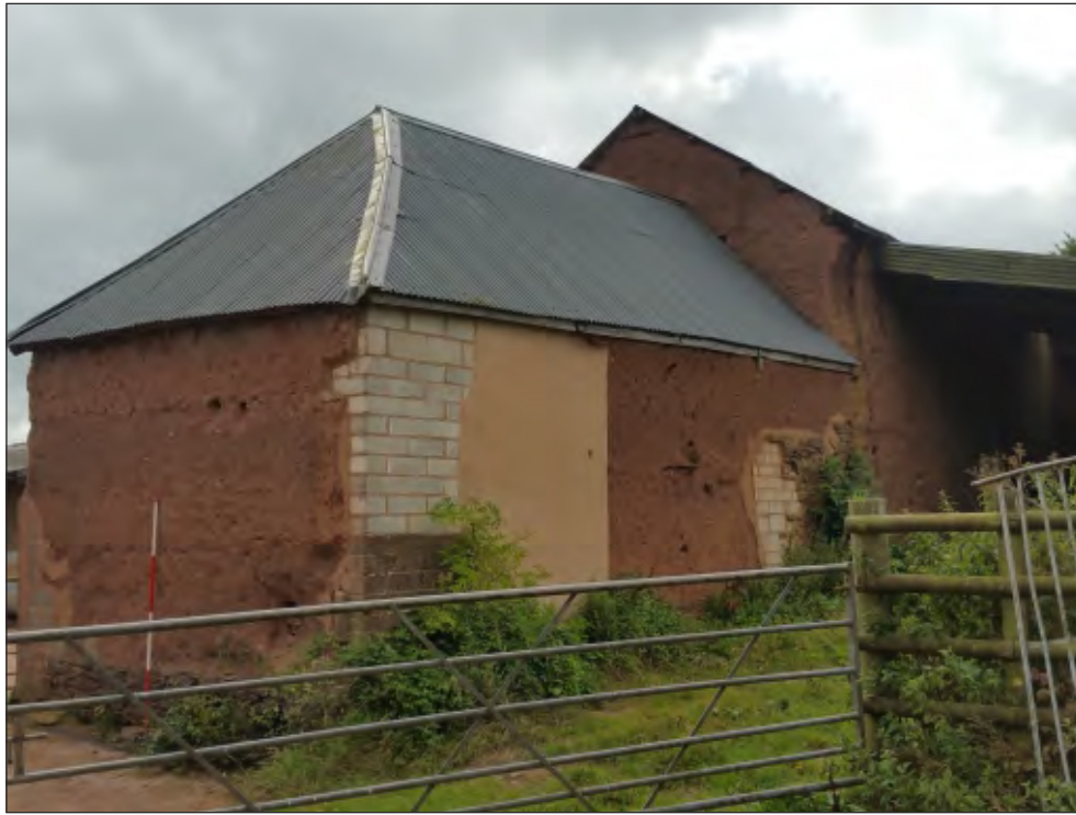
Fig. 45 General view of rear elevation of linhay. 2m scale. Looking southeast.
