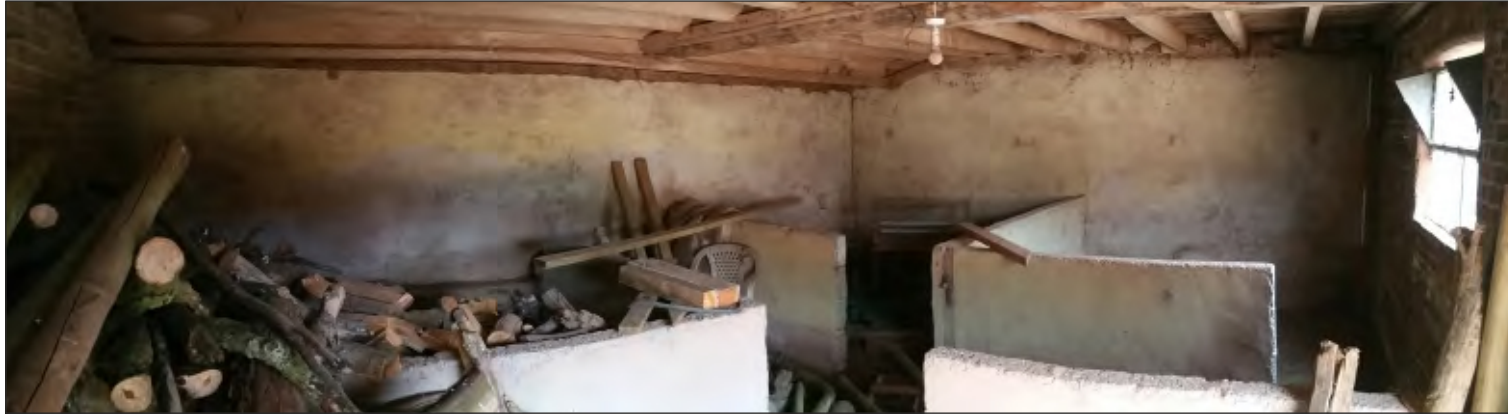
Fig.16 General view of central room with feeding hatch in rear elevation. Looking northeast.
