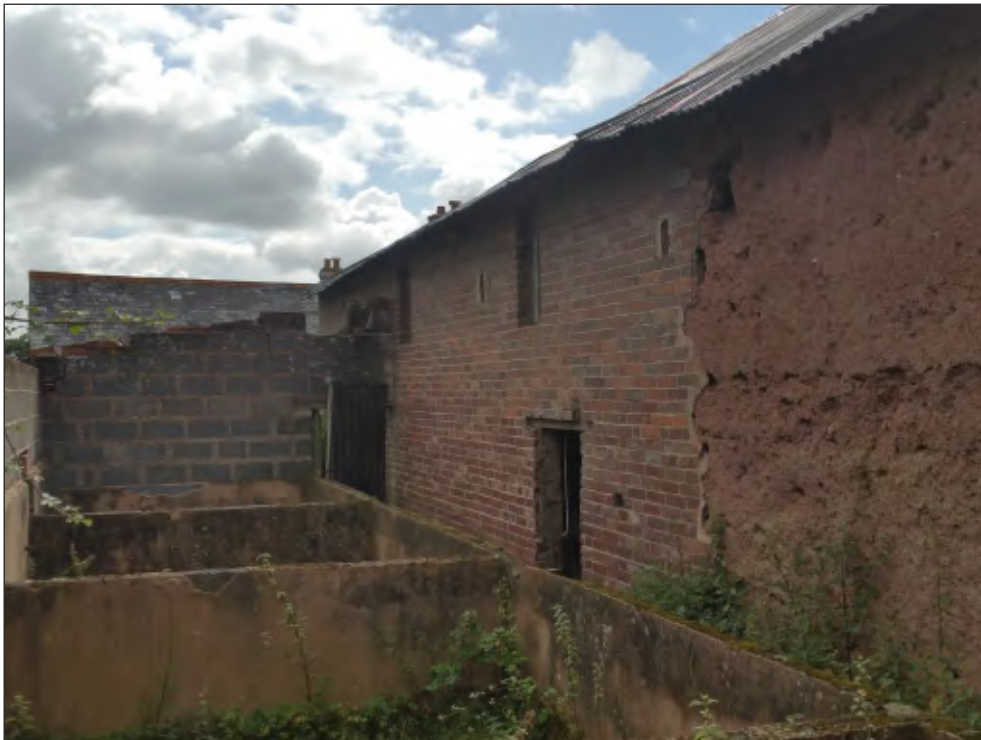
Fig. 15 General view of rear elevation showing rebuilt section. Looking southeast.
