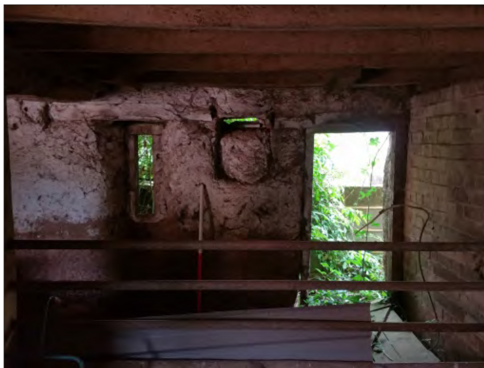
Fig. 20 General view of window and door arrangement. 1m scale. Looking north.
