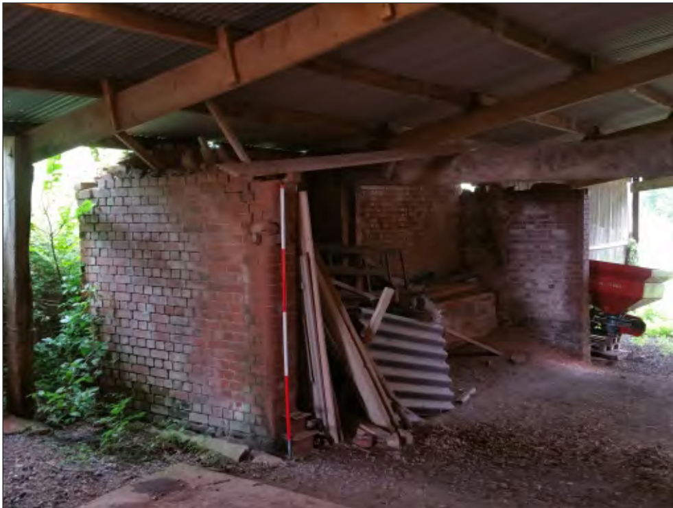
Fig. 34 General view of structure at rear of threshing barn. 2m scale. Looking northwest.
