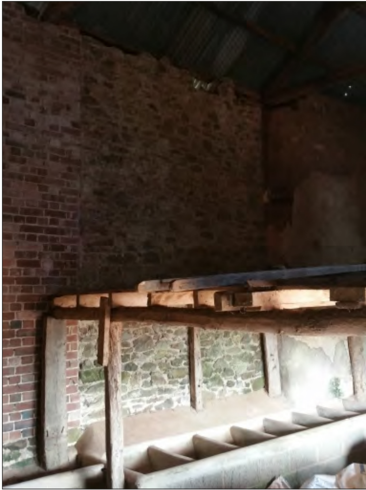
Fig. 43 General view of blocked doorway in lower threshing barn. Looking northwest.
