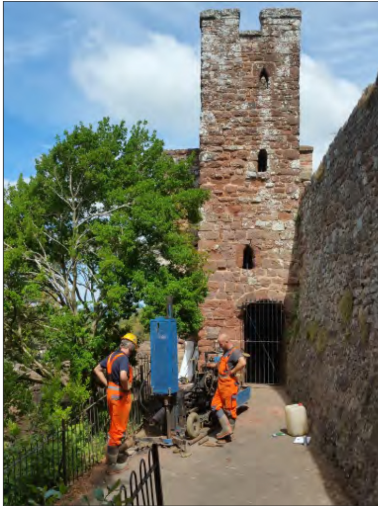
Pl. 1 Excavating Borehole 1 using a tracked percussive auger rig. Looking northwest.
