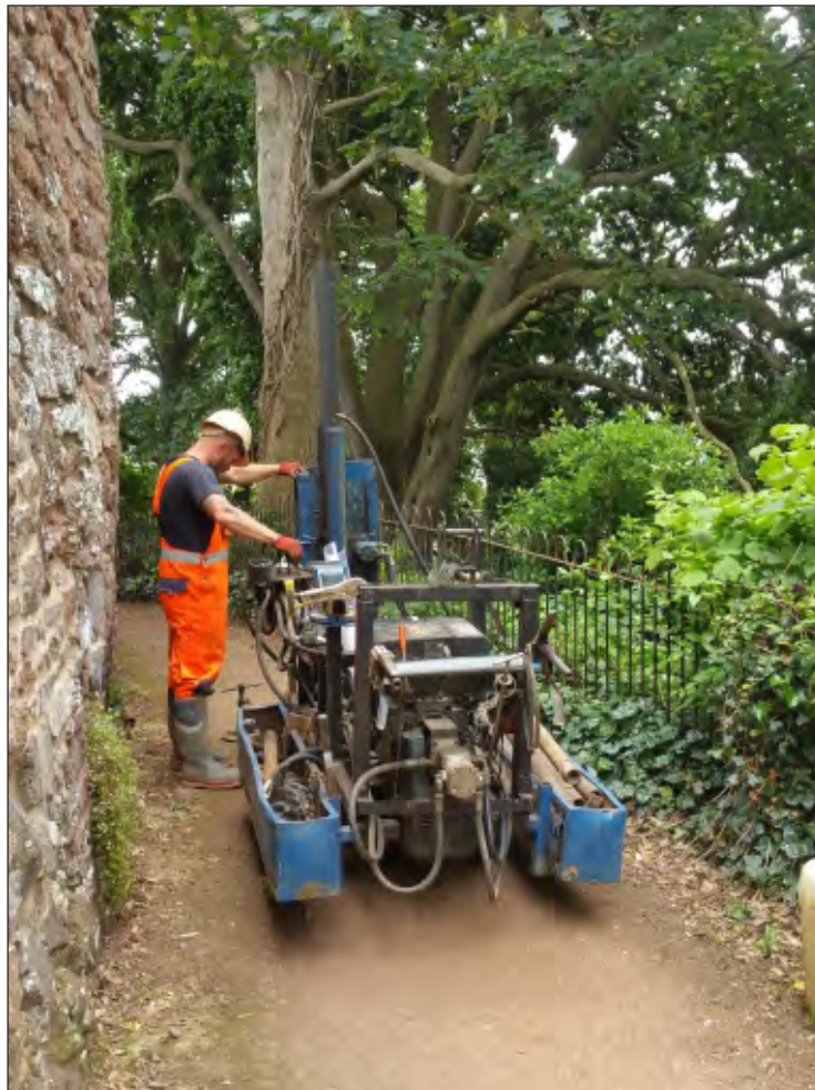
Pl. 12 Excavating Borehole 7 using a tracked percussive auger rig. Looking southeast.
