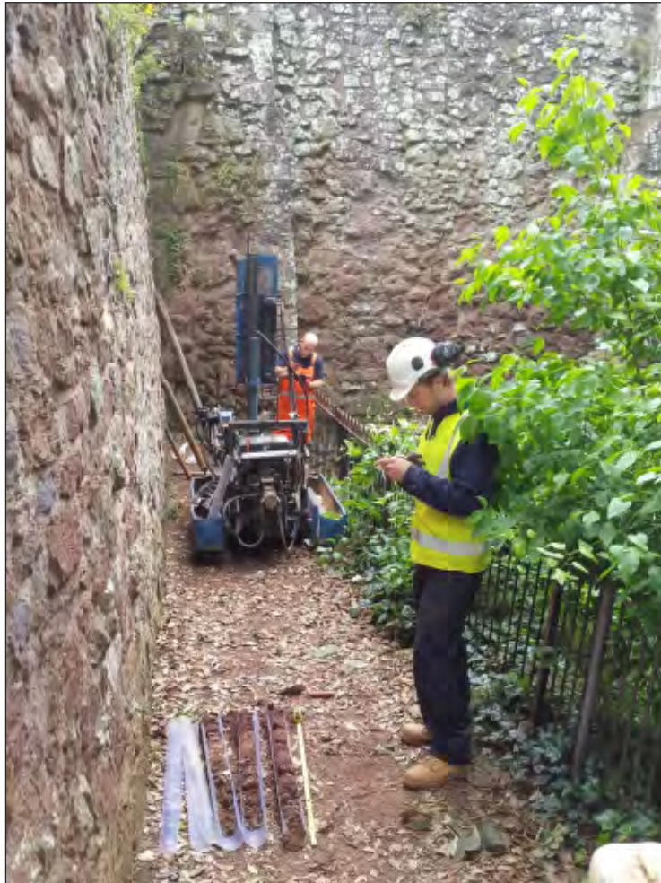
Pl. 17 Excavating Borehole 10 using a tracked percussive auger rig. Looking northeast.
