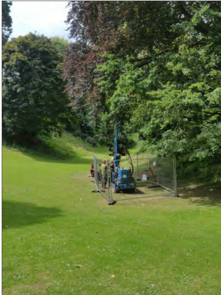
Pl. 15 General view of tracked percussive auger rig excavating Borehole 9. Looking west.
