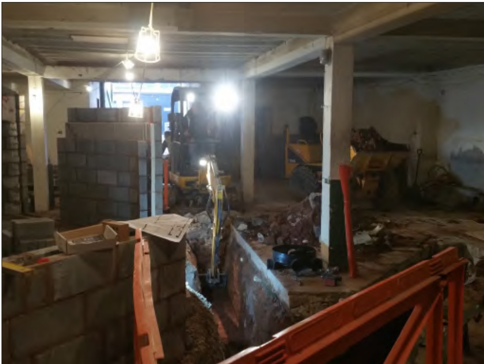
Pl. 4 General view of site. Looking northwest.
