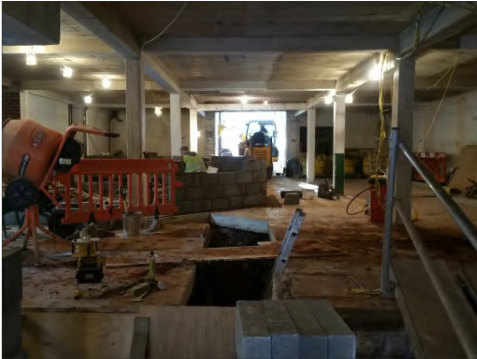
Pl. 1 General view of site. Looking northwest.
