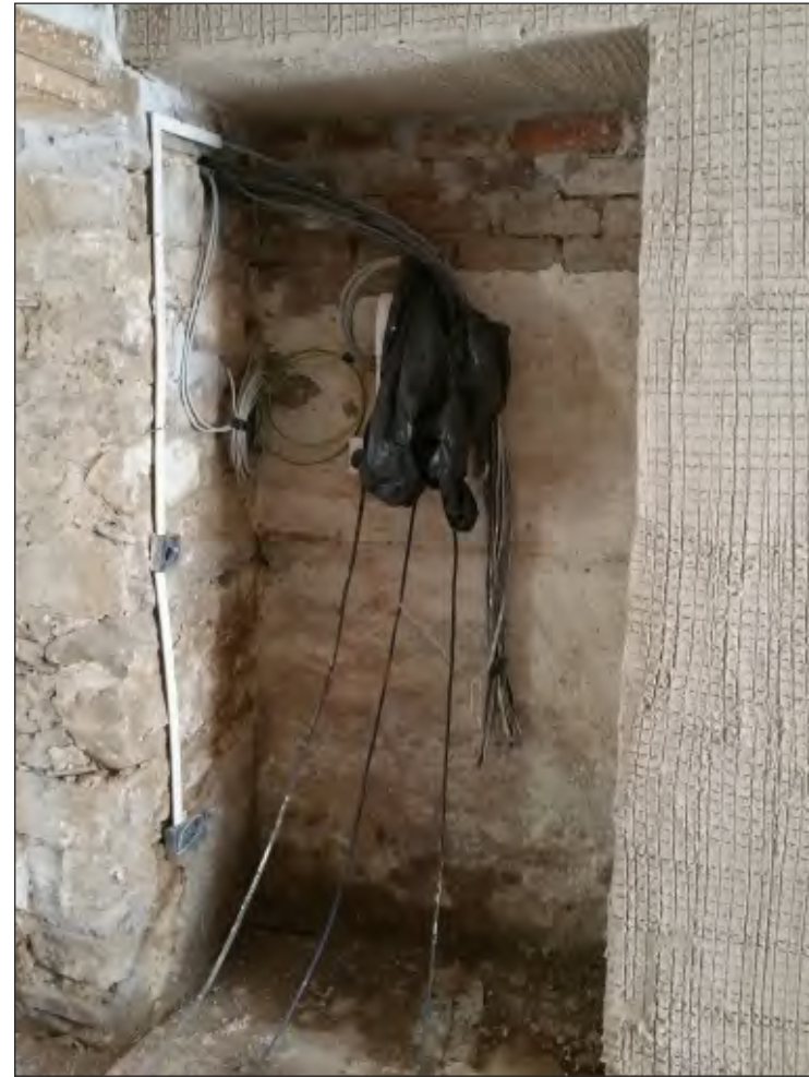
Pl. 18 General view of blocked doorway in north-eastern corner of room G6 showing late 19th century brick blocking. Looking northeast.
