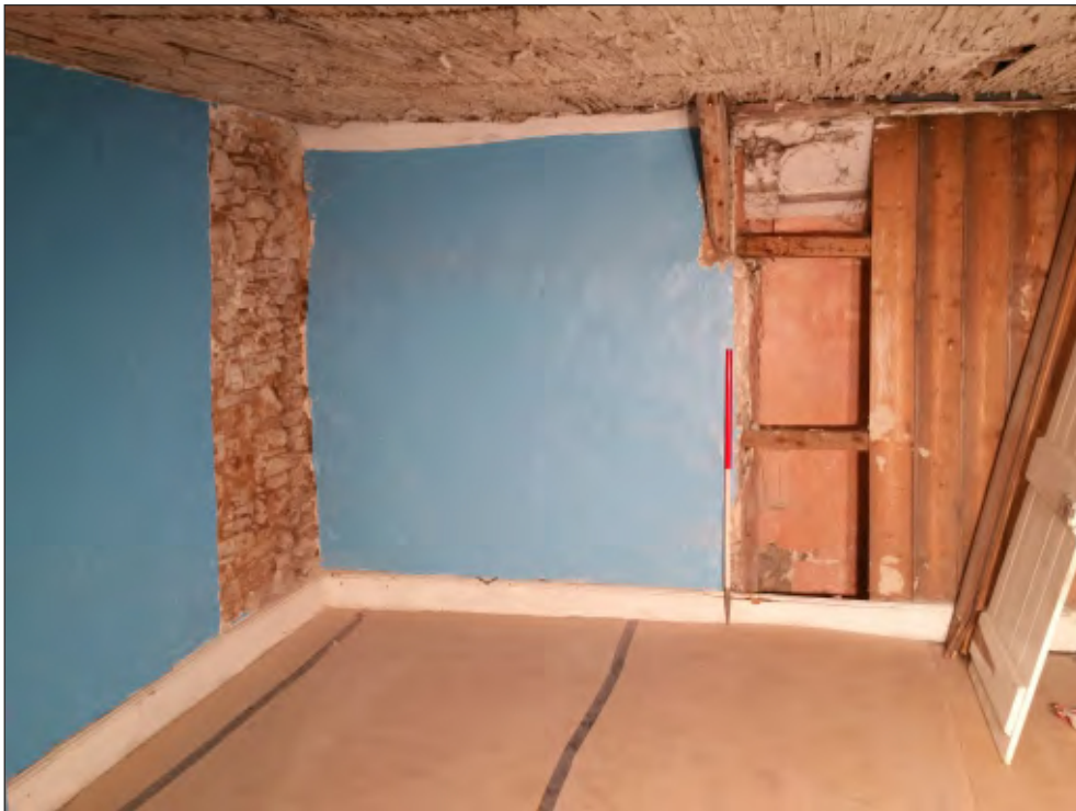
Pl. 26 General view of room F6 showing newel stair in north-eastern corner. 1m scale. Looking north.
