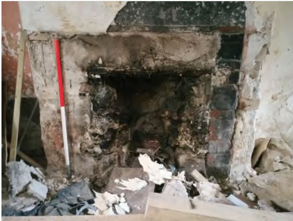
Pl. 10 General view of fireplace in room G4 showing stone jamb (right) of medieval fireplace. 1m scale. Looking west.
