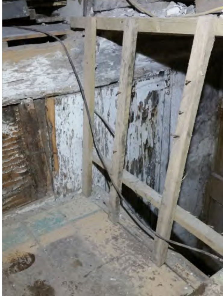
Pl. 9 Close-up of random door in partition between corridor G3 and room G4 and partially obstructed by late 19th century staircase. Looking northwest.
