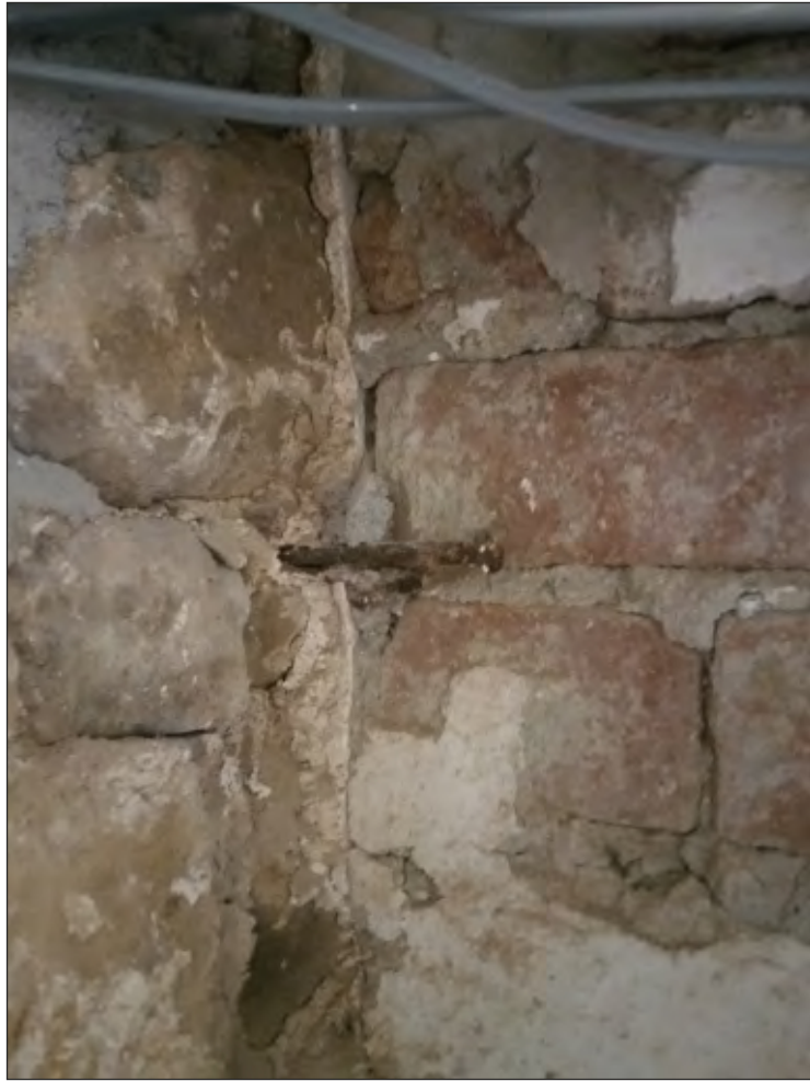
Pl. 19 Close-up showing later brick blocking of doorway in east elevation of room G6 butting up to earlier plaster. Looking northeast.
