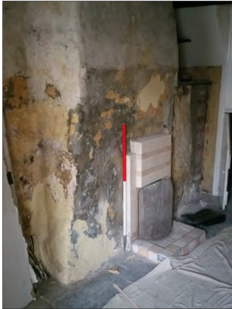
Pl. 21 General view of fireplace in room G2. 1m scale. Looking northwest.
