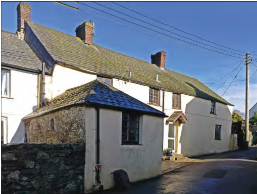
Pl. 1 General view of the main facade of Staddons prior to removal of external render. Looking northeast.
