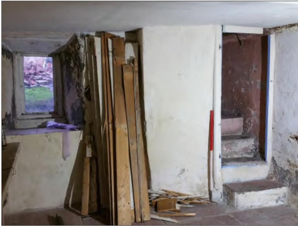
Pl. 11 General view of the newel stair in northeast corner of room G4. 1m scale. Looking northeast.
