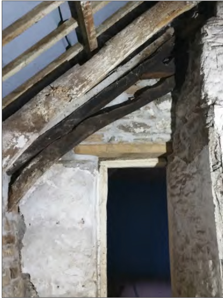
Pl. 31 General view of medieval roof truss. Looking east.
