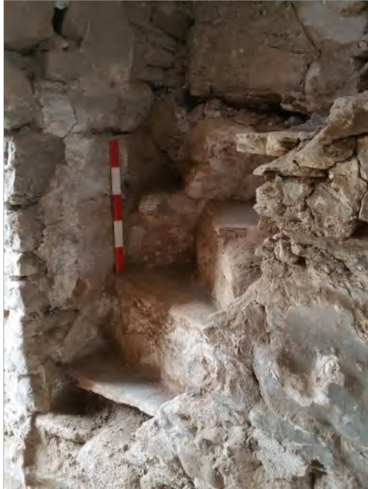
Pl. 13 General view of medieval stair revealed following the removal of the late 19th century staircase. 0.5m scale. Looking northeast.
