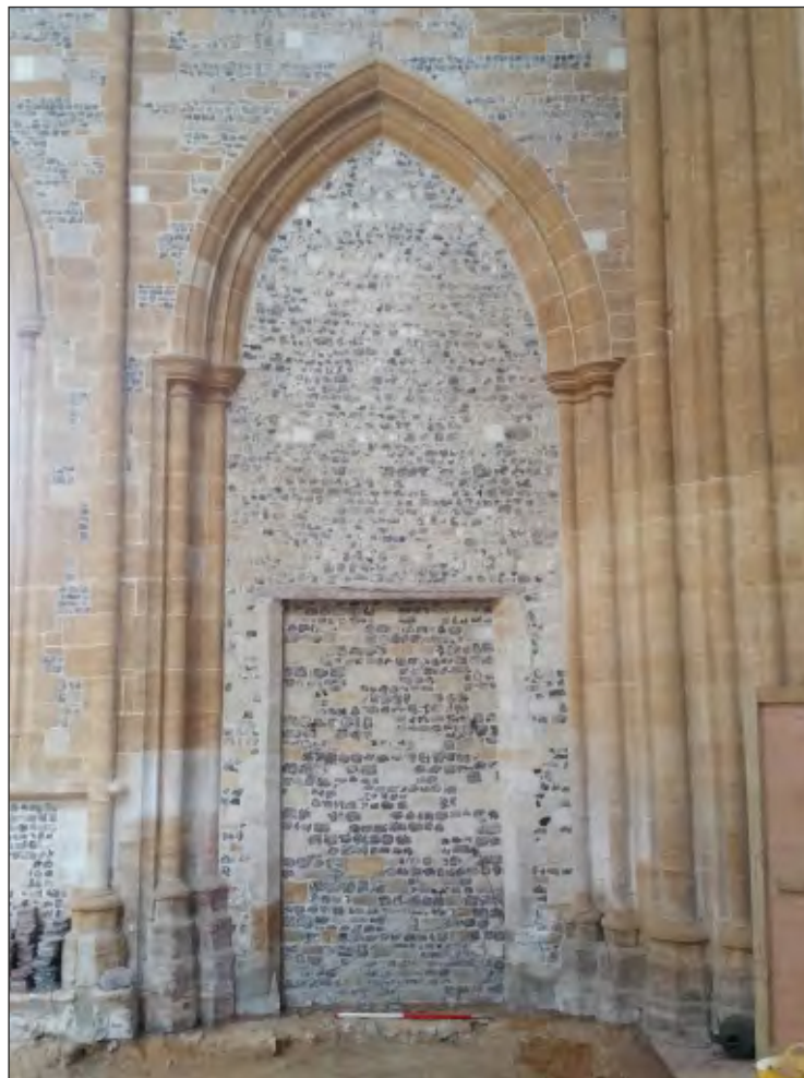
Pl. 10 General view of south nave aisle opening showing pier foundations (1018) and 1020) and foundation (1023) of door blocking (1024).
