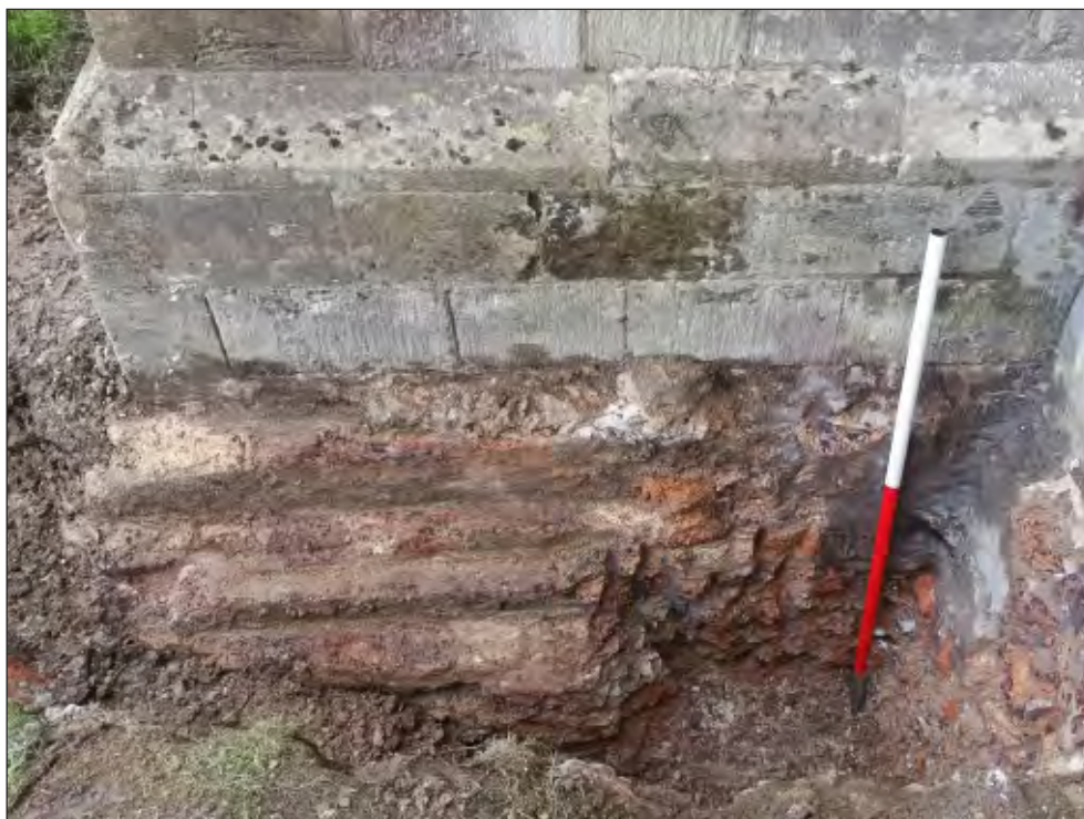
Pl. 21 Close-up of post-medieval underpinning of buttress on north elevation. 1m scale. Looking east.
