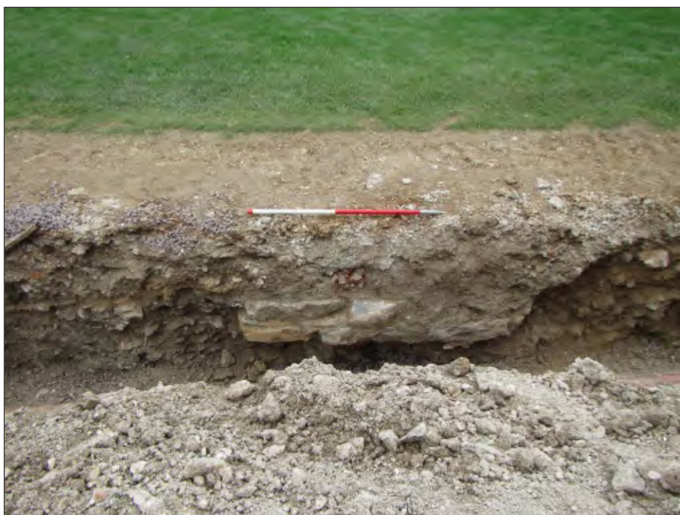
Pl. 14 Close-up showing foundation (2013), main wall (2014) and buttress foundation (2015). 1m scale. Looking east.
