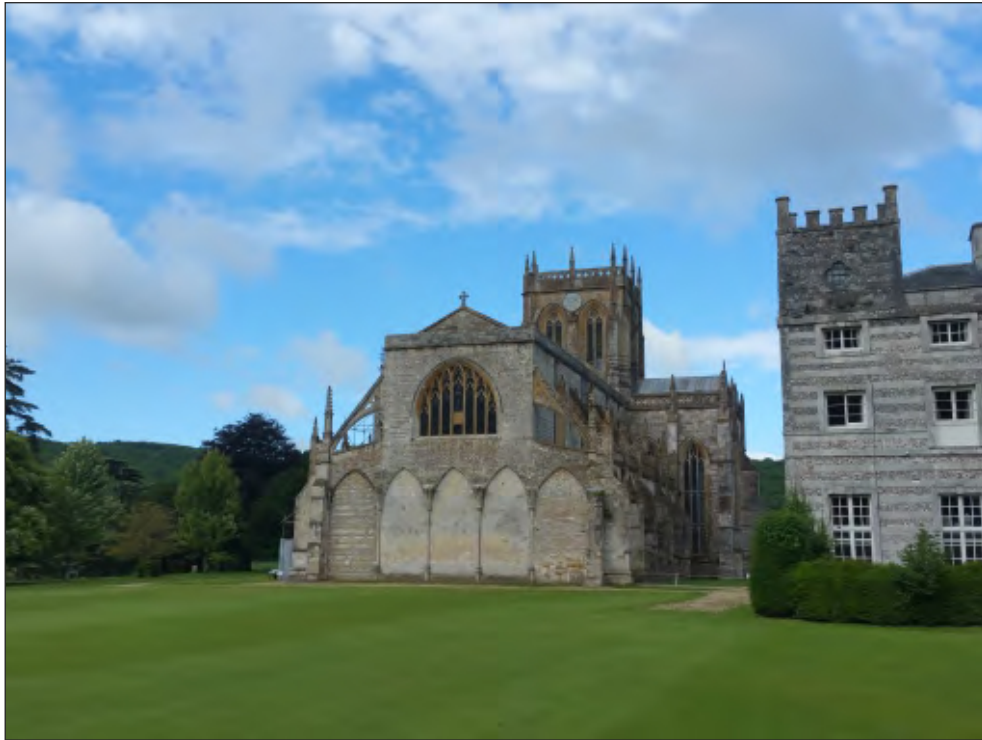
Pl. 3 General view of east end showing location of demolished Lady Chapel. Looking southwest.
