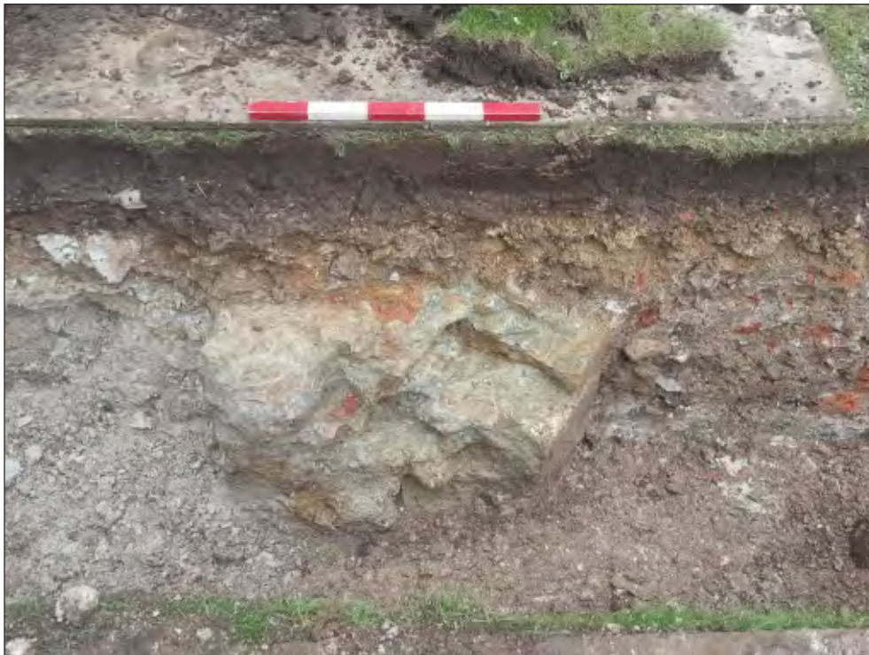
Pl. 20 Close-up of late 16th-mid 18th century wall foundation (2066). 0.5m scale. Looking west.
