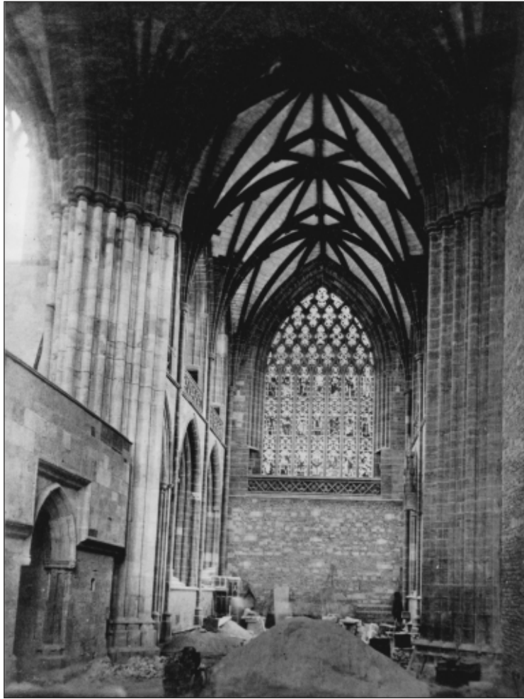
Fig. 8 Photograph of the crossing and south transept taken in 1865 during George Gilbert Scott's restoration of the church. Looking south.
