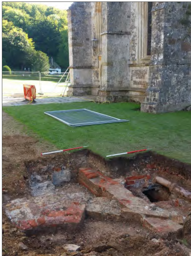
Pl. 18 General view of late 17th- 18th century wall (2052) and late 19th century conservatory wall (2055). 1m scales. Looking east.
