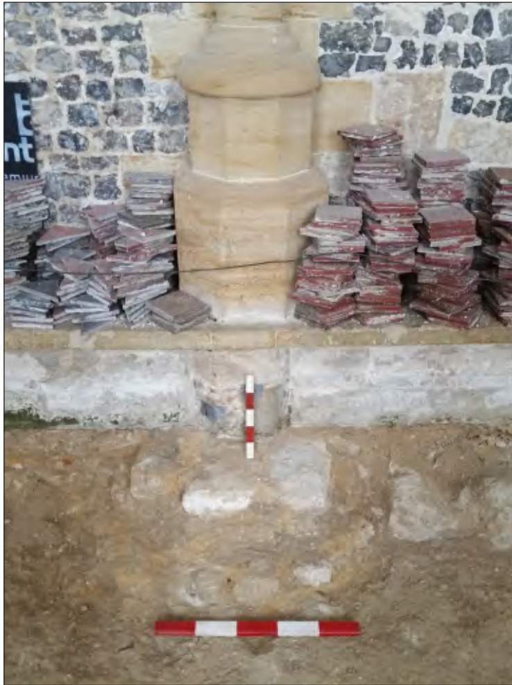
Pl. 7 Close-up showing stone rubble and clay foundations (1010) of east elevation south transept. 0.25m and 0.5m scales. Looking east.
