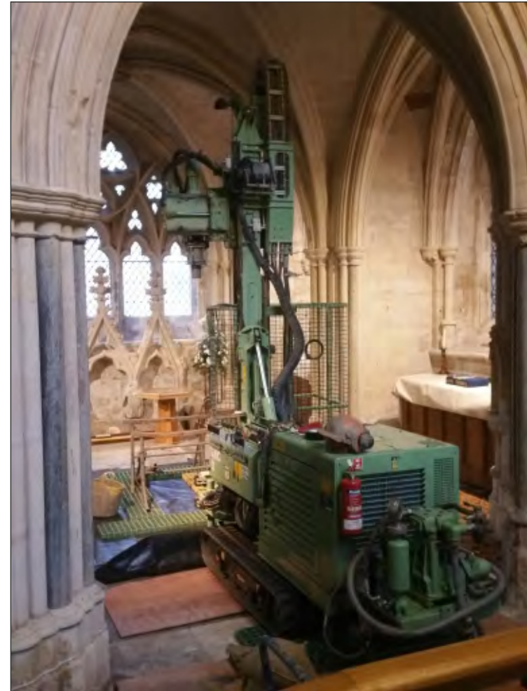
Pl. 10 General view of percussive auger rig excavating Borehole 5. 1m scale. Looking northeast.
