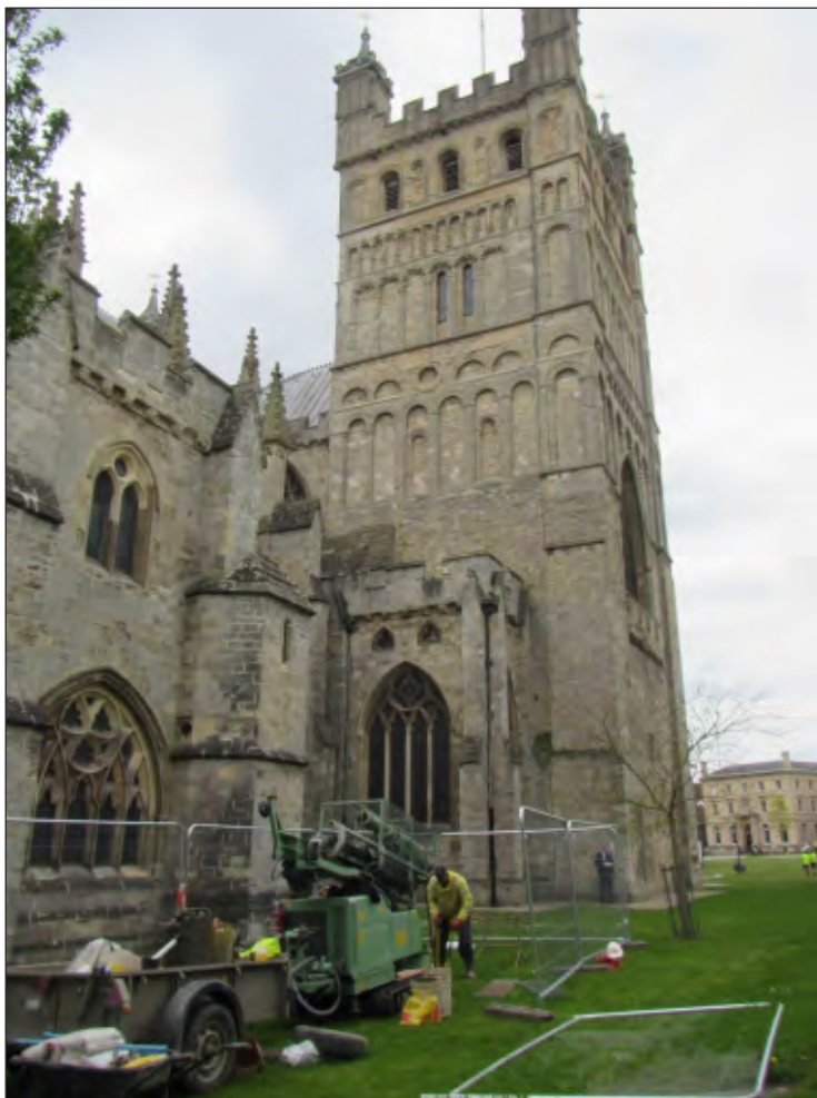
Pl. 7 General view of tracked percussive auger rig excavating Borehole 4. Looking southwest.
