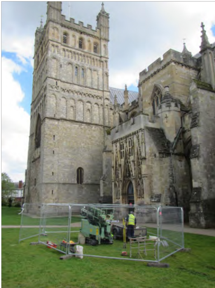
Pl. 3 General view of tracked percussive auger rig excavating Borehole 2. Looking southeast.
