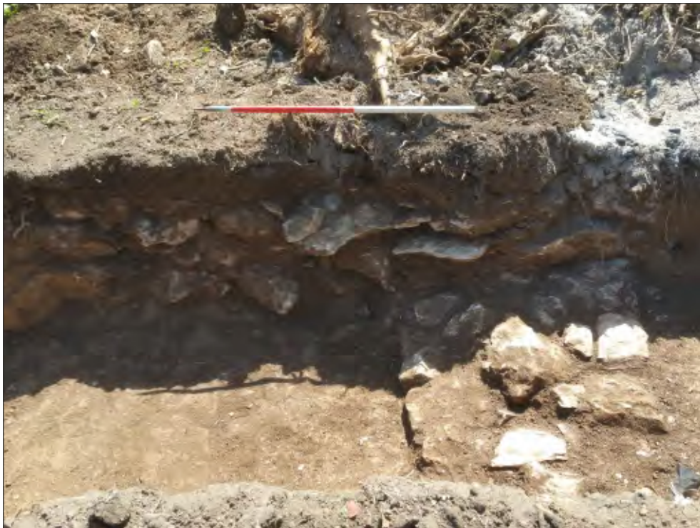
Pl. 2 General view of wall foundation (103). 1m scale. Looking south.
