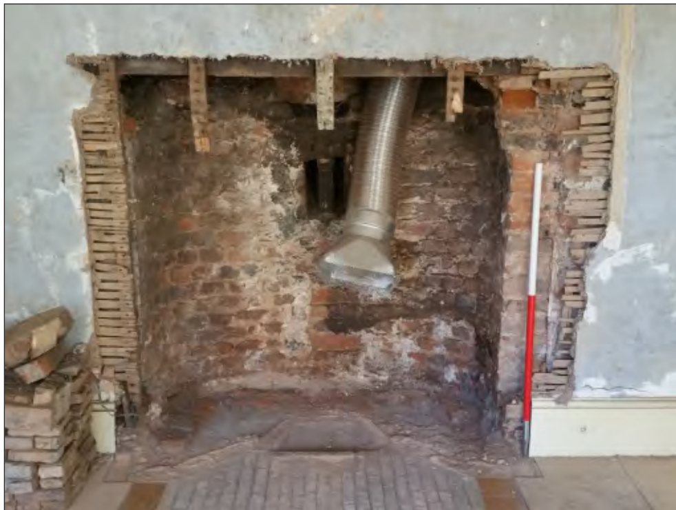
Pl. 20 General view of early-to-mid 18th century 'Dutch' style fireplace with curved sides and rear. 1m scale. Looking northwest.
