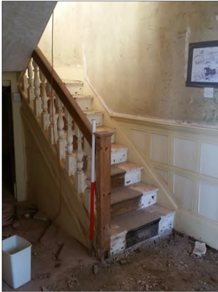
Pl. 17 General view of main staircase. 1m scale. Looking north.
