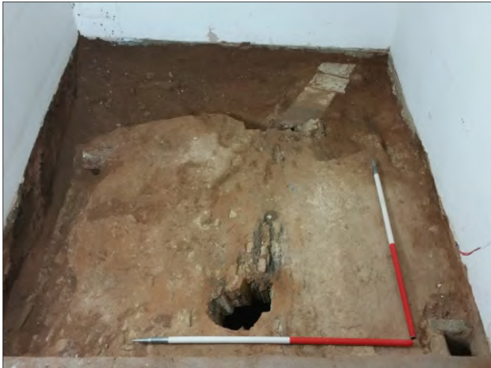
Pl. 22 Cistern and drain (top right) uncovered during work in ground-floor room G09. 1m scales. Looking northeast.
