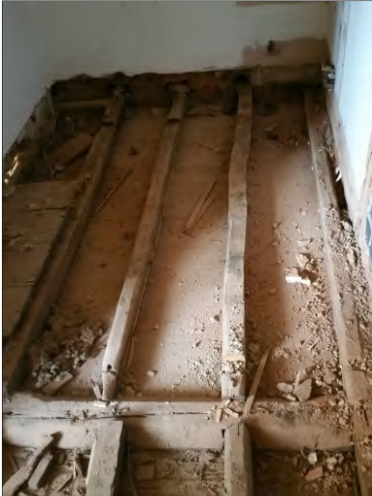
Pl. 33 Position of rear stair within first-floor room F05. Looking northwest.
