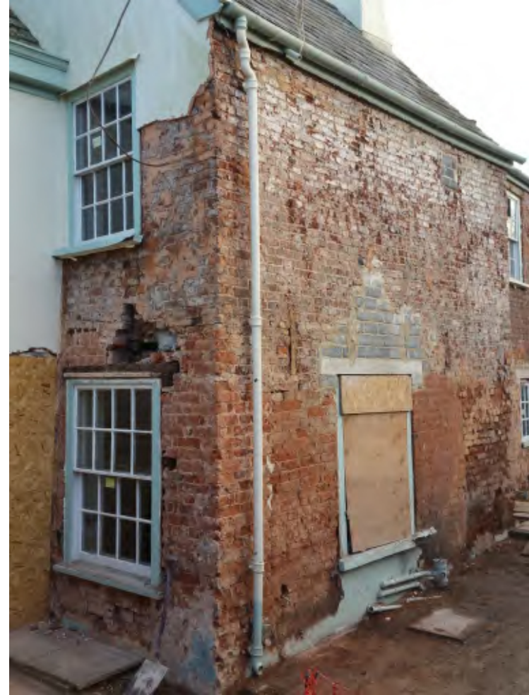
Pl. 4 General view of Kitchen block showing 18th and 19th century alterations to the window openings. Looking northeast.
