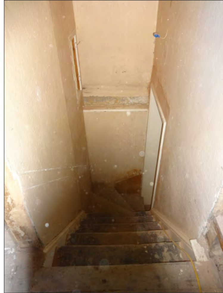
Pl. 34 General view of modern stair within rear range. Looking northwest.
