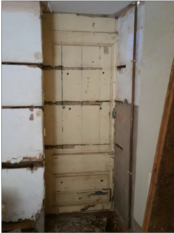
Pl. 21 17th-century panelling re-used in alcove in ground-floor room G06. Looking west.
