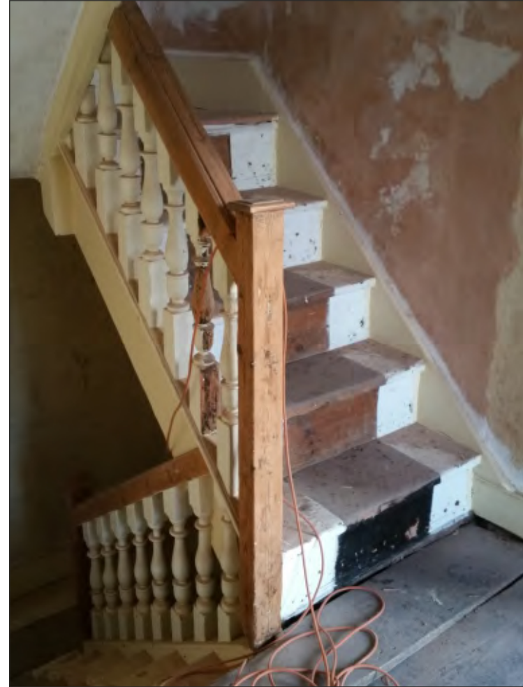
Pl. 24 General view of main stair on first-floor landing. Looking northeast.
