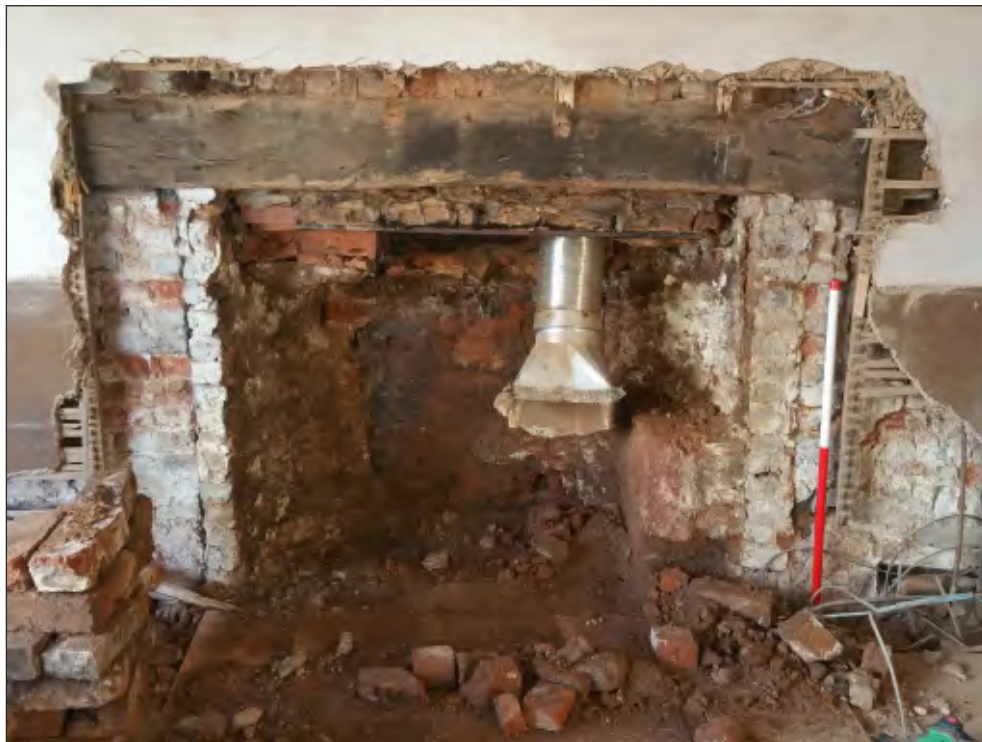
Pl. 12 General view of late 17th or early 18th century 'Dutch' style fireplace with curved sides and back. 1m scale. Looking northwest.
