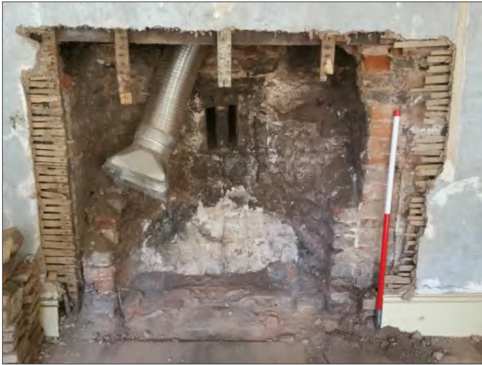
Pl. 19 General view of mid-to-late 18th century 'Dutch' style fireplace with curved sides and rear. 1m scale. Looking northwest.
