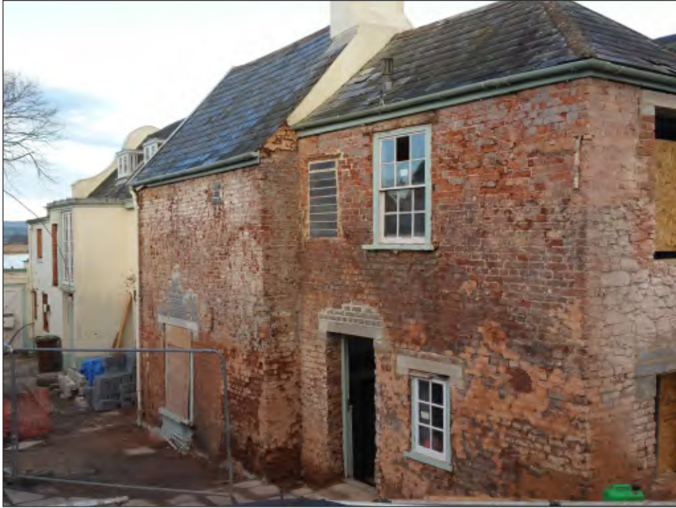
Pl. 5 General view of Kitchen block and rear building. Looking northwest.
