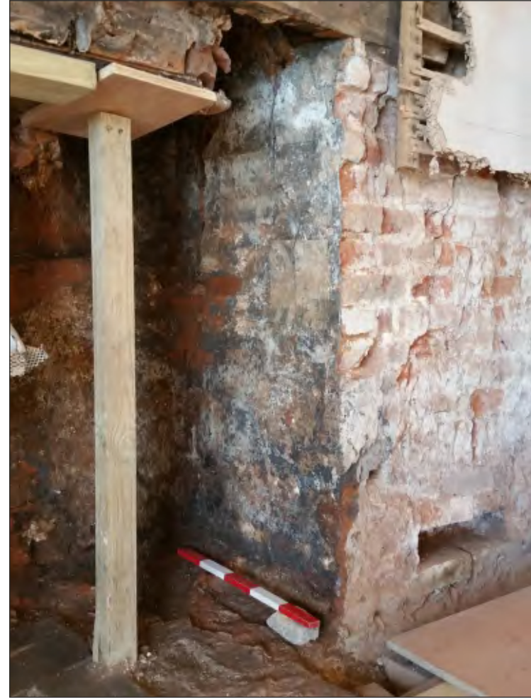
Pl. 14 Close-up of eastern jamb of fireplace showing black-and-white chequerboard painted plaster decoration. 0.5m scale. Looking north.
