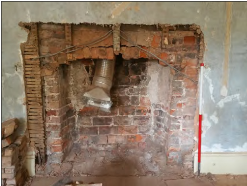
Pl. 18 General view of late 18th or early 19th century fireplace in ground-floor room G05 following removal of modern fireplace. 1m scale. Looking northwest.
