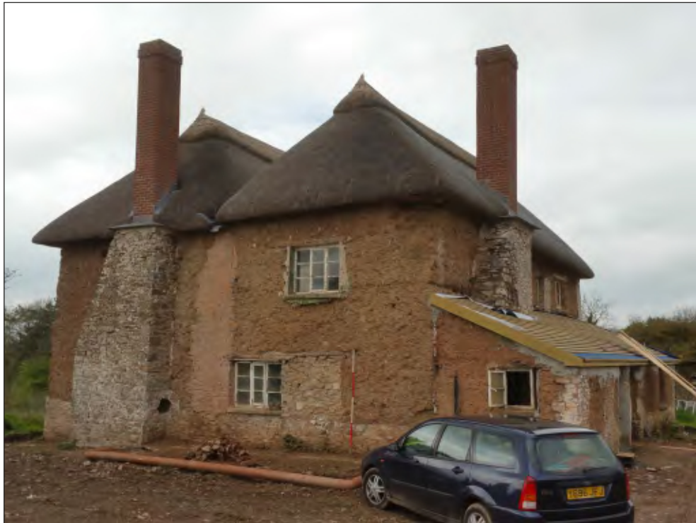
Pl. 3 General view of east elevation showing window arrangement and early 19th century outshuts. 2m scale. Looking west.
