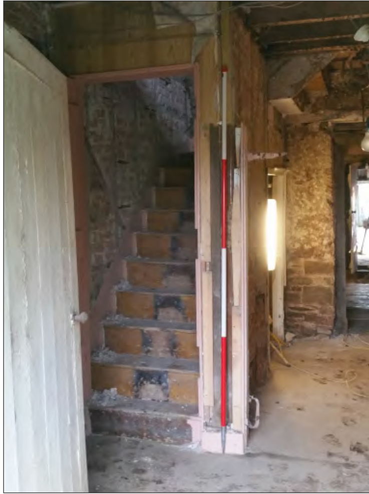
Pl. 5 General view of entrance hall G01 showing original through passage and main stair. 2m scale. Looking north.
