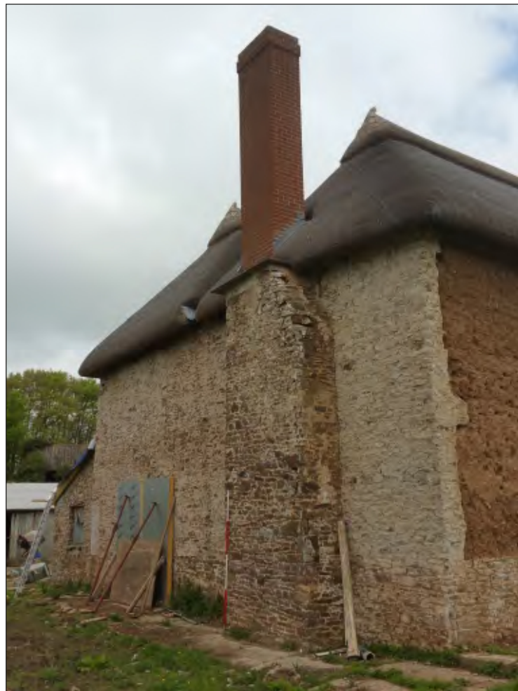
Pl. 2 General view of western elevation showing chimneystack. 2m scale. Looking northeast.
