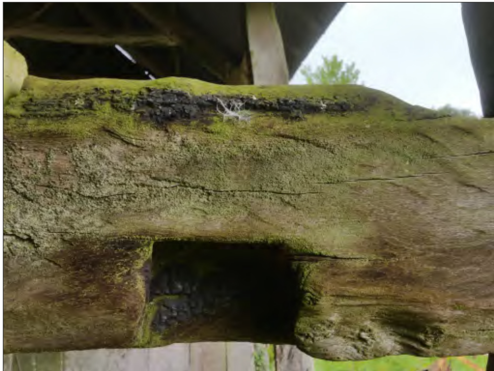
Pl. 26 Close-up of re-used timber within Linhay showing traces of burning. Looking north.
