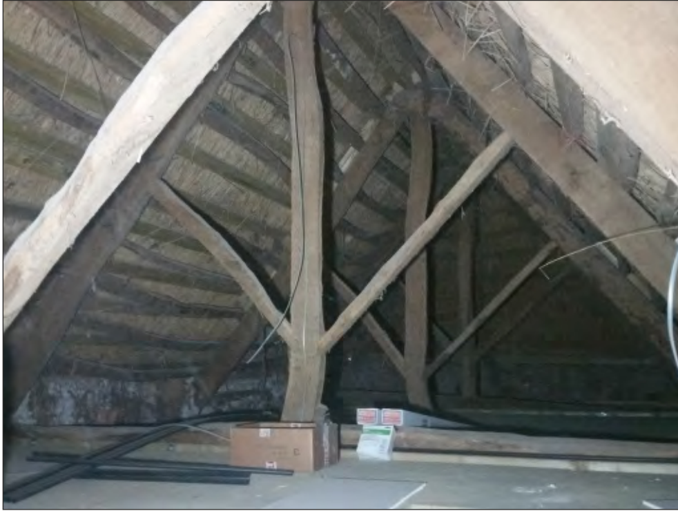
Pl. 23 General view of roof arrangement. Looking northeast.
