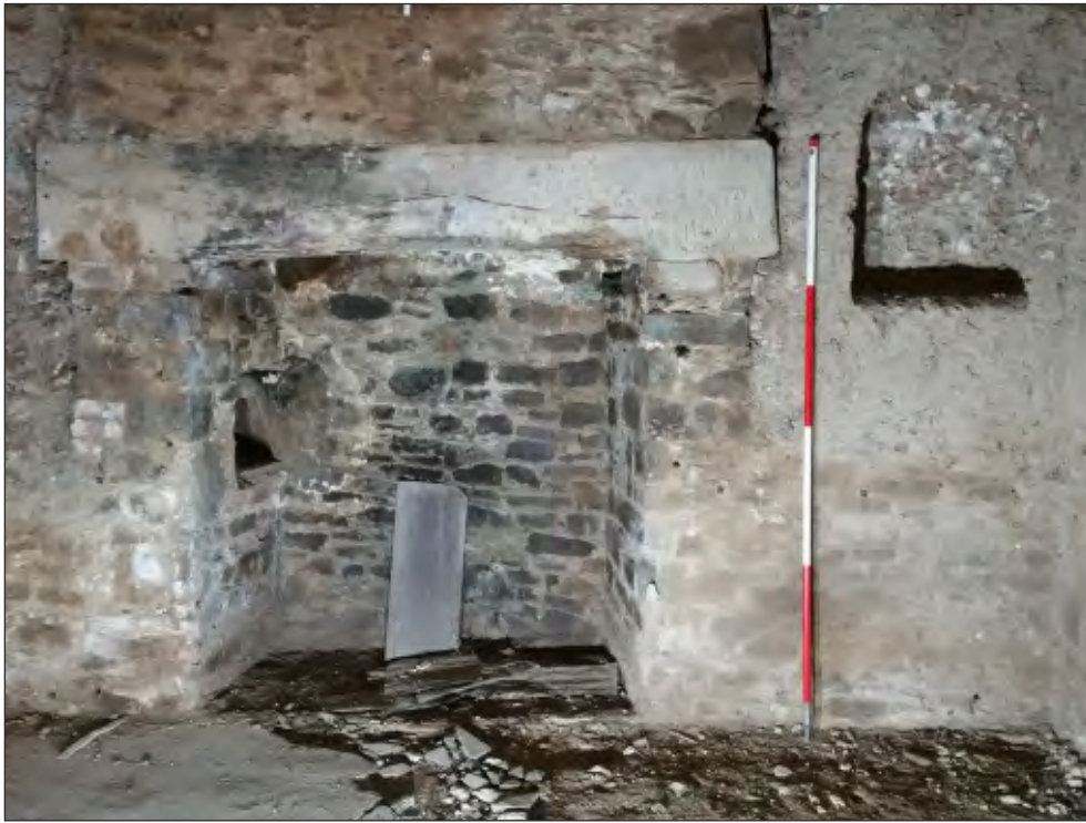
Pl. 9 General view of east elevation ground-floor room G03 showing fireplace with re-used lintel, inserted cloam oven and high-level cupboard. 2m scale. Looking east
