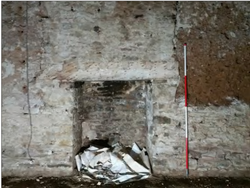
Pl. 7 General view of west elevation ground-floor room G02 showing fireplace with re-used lintel. 2m scale. Looking west.
