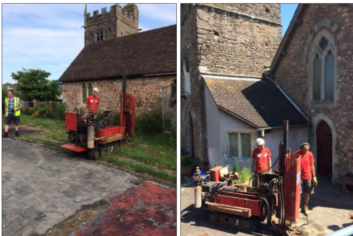
Fig. 2 Plan showing location of observations and photos showing drilling of borehole 2 (left) and borehole 4 (right).
