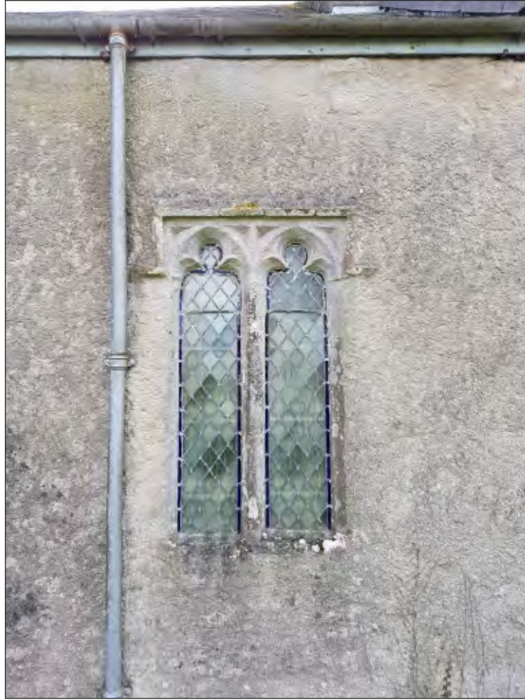
Pl. 22 General view of 14th century window with squared head and hood mould, St Mary, Rattery.
