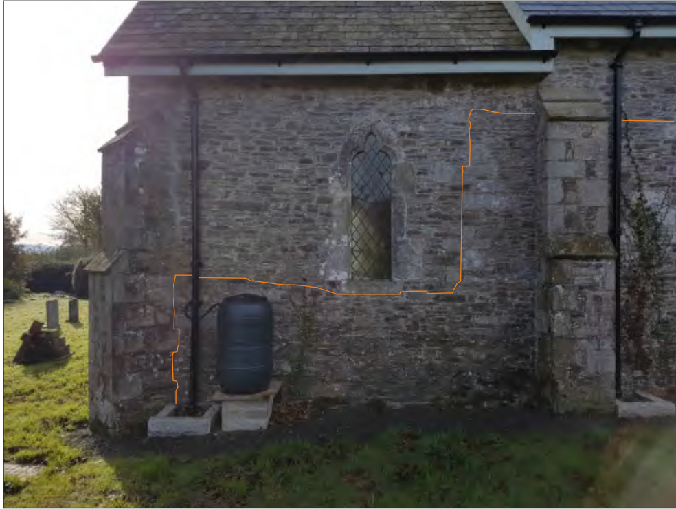
Pl. 16 General view of north elevation showing sections rebuilt in the late 19th century. Looking south.
