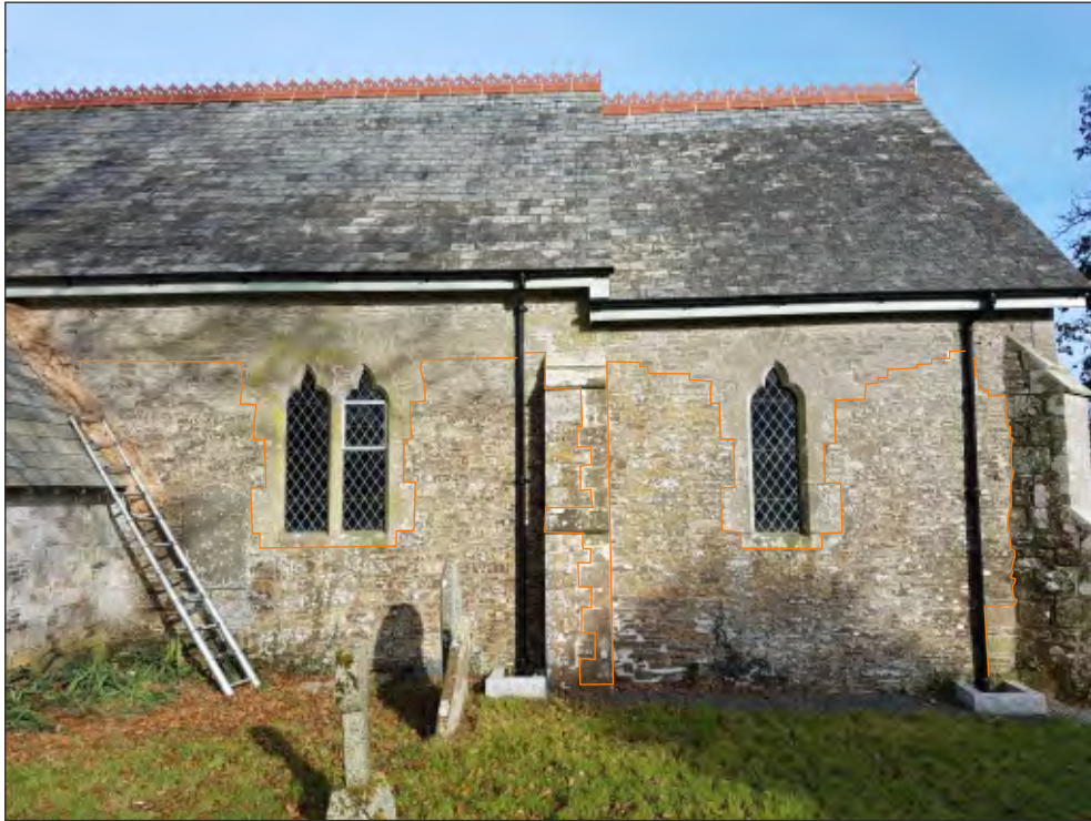
Pl. 14 General view of south elevation showing sections rebuilt in the late 19th century. Looking north.
