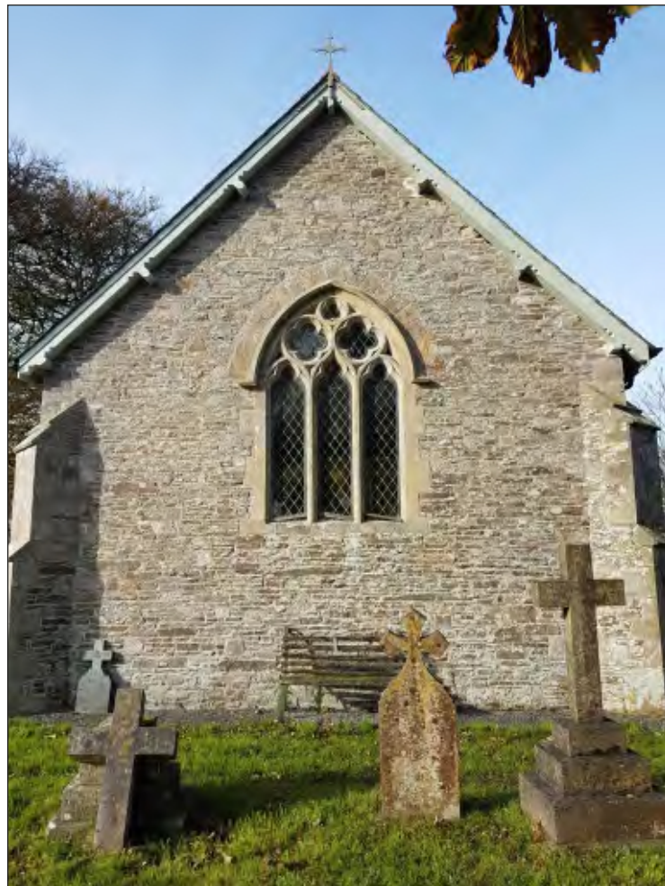
Pl. 15 General view of east end as rebuilt in 1871. Looking west.
