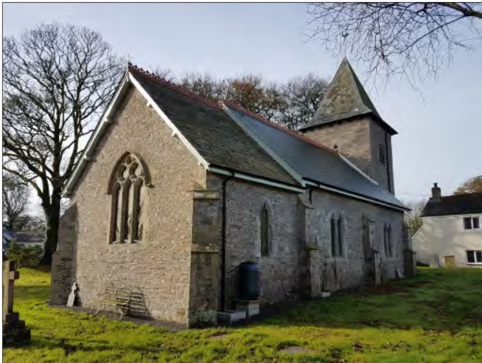
Pl. 2 General view of St Alban's Church, Beaworthy. Looking southwest.
