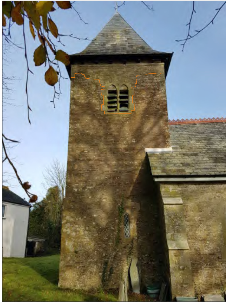
Pl. 12 General view of church tower showing 19th century rebuild (top). Looking north.
