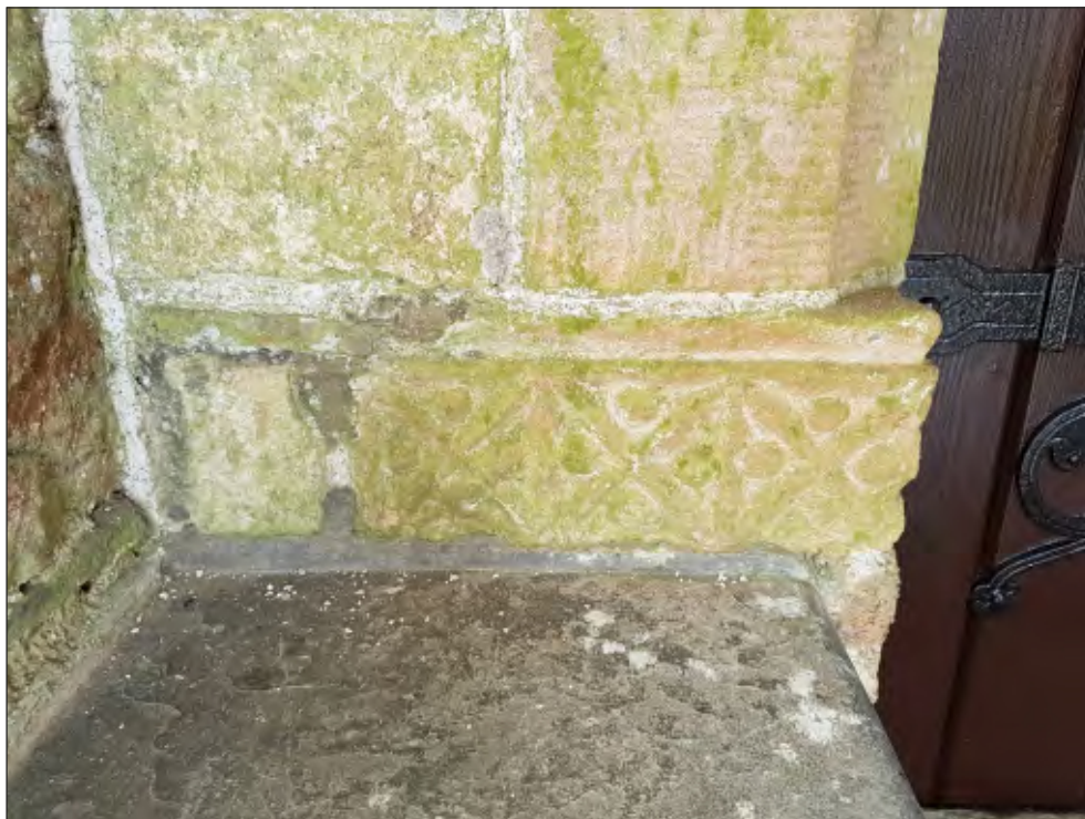
Pl. 5 Close-up of possible western capital head. Looking north.
