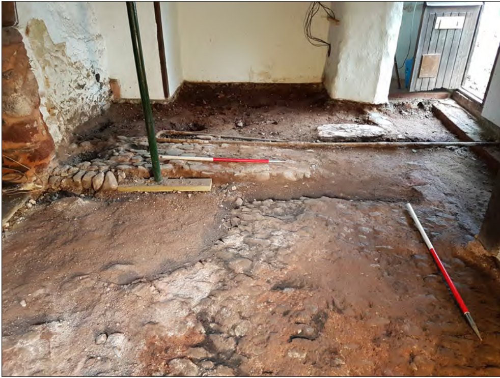
Pl. 3 General view of ground-floor showing heavily disturbed cobbled floor. 1m scales. Looking north.
