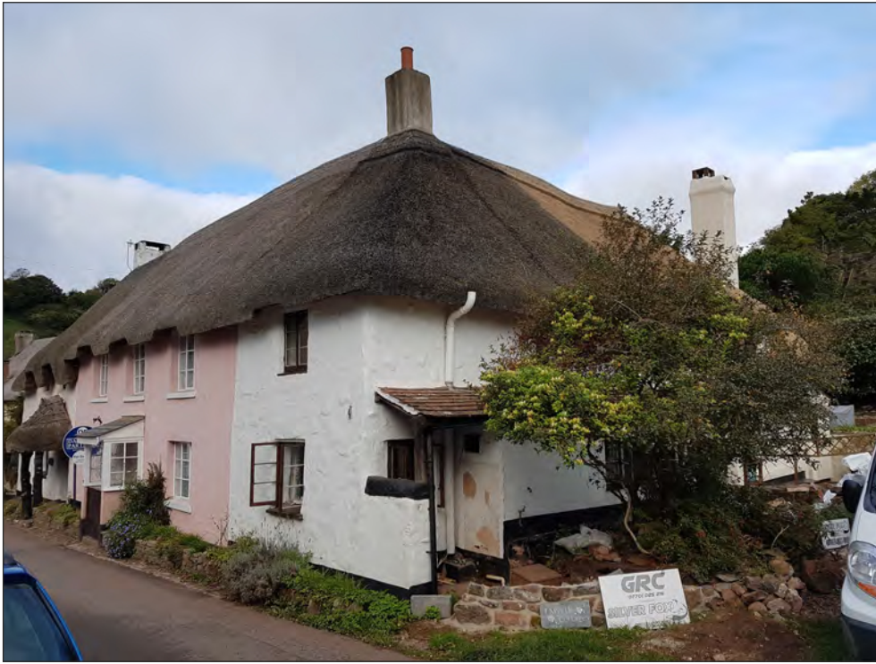
Pl. 1 General view of Mole End, Dean Cottage and No. 1 Myrtle Cottage. Looking northwest.
