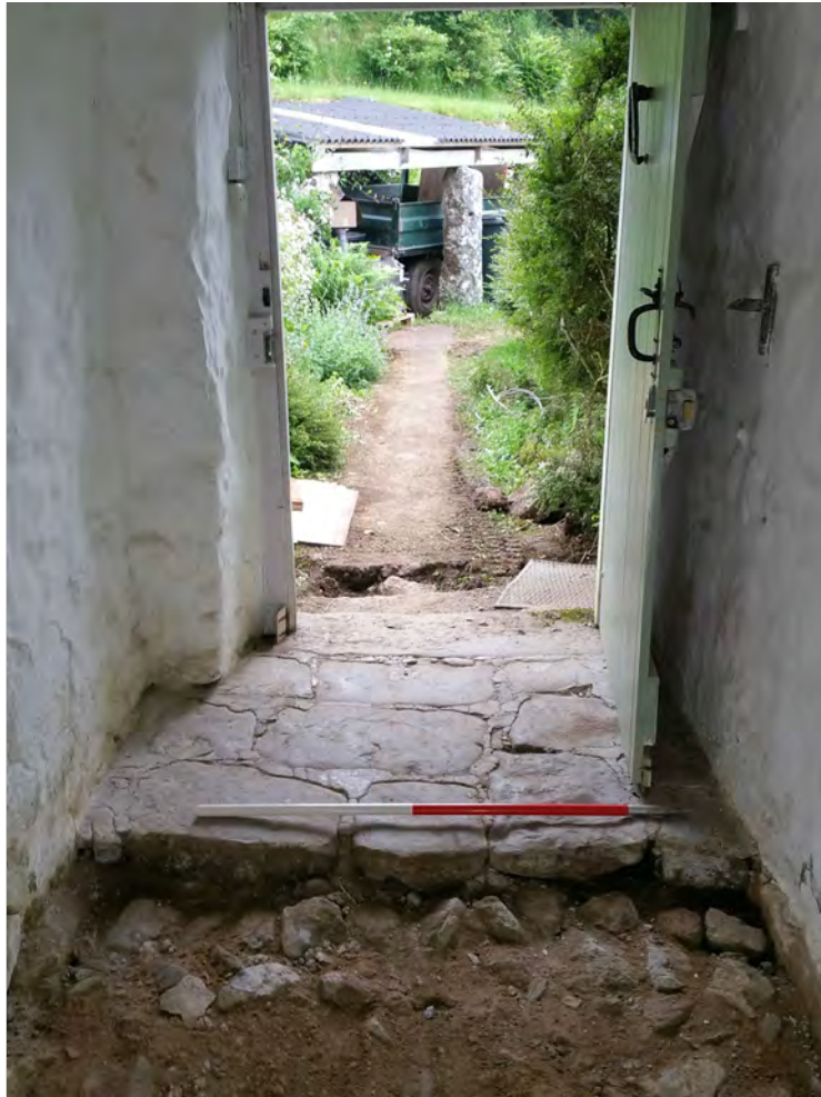
Pl. 1 General view of cross-passage showing disturbed granite cobbles underneath later floor surface. 1m scale. Looking east.
