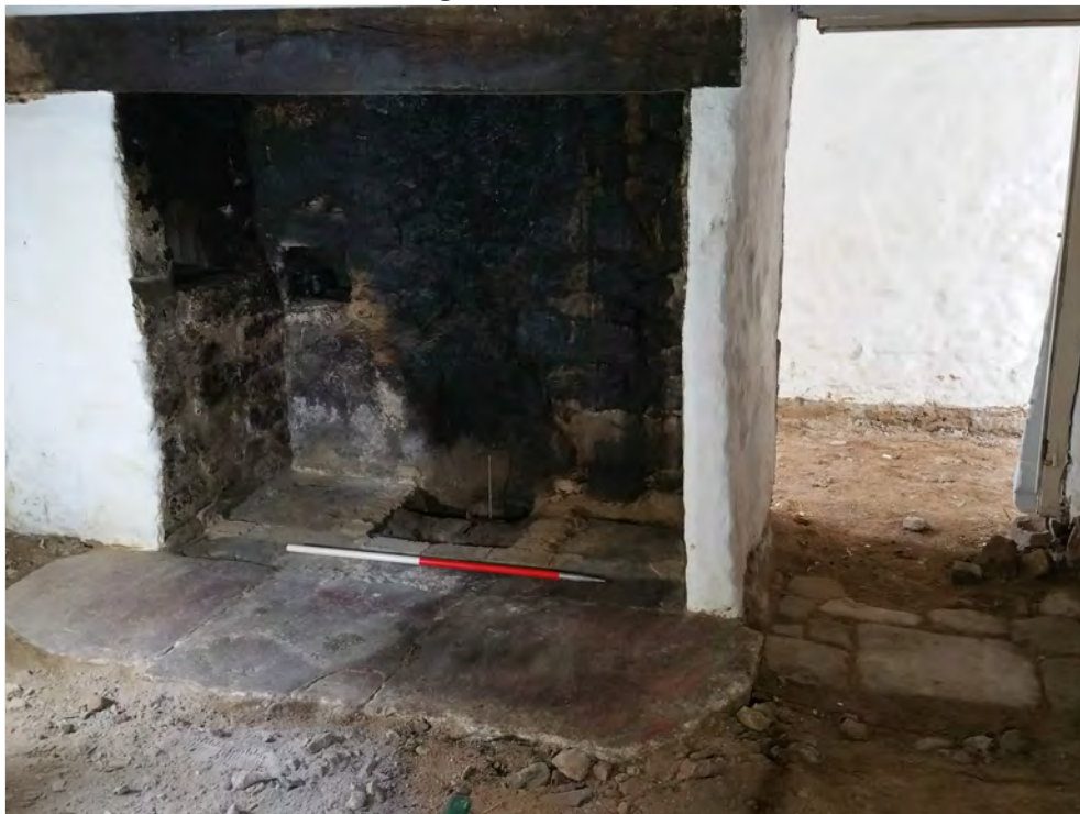
Pl. 2 General view of hall showing granite slabs in front of fireplace and lower surface (right) exposed during the works. 1m scale. Looking south.
