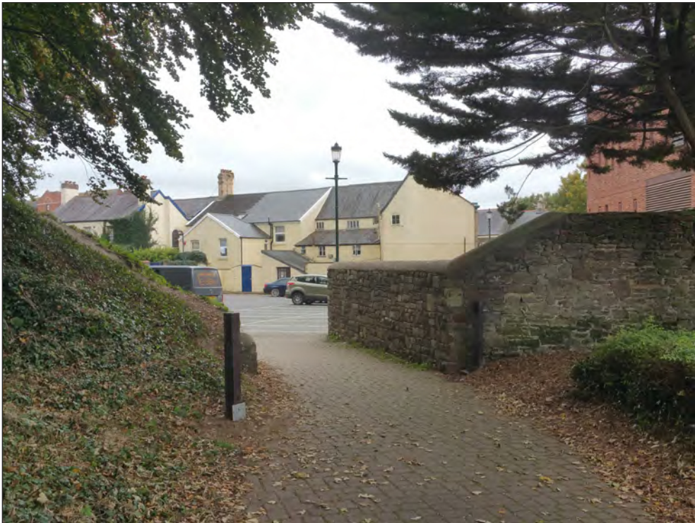
Pl. 9 General view of counter location 4 after installation. Looking southeast.
