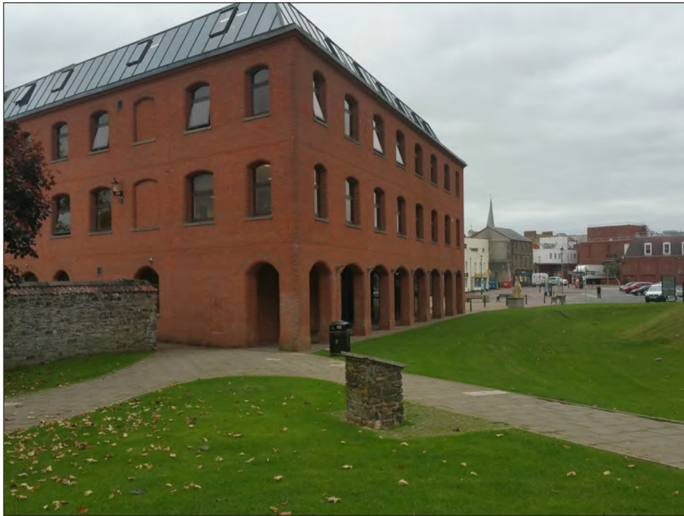
Pl. 12 General view of counter location 5 before installation. Looking southeast.
