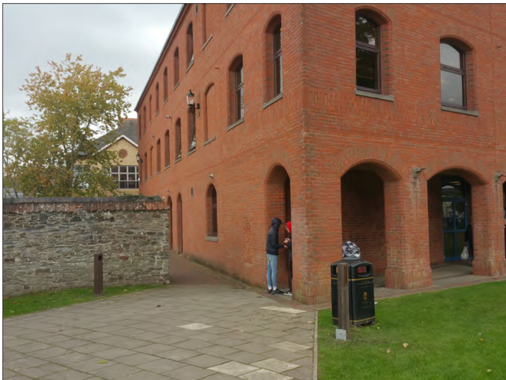
Pl. 13 General view of counter location 5 after installation. Looking southeast.
