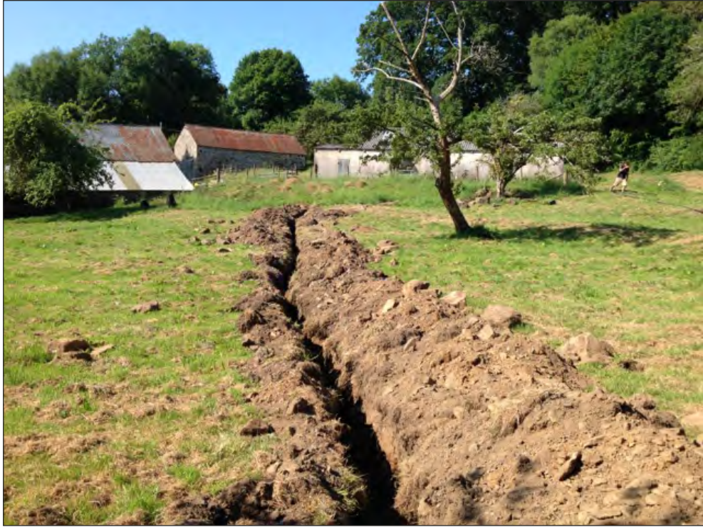
Pl. 3 General view of trench at rear of building. Looking southwest.
