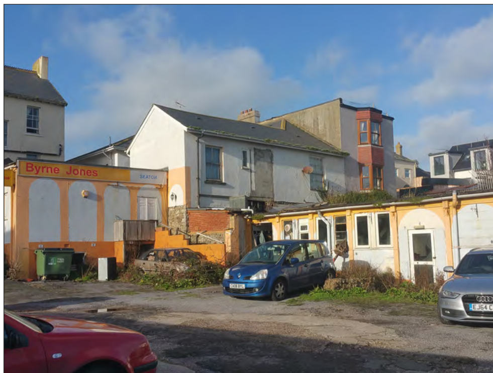
Pl. 4 General view of No. 1 Vintage Court and No. 11 Marine Place showing mid-to-late 19th century outbuilding and post-war extensions. Looking northwest.
