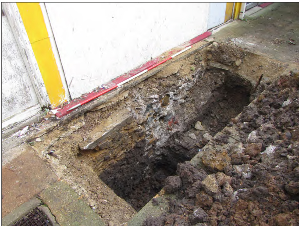
Pl. 6 General view of section through Trench 1 showing wall 108 and underlying deposits (109)-(112). 2m scale. Looking northeast.
