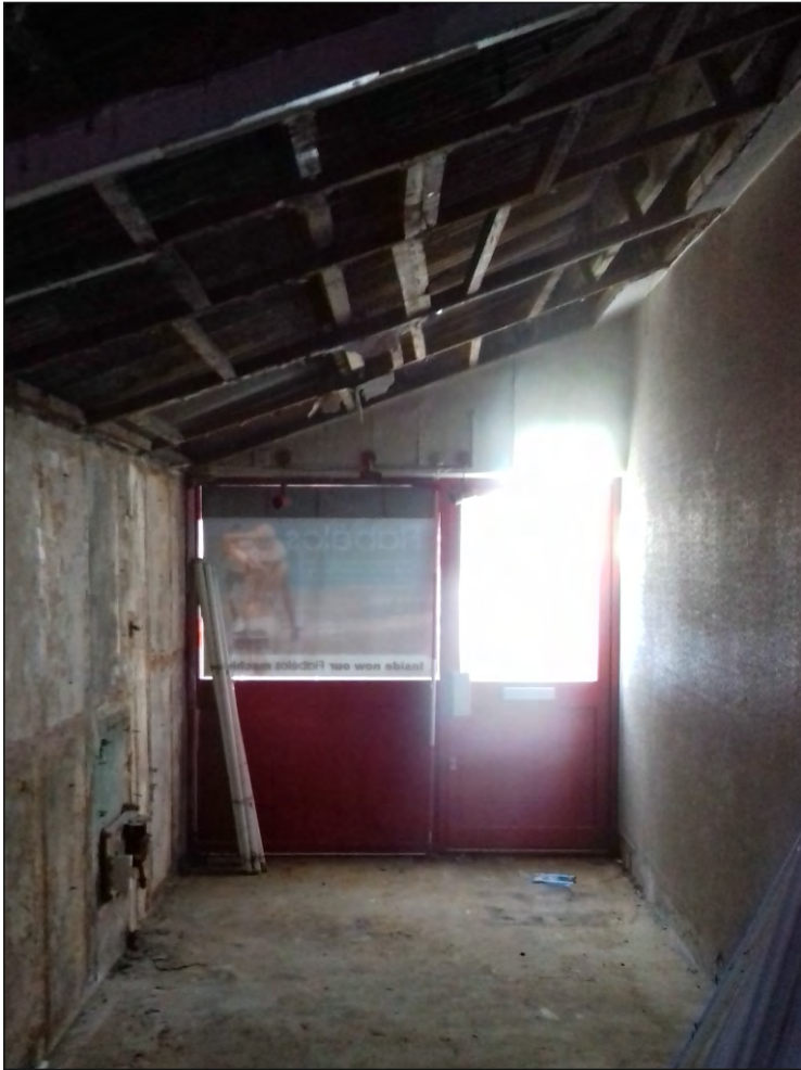
Pl. 6 General view of front elevation of No. 80a Ebrington Street. 2m scale. Looking south.
