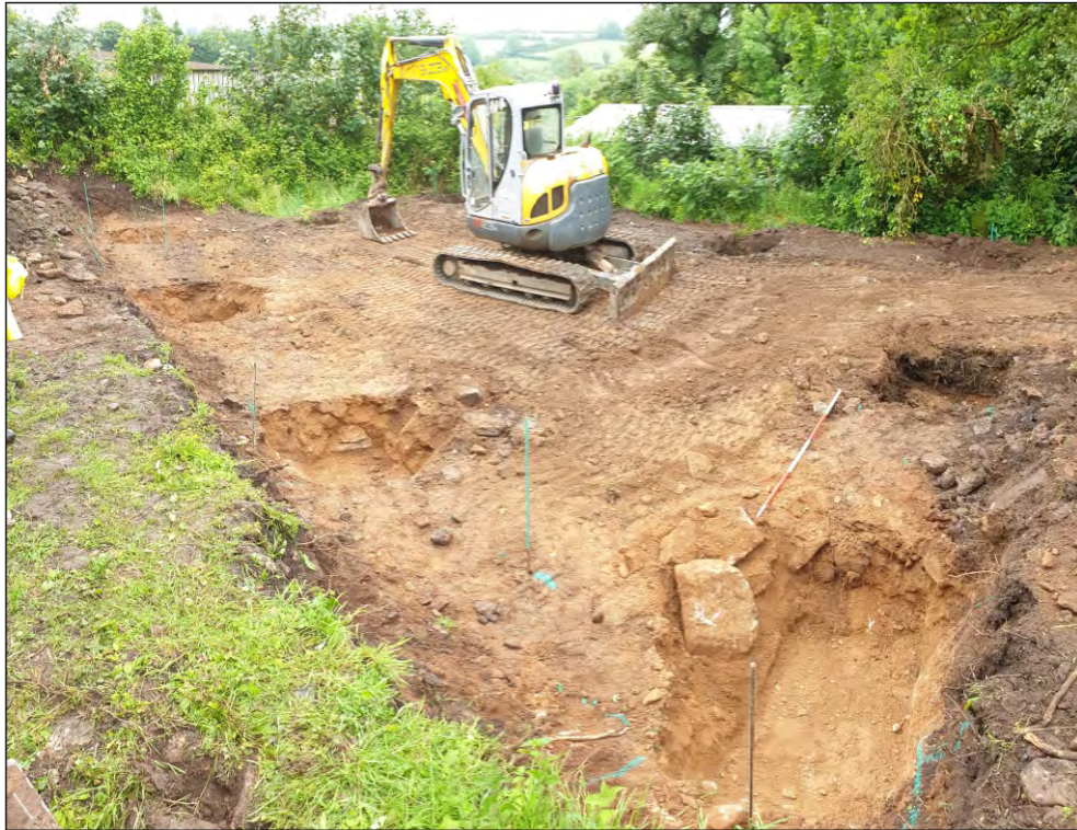
Pl- 1 General view of excavation showing area of cut-and-fill and foundation pads. 2m scale. Looking northeast.
