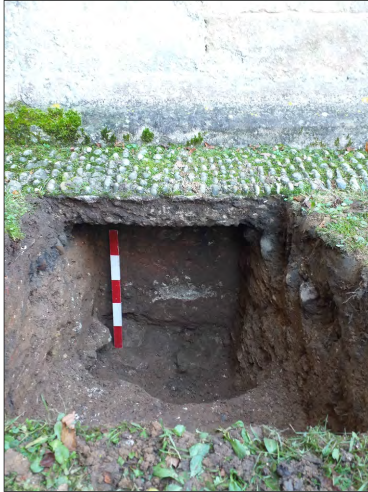
Pl. 3 General view of Trench 3 showing regular masonry (308) above rubble footing (307). 0.5m scale. Looking west.
