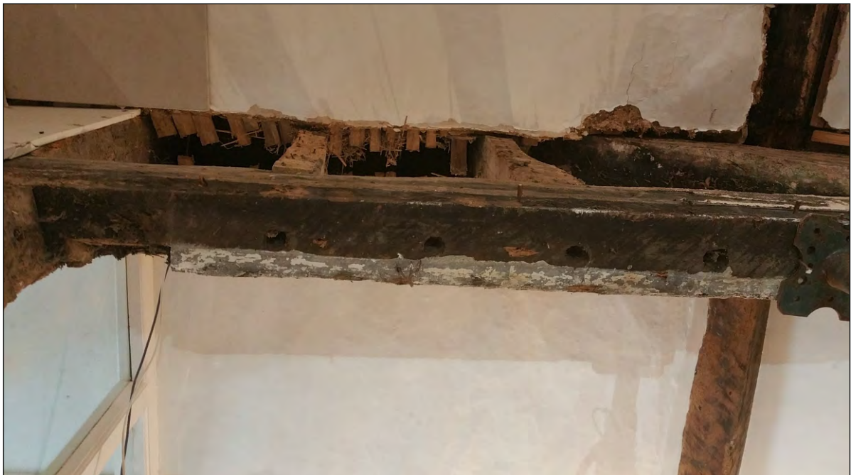
Pl. 20 Close-up of secondary collar showing circular lath holes.
