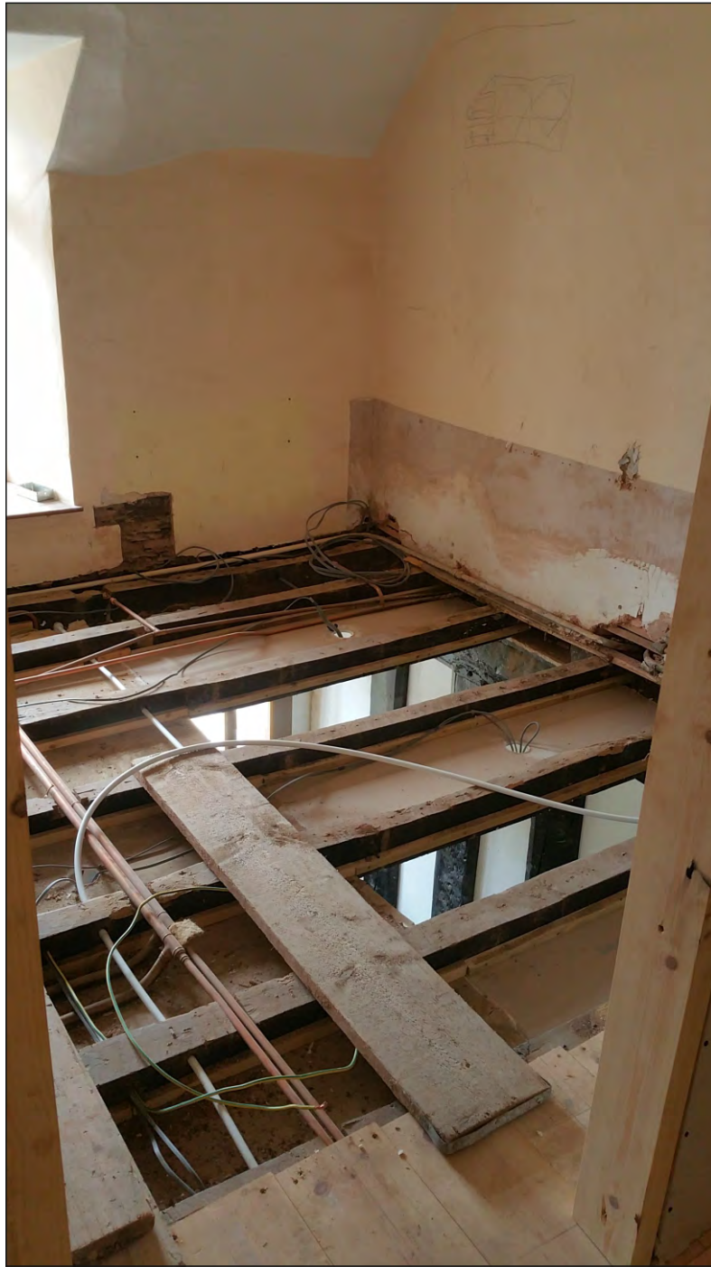
Pl. 21 General view of room F08 showing 19th century floor joists. Looking southeast.
