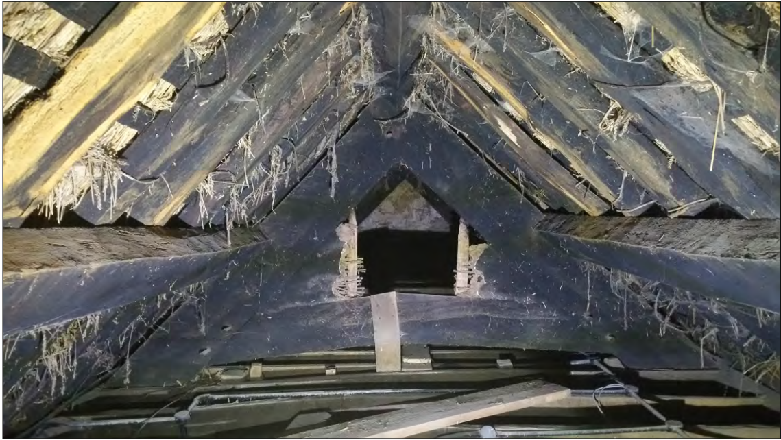
Pl. 24 Close-up of northern jointed cruck truss apex showing cambered collar, trenched purlins, partition and extensive sooting. Looking north.
