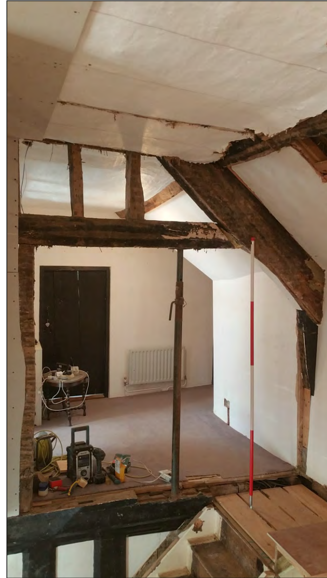
Pl. 18 General view of area at the top of the modern stair showing successive flooring and first-floor partition. 2m scale. Looking southwest.
