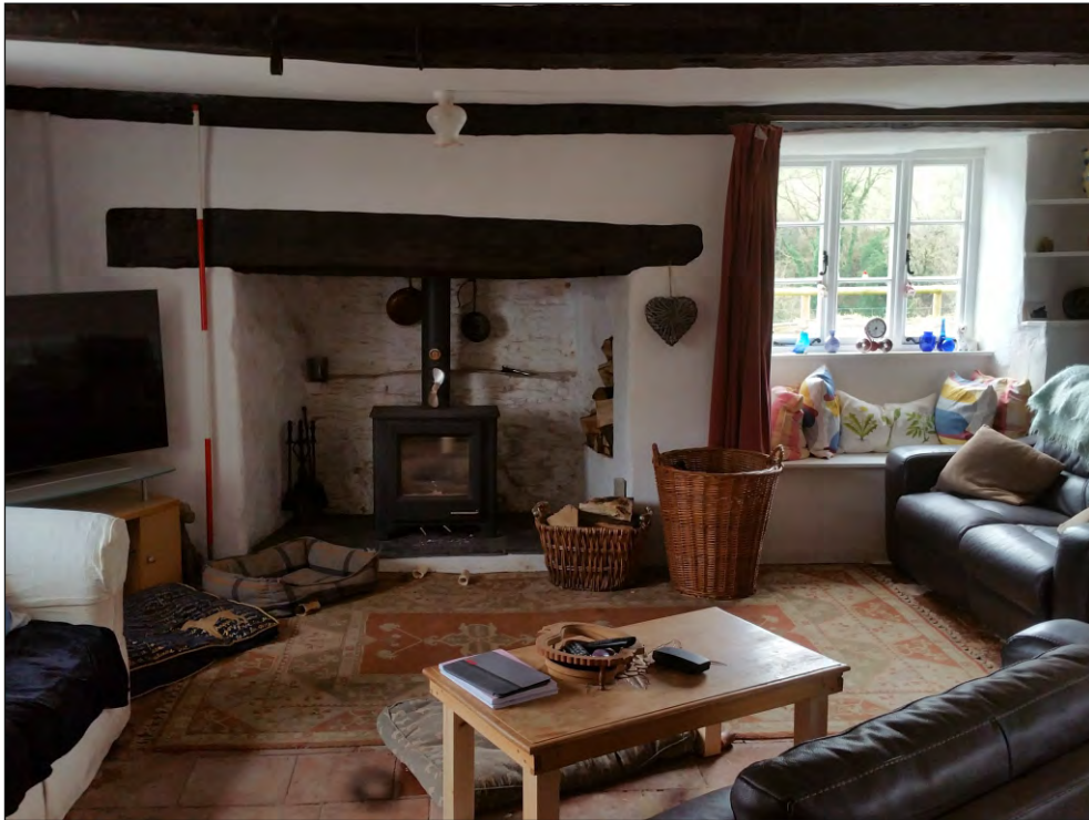
Pl. 8 General view of south elevation of former lower end showing former fireplace and later window. 2m scale. Looking south.
