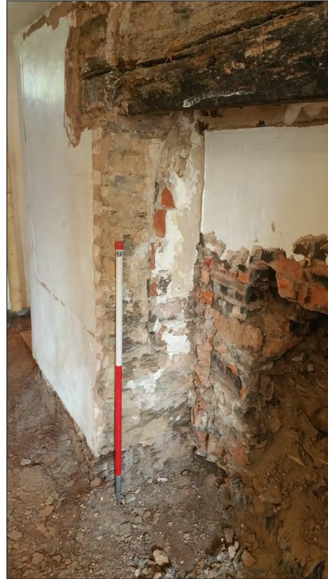
Pl. 16 Close-up of west jamb showing blocked bread-oven. 1m scale. Looking northwest.
