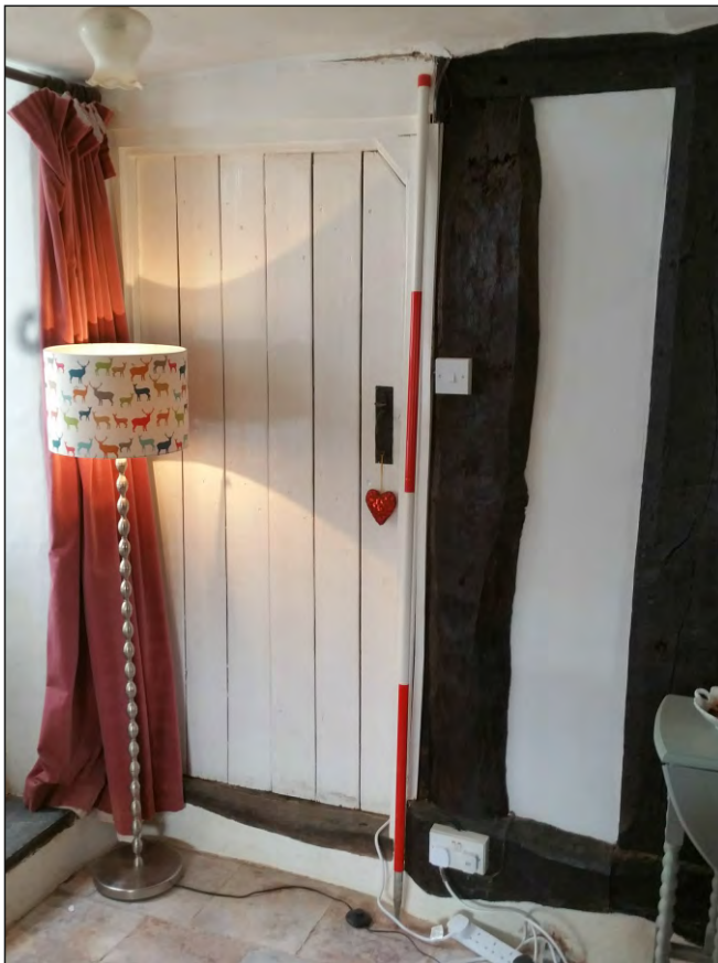
Pl. 6 Close-up showing western end of screen with later doorway and replacement muntin. 2m scale. Looking northwest.
