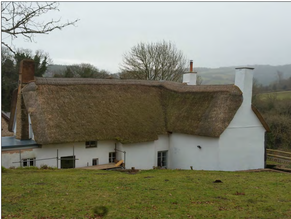
Pl. 2 General view of west elevation of main range with 17th and 20th century extensions. Looking southeast.
