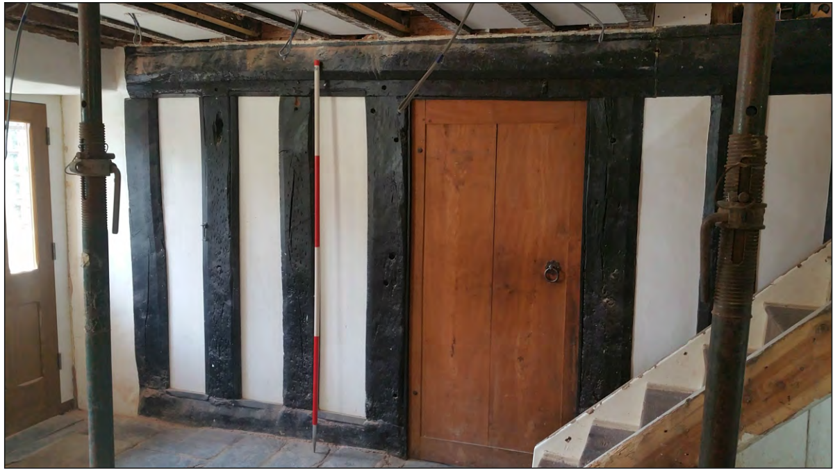
Pl. 3 General view of the plank-and-muntin screen showing original doorway and 20th century staircase. 2m scale. Looking southeast.
