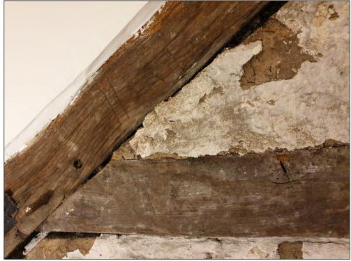
Pl. 16 Close-up of crown strut showing carpenters marks. Looking east.
