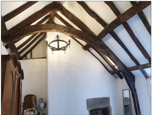
Pl. 10 General view of the jointed cruck truss at the eastern end of Room F05, with through purlins and common rafters. Looking east.
