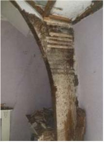
Photo 3: Smoke-blackened rafters & crown strut in truss A
