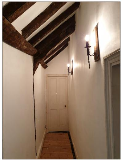
Pl. 8 General view of corridor leading to room F04 showing sooting on the jointed cruck, through purlin and common rafters. Looking east.
