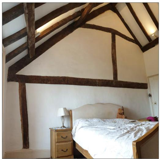
Pl. 13 General view of crown strut forming western partition with simple vertical brace below. Looking northwest.
