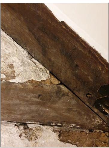
Pl. 17 Close-up of crown strut showing carpenters marks. Looking east.
