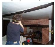
Photo 7: Extraction of a core in progress
