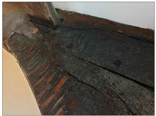
Pl. 12 Close-up of jointed cruck truss showing carpenters marks. Looking east.
