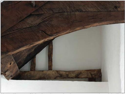
Pl. 11 Close-up of jointed cruck truss showing carpenters marks and detail of later close-studded partition in background. Looking east.
