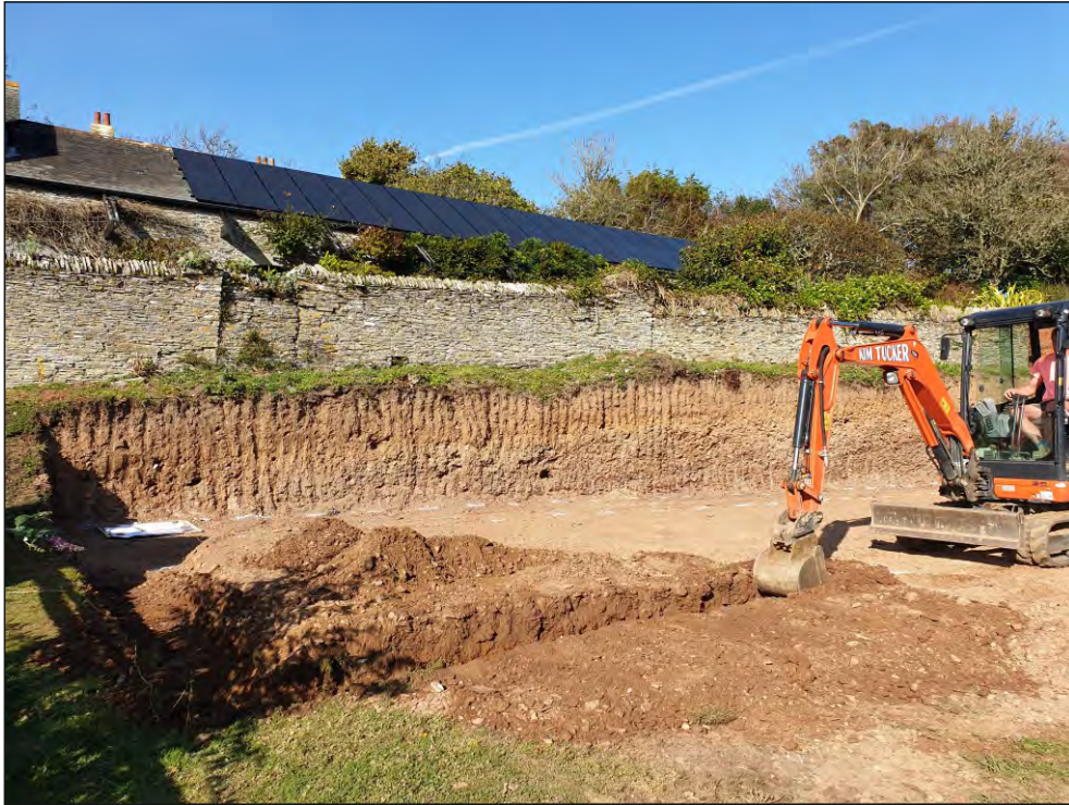
Pl. 1 General view of excavations showing depth of terracing (background) and shallow nature of foundation trenching at western edge. Looking northeast.
