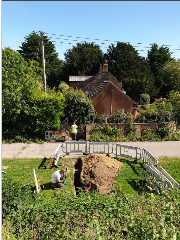
Pl.1 General view of Trenches 1-2. Looking northeast.
