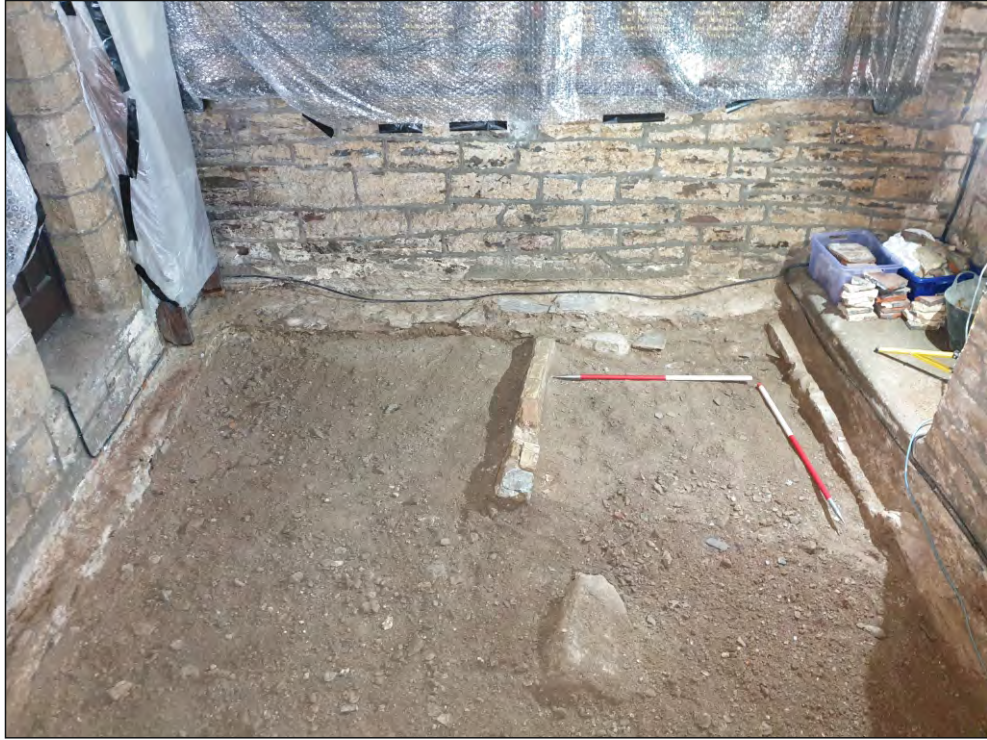
Pl. 1 General view of excavations showing the remains of vault (103/104). 1m scales. Looking southwest.
