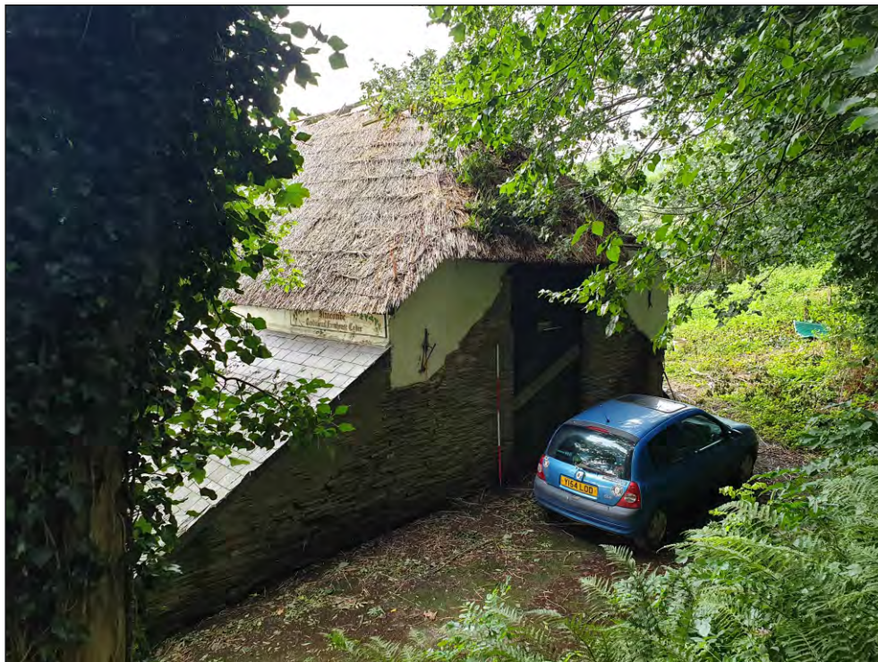
Fig. 6 General view of north elevation showing the original roof height of the lean-to extension and the barn and the subsequent raising of both walls. 2m scale. Looking southwest.
