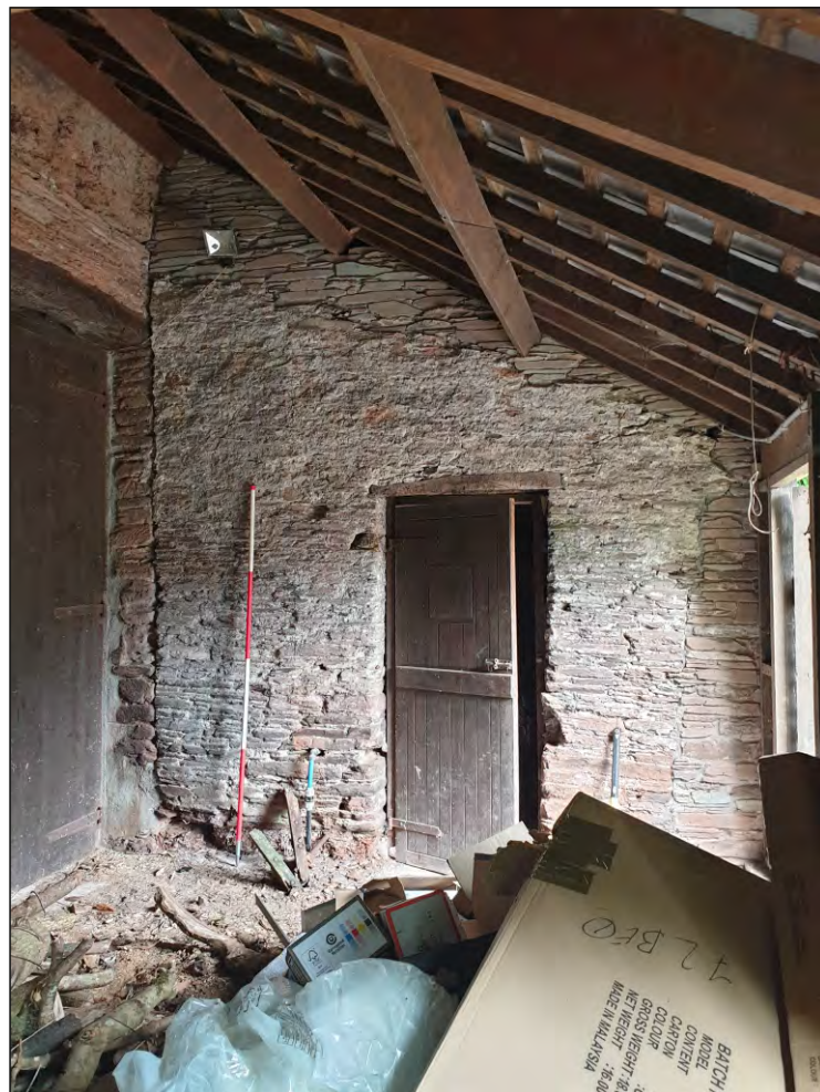
Pl. 2 General view of south elevation of lean-to showing original doorway into the extension with 20th century door. 2m scale. Looking northwest.
