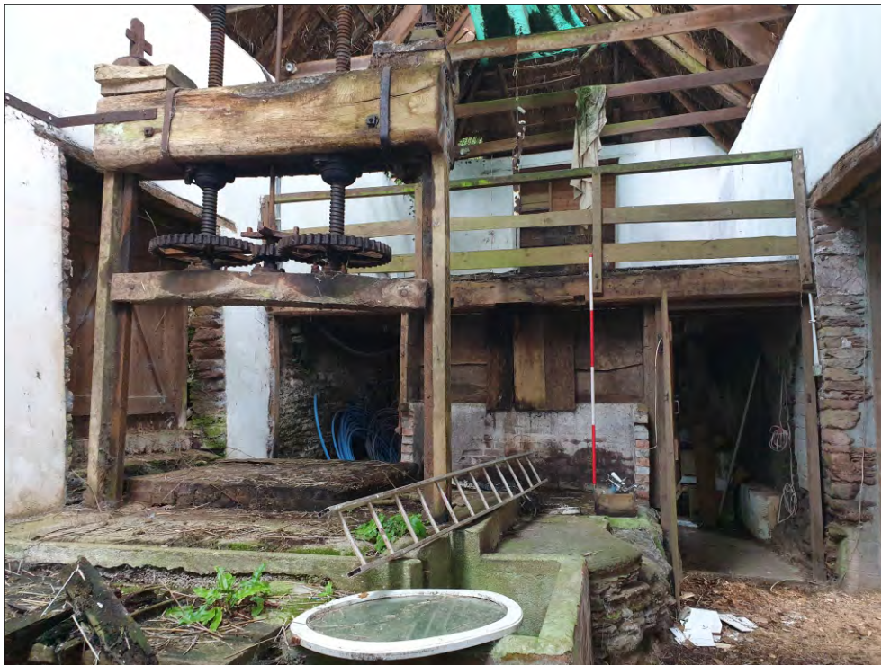
Fig. 11 General view of north end showing modern ground-floor partition with first floor above. 2m scale. Looking northwest.
