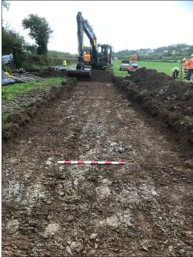
Pl. 1 General view of access road excavations. 1m scale. Looking northwest.
