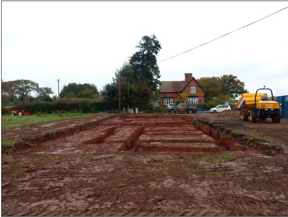
Pl. 1 General view of the two sets of foundations. Looking north.
