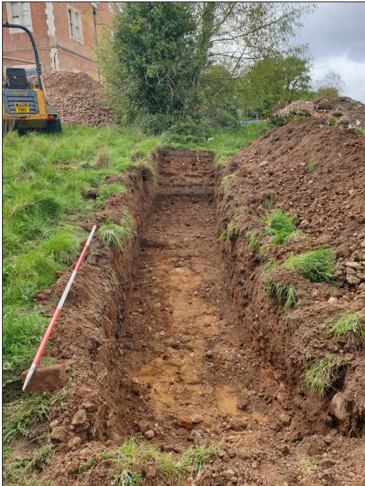
Pl. 20 General view of Trench 5. 2m scale. Looking west.
