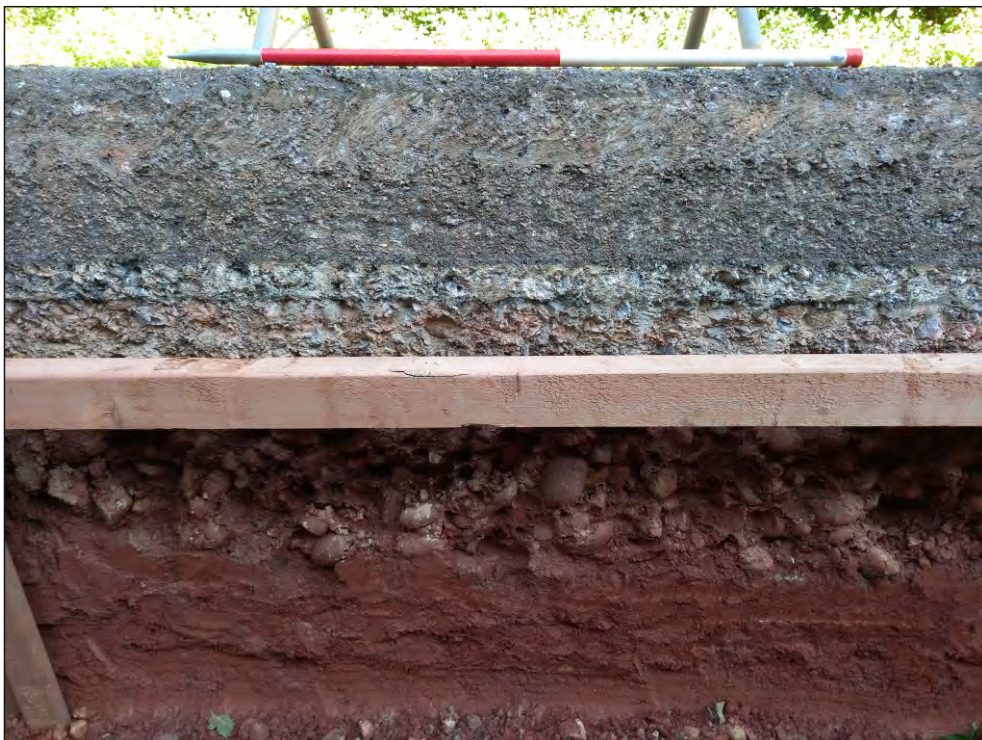
Pl. 14 Close-up showing typical deposit sequence of modern road make-up. 1m scale. Looking northwest.
