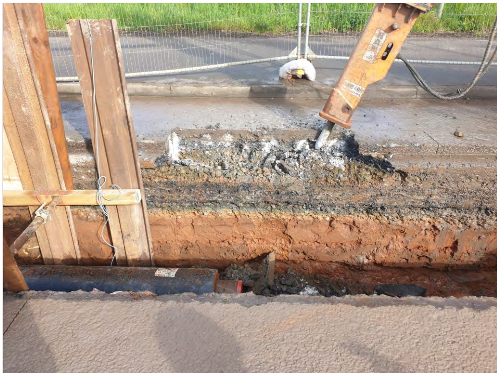
Pl. 4 Close-up showing typical deposit sequence of modern road make-up. 2m scale. Looking northwest.
