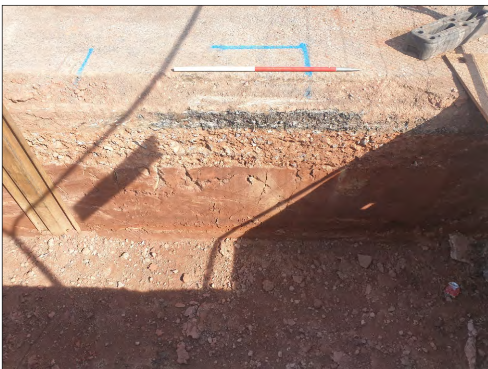
Pl. 6 Close-up showing typical deposit sequence of modern road make-up. 2m scale. Looking northwest.
