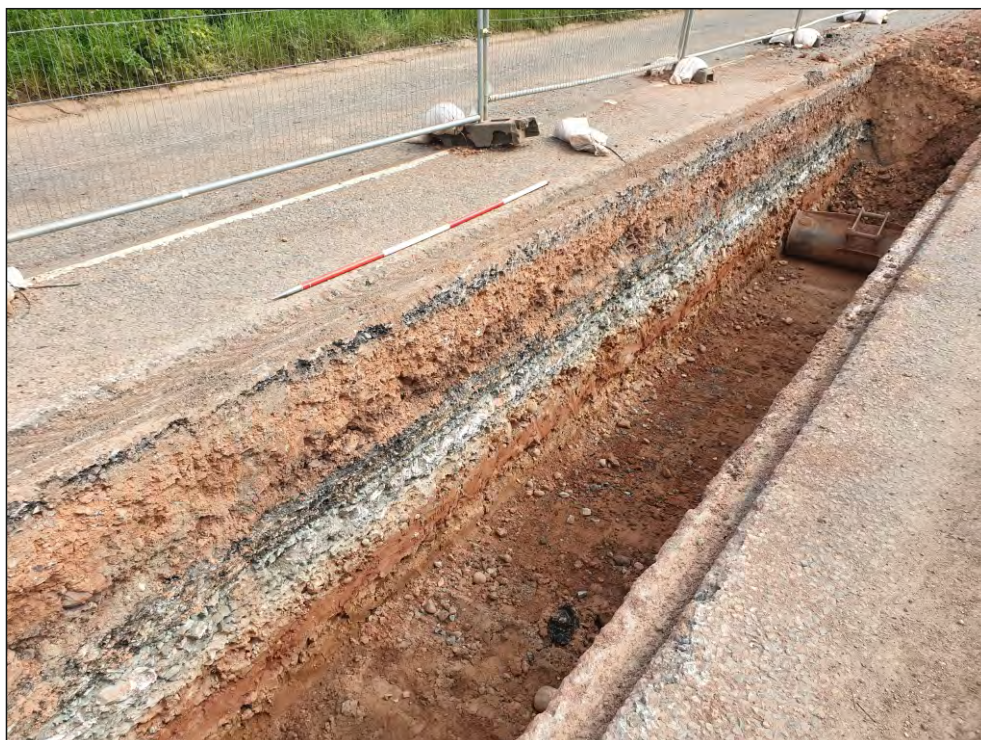
Pl. 8 Close-up showing typical deposit sequence of modern road make-up. 2m scale. Looking northeast.
