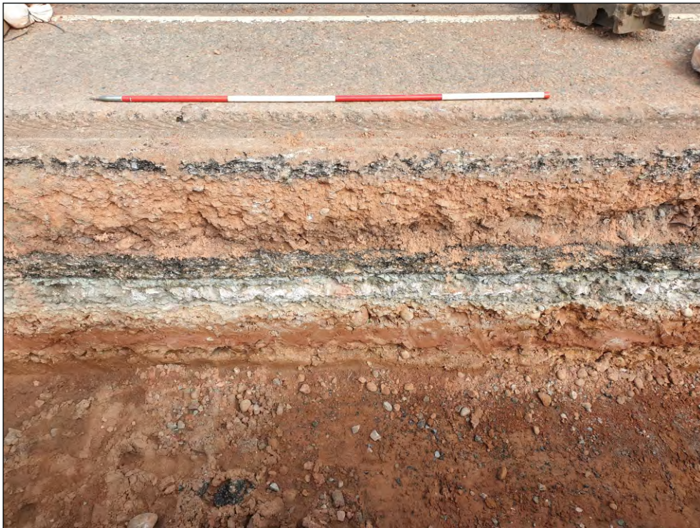
Pl. 9 Close-up showing typical deposit sequence of modern road make-up. 2m scale. Looking northwest.
