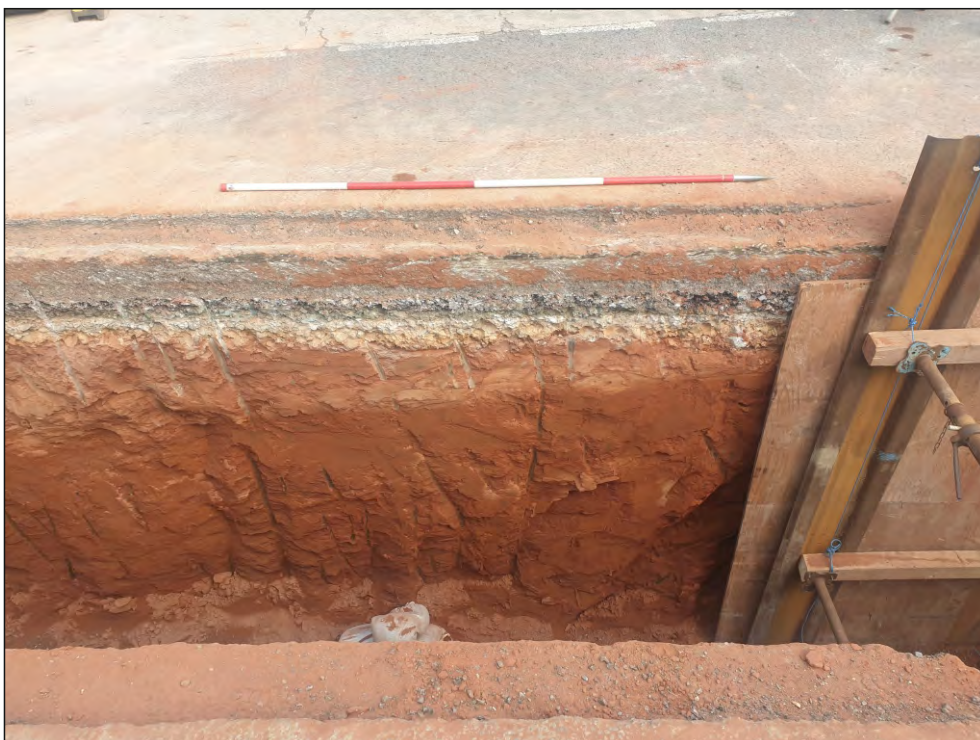
Pl. 2 Close-up showing typical deposit sequence of modern road make-up. 2m scale. Looking northwest.
