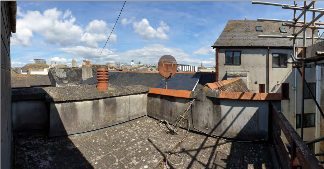
Pl. 37 General view of terrace T03. Looking north.
