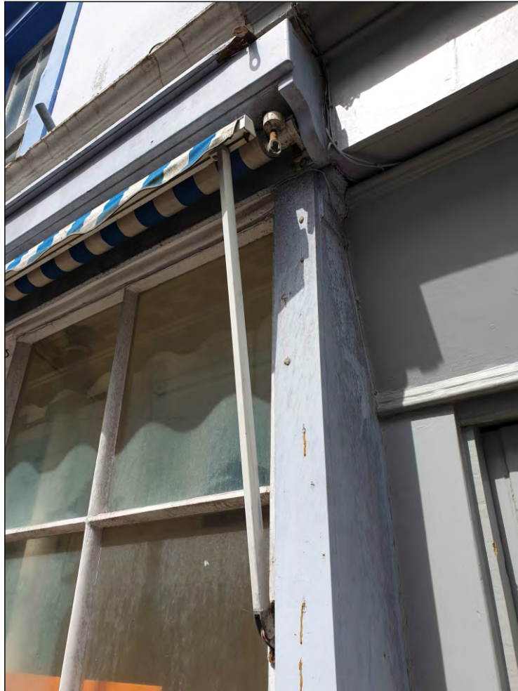
Pl. 3 Close-up of modern awning below original wooden container at No. 25. Looking northwest.
