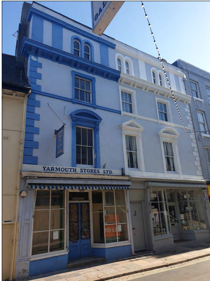
Pl. 1 General view of Nos. 25 and 26 showing mid-19th century stucco façade and originally symmetrical late 19th century ground-floor shop premises. Looking northeast.
