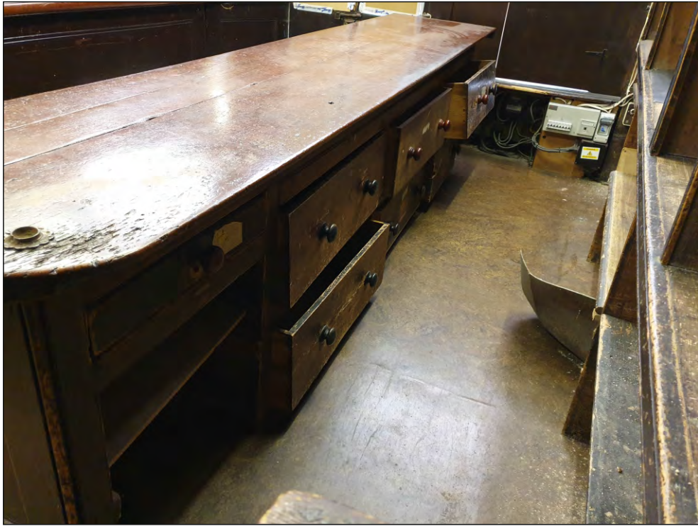
Pl. 7 Close-up of rear of western shop counter showing original drawer configuration and later alterations. Looking southeast.
