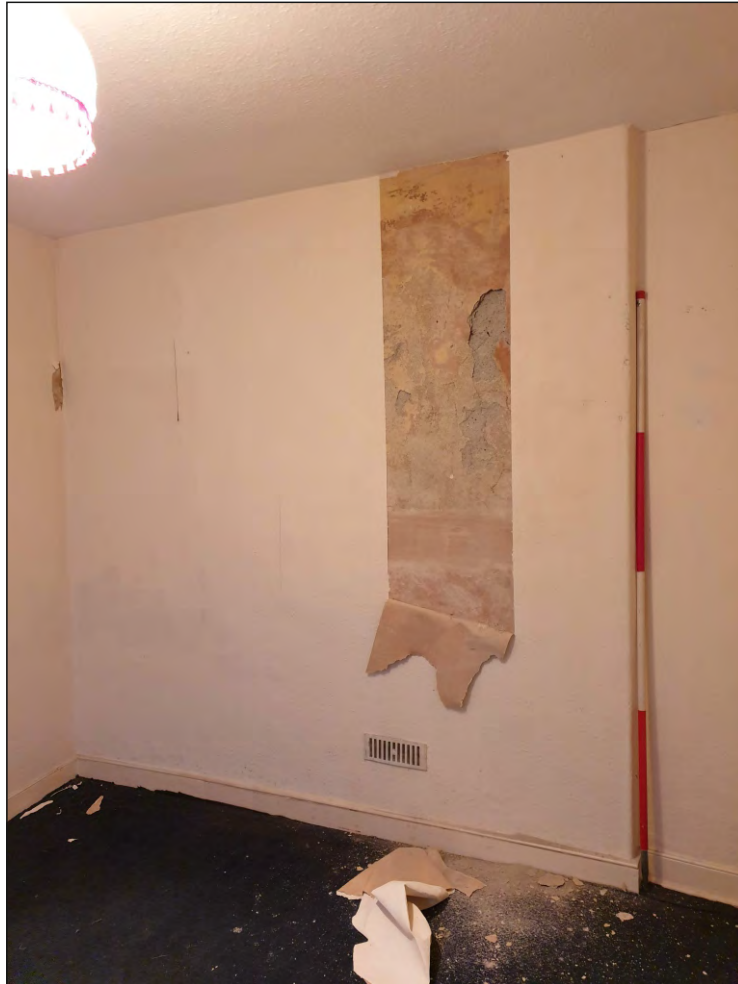
Pl. 31 General view of S04 showing position of former mid-19th century fireplace. 2m scale. Looking southwest.
