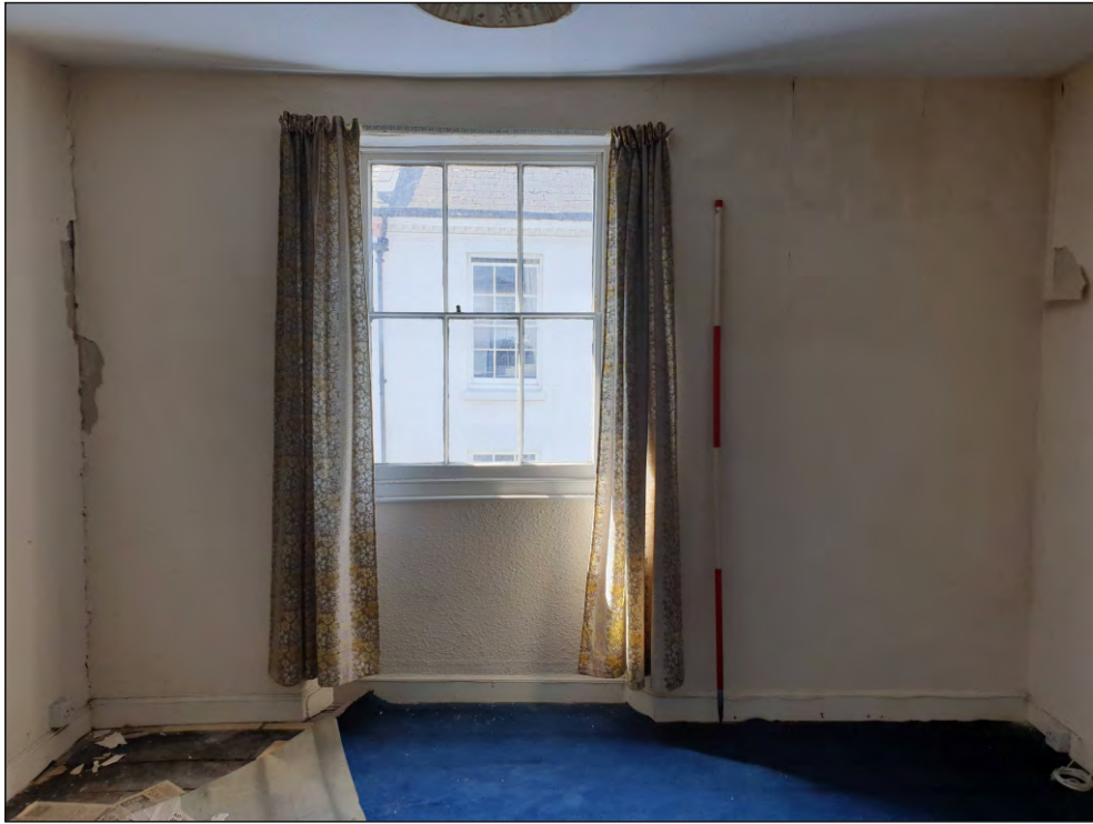
Pl. 27 General view of mid-19th century hornless sash window in S03. 2m scale. Looking south.
