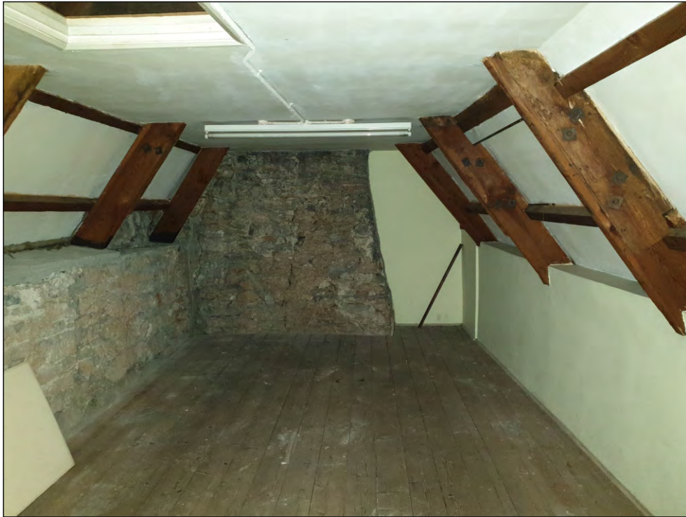
Pl. 47 General view of T04 showing multi-phase chimney in north elevation and feet of heavily repaired 17th century roof trusses. Looking north.
