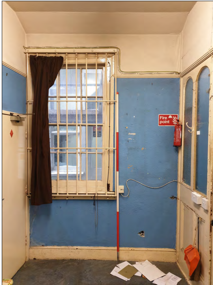
Pl. 11 General view of G02 showing mid-19th century window in east elevation with late 19th century partitions to right and modern door to left. 2m scale. Looking east.
