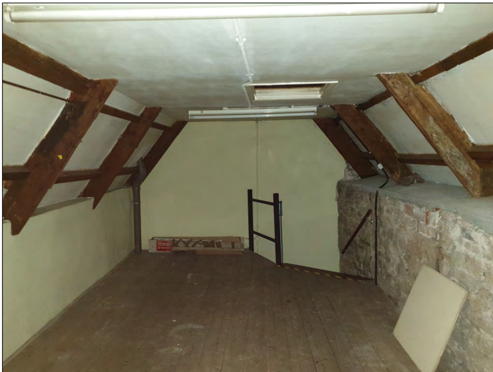
Pl. 48 General view of T04 showing blocking in west elevation of possible dormer window and feet of heavily repaired 17th century roof trusses. Looking north.
