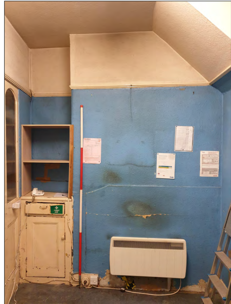
Pl. 12 General view of G02 showing position of former mid-19th century fireplace with low late 19th century cupboard to left. 2m scale. Looking west.
