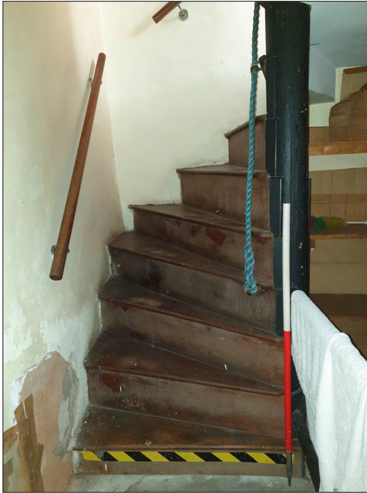
Pl. 43 Close-up of circular stair in G04 showing newel consisting of re-used mast and modern treads-and-risers. 1m scale. Looking west.
