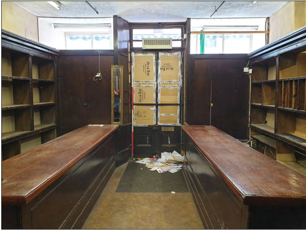
Pl. 5 General view of G01 showing 20th century doorway and modern shop window splays and backs, with late 19th century counters and shelves to left and right. 2m scale. Looking south.
