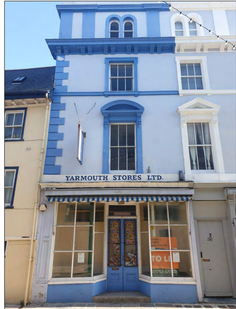
Pl. 2 Close-up of No. 25 showing 20th century replacement shop doorway and door, replacement single glazing bars on both shop window splays and modern awning. Looking north.
