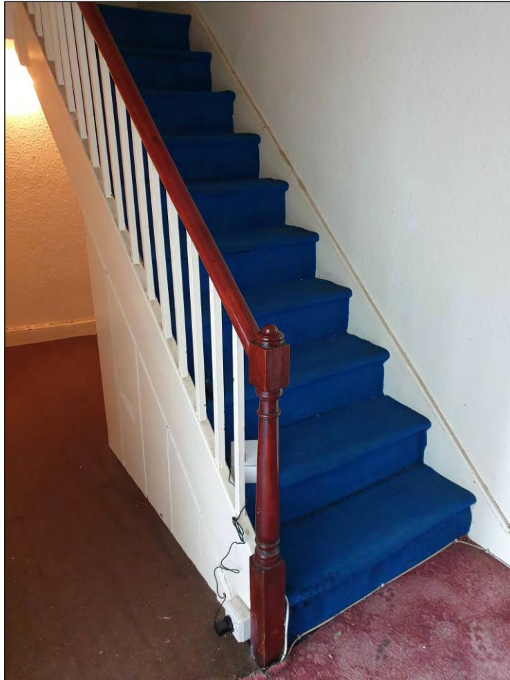
Pl. 25 General view of mid-19th century staircase to second floor. Looking northwest.
