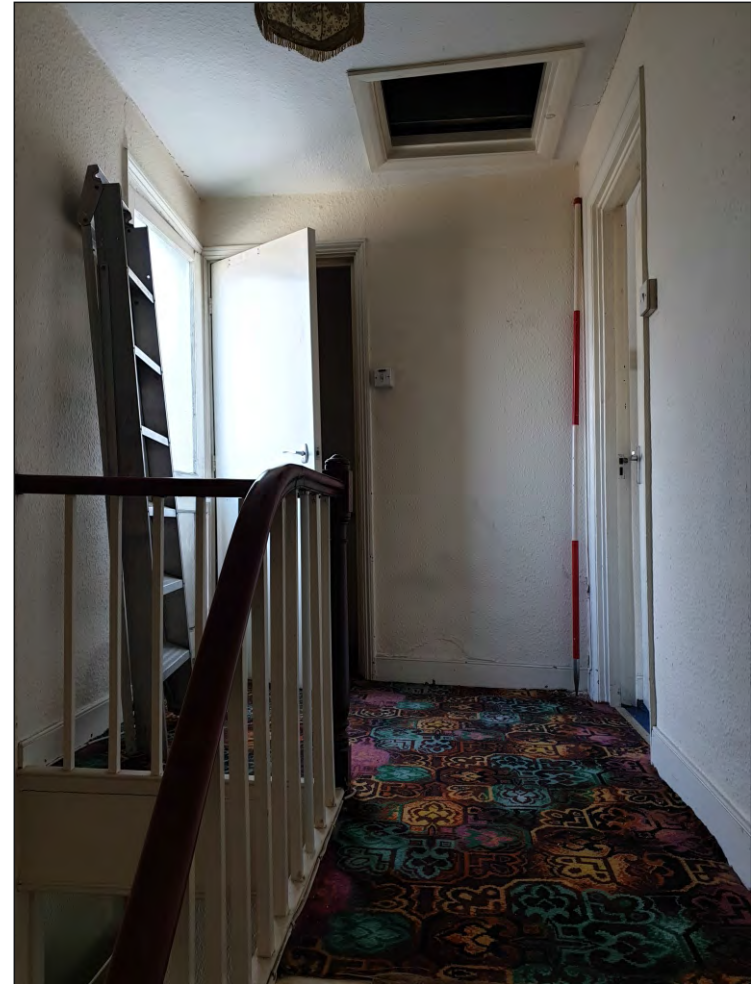
Pl. 32 General view of third floor landing T01 with modern partition in background. 2m scale. Looking east.
