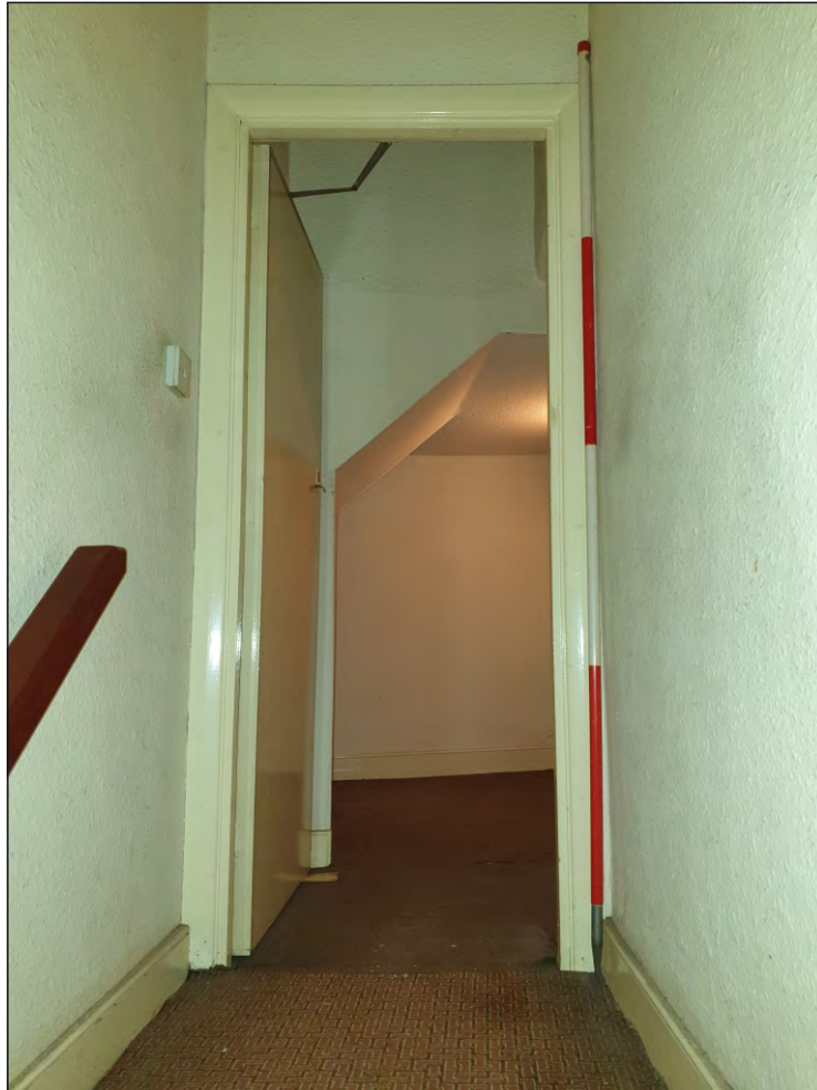
Pl. 17 General view of awkward late 19th century landing F01 above G02 with modern door. 2m scale. Looking south.
