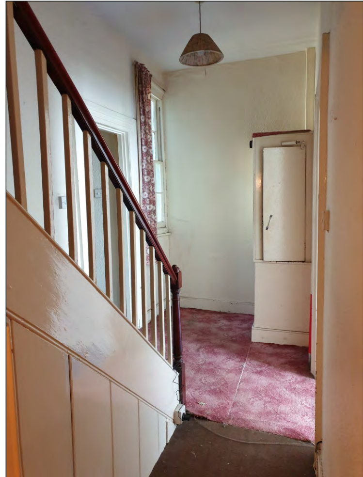
Pl. 18 General view of mid-19th century landing F02 with original mid-19th century sash window in background. 2m scale. Looking east.
