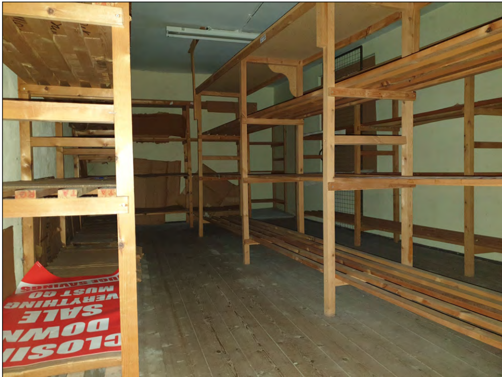
Pl. 46 General view of S05 showing position of former fireplace in north elevation and modern windows in east elevation. 2m scale. Looking north.
