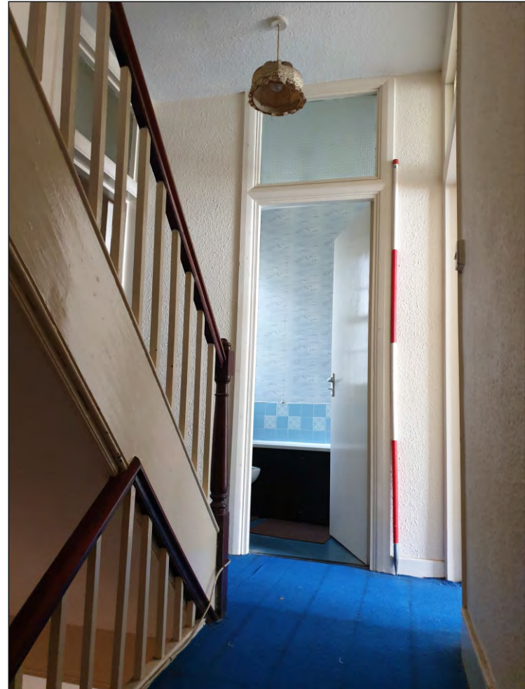
Pl. 26 General view of second floor landing S01 with modern bathroom in background. 2m scale. Looking east.
