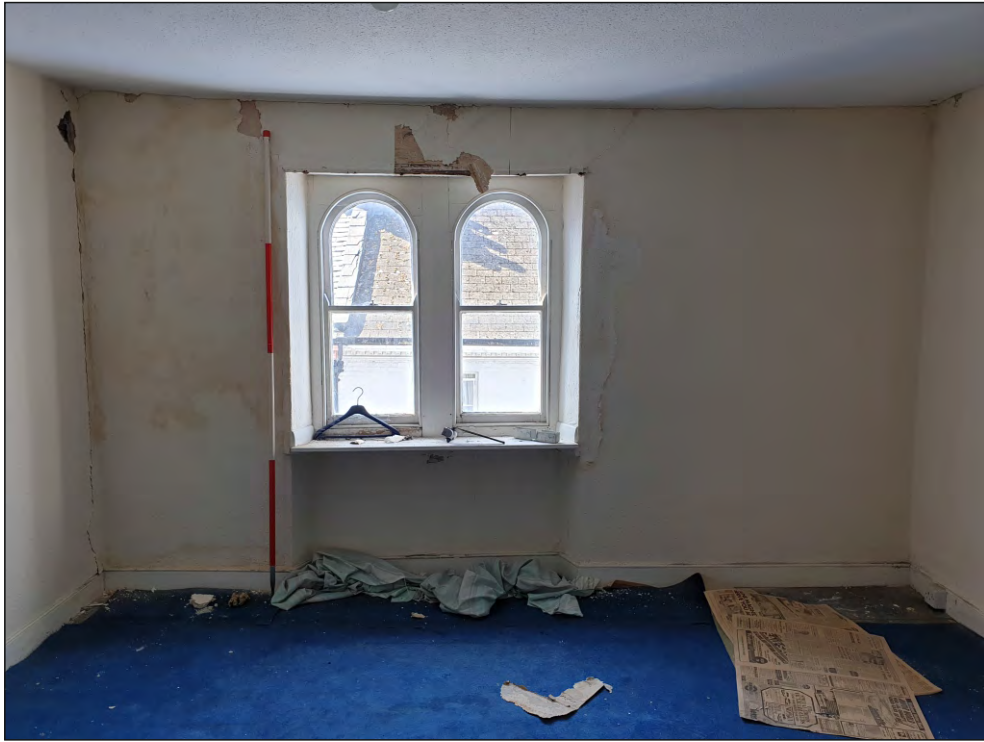
Pl. 35 General view of paired round-arched windows with horned sashes in T02. 2m scale. Looking south.
