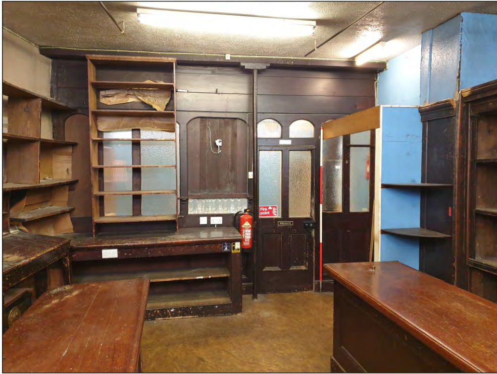
Pl. 9 General view of rear of G01 showing late 19th century partition and modern shelves, with late 19th century shop counter in foreground. 2m scale. Looking north.
