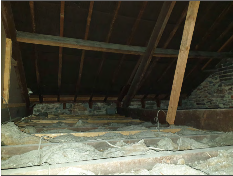
Pl. 40 General view of mid-19th century roof structure. Looking south.
