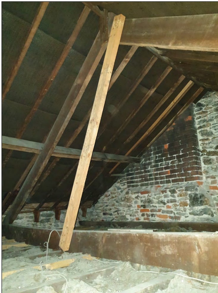
Pl. 38 General view of mid-19th century roof structure. Looking southwest.
