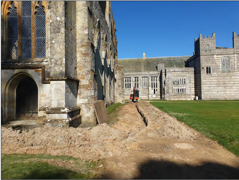
Pl. 5 General view of electric trench across east end of abbey church. Looking north.
