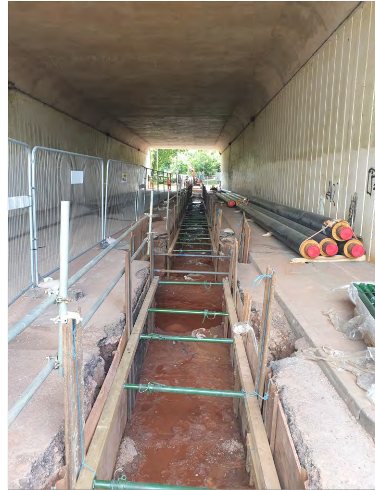
Pl. 2 General view of trenching route within M5 Motorway tunnel. Looking northwest.
