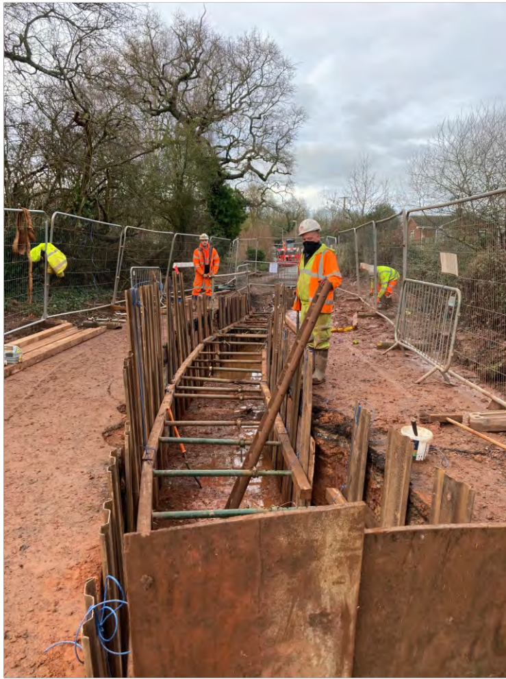
Pl. 3 General view of trenching route leading to Pin Brook. Looking northwest.
