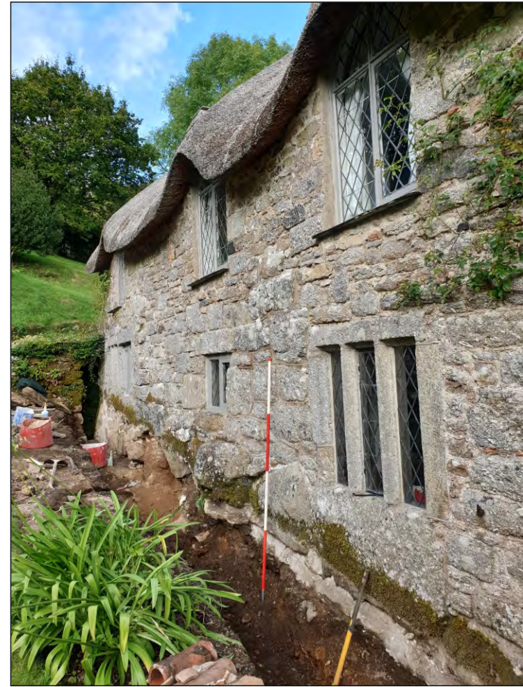
Pl. 2 General view of west elevation showing base of wall above gowan and granite bedrock protrusions. 2m scale. Looking northeast.
